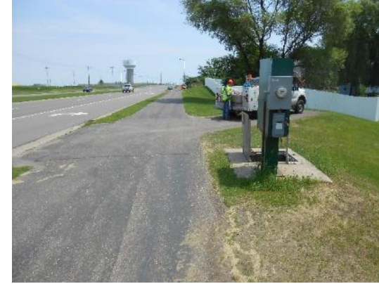
Meter Telemetry Cabinet & Instrumentation Panel
