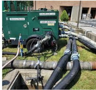
Source: Trenchless Technologies, website
