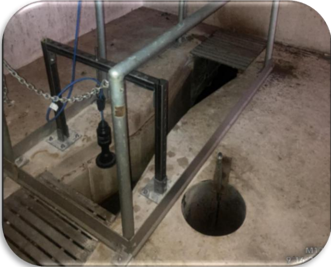
Parshall Flume with suspended level “radar” sensor. Note stilling well.
