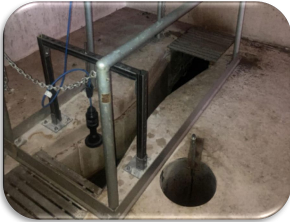
Parshall Flume with suspended level “radar” sensor. Note stilling well.
