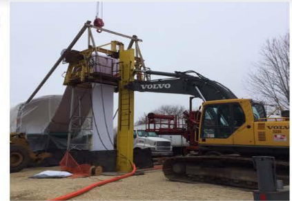
Large equipment is needed to insert liners into manholes and sewers.
