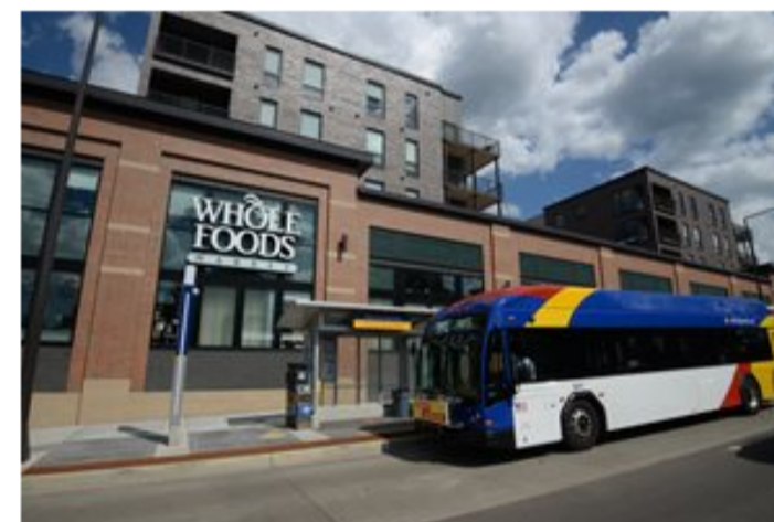
St. Paul, Snelling Avenue. A new station for the A Line Rapid Bus resulted from coordination between the City of St. Paul, Metro Transit, and the developer of the Vintage on Selby, the Excelsior Group.
