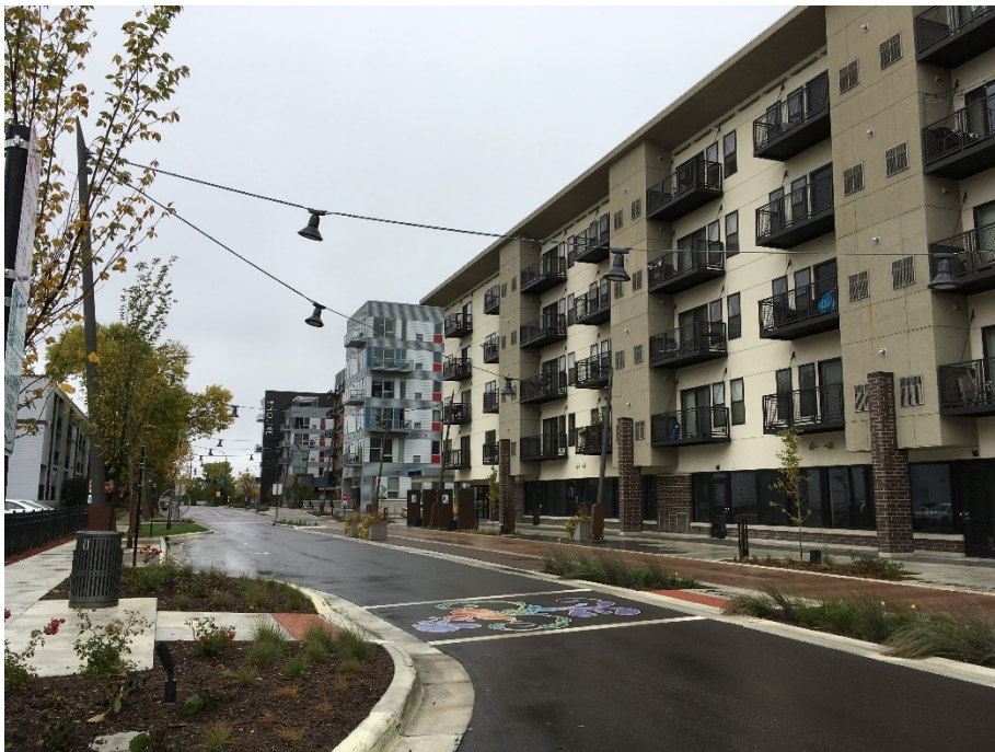
Looking south along the Artery with the recent development of Gallery Flats (foreground) and the Moline (background)
