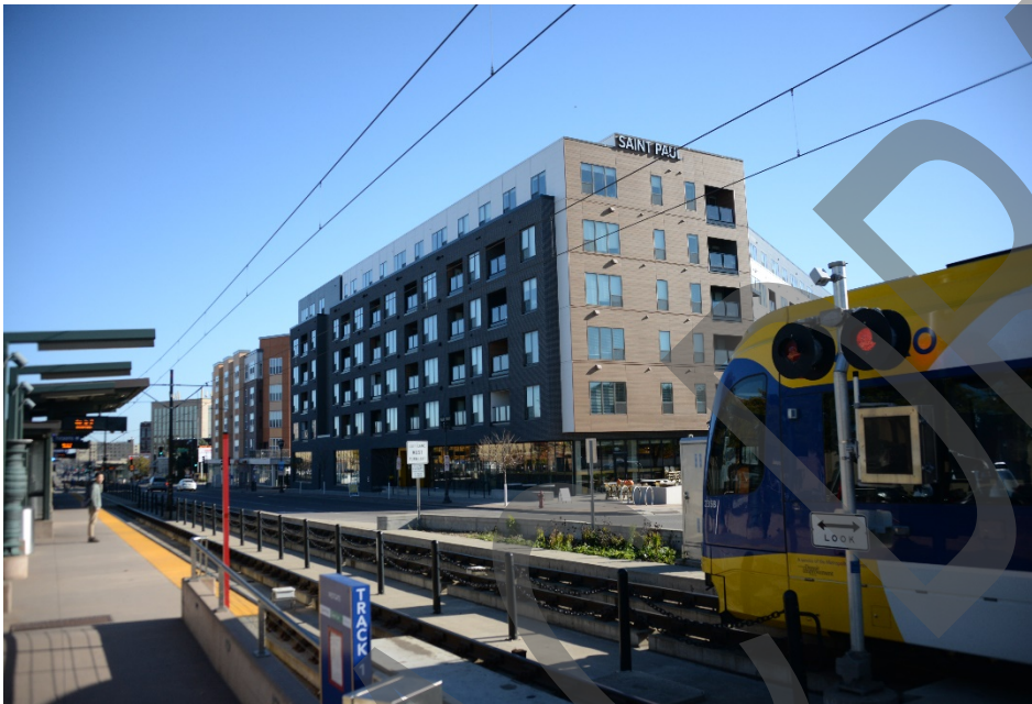
Saint Paul, University Avenue. Looking southeast toward 2700 University across the street from the METRO Green Line Westgate Station.
