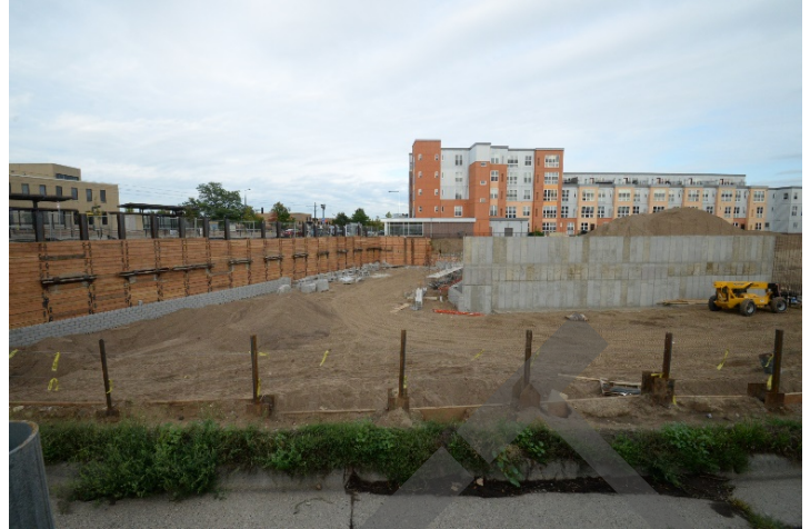
Construction underway on 2700 University Avenue
