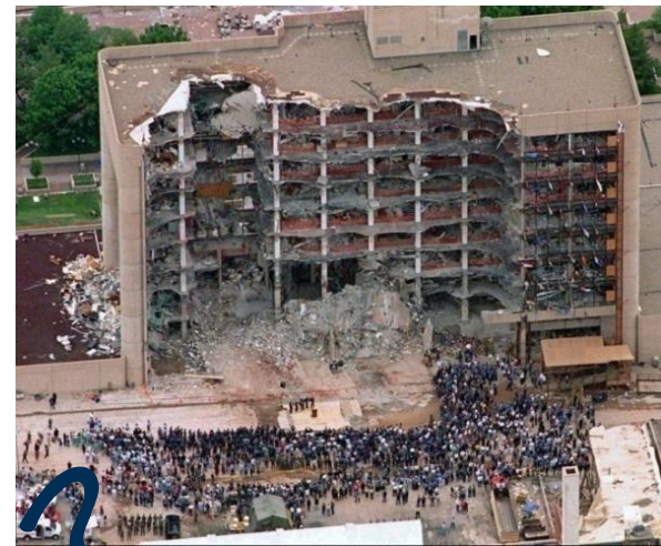
A. P. Murrah Building Oklahoma City, OK
