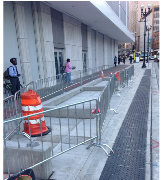
Figure 2: Constructed Station Improvements
