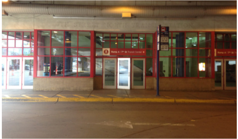
Figure 1: Existing Ramp A/7th Street Transit Center
