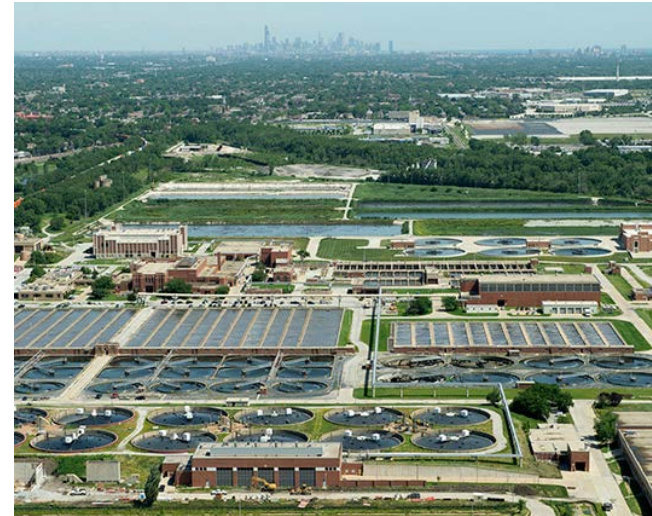
Calumet Water Reclamation Plant
