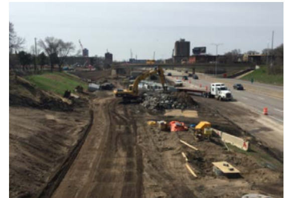
11th St Ramp Reconstruction
