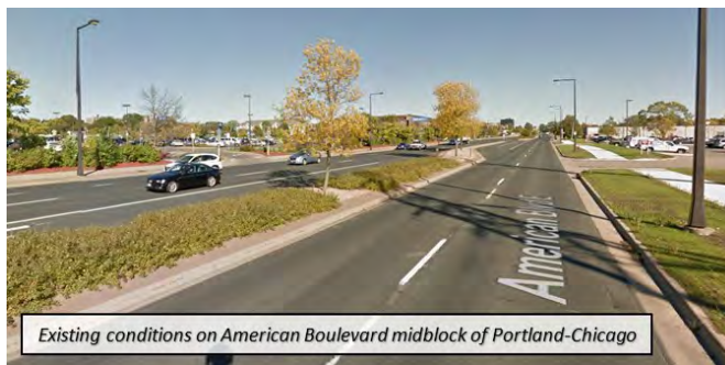
Figure 63: Midblock locations on American Boulevard
