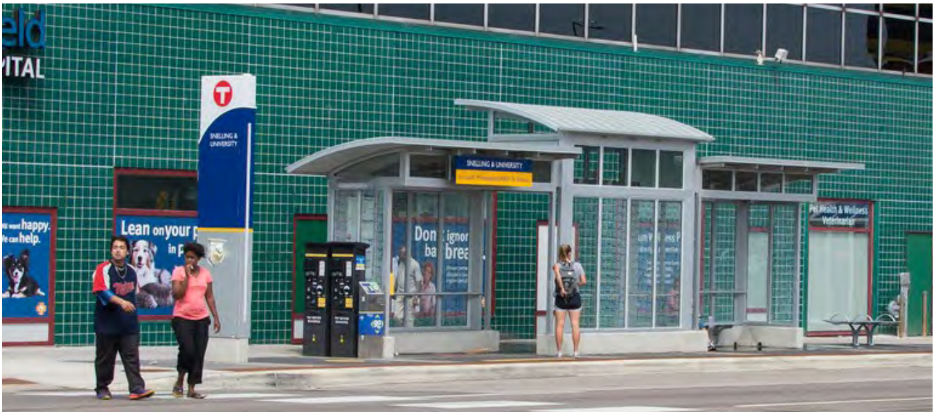
Figure 13: Large shelter on the A Line, Snelling & University station
