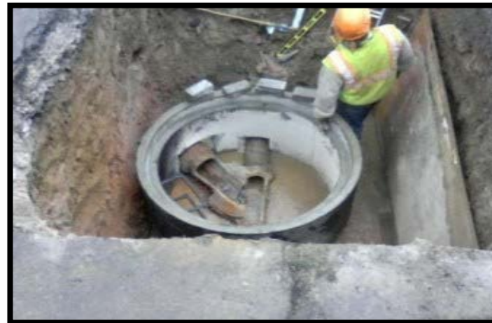
Replace Manhole Structures
