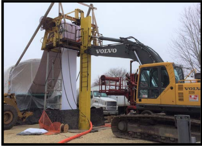
Riverview Lane (CIPP Lining)
