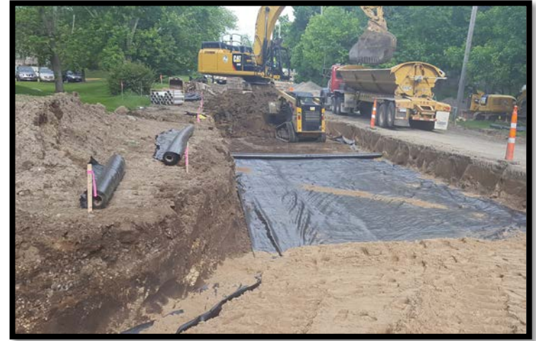
Mississippi Lane (Pipe Replacement)
