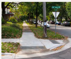
ADA-Compliant Curb Ramps
