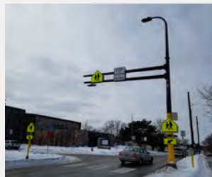
Traffic control device and APS push buttons
