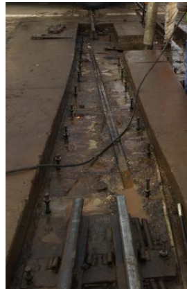
Crossover Casting Replacement
