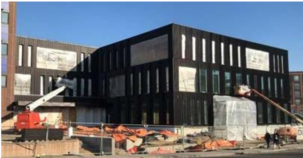
(New MTPD facility under construction)
