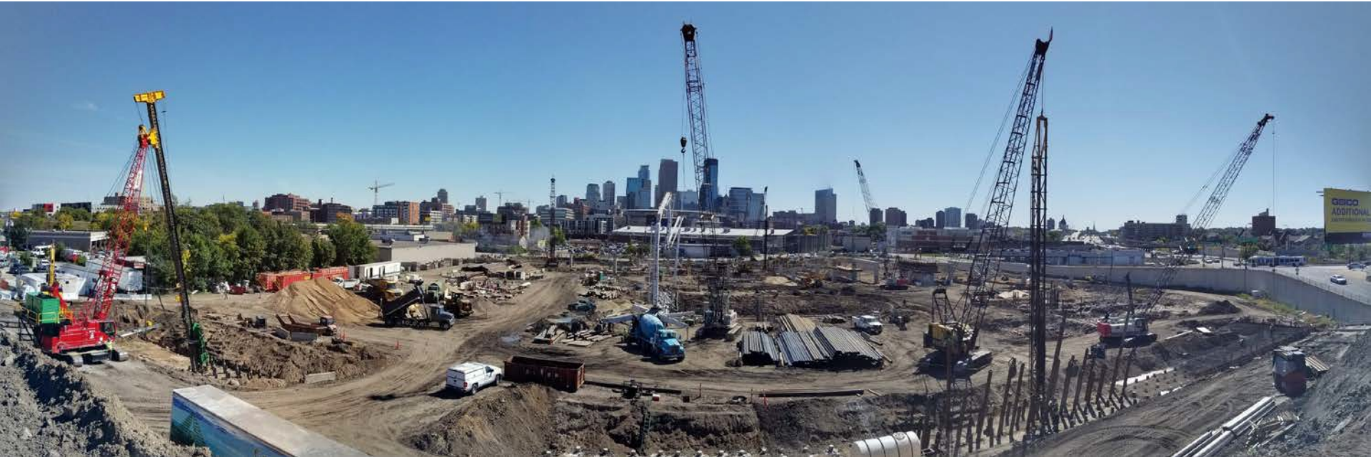
Pile driving, excavation for rainwater storage tank, retaining wall foundation
