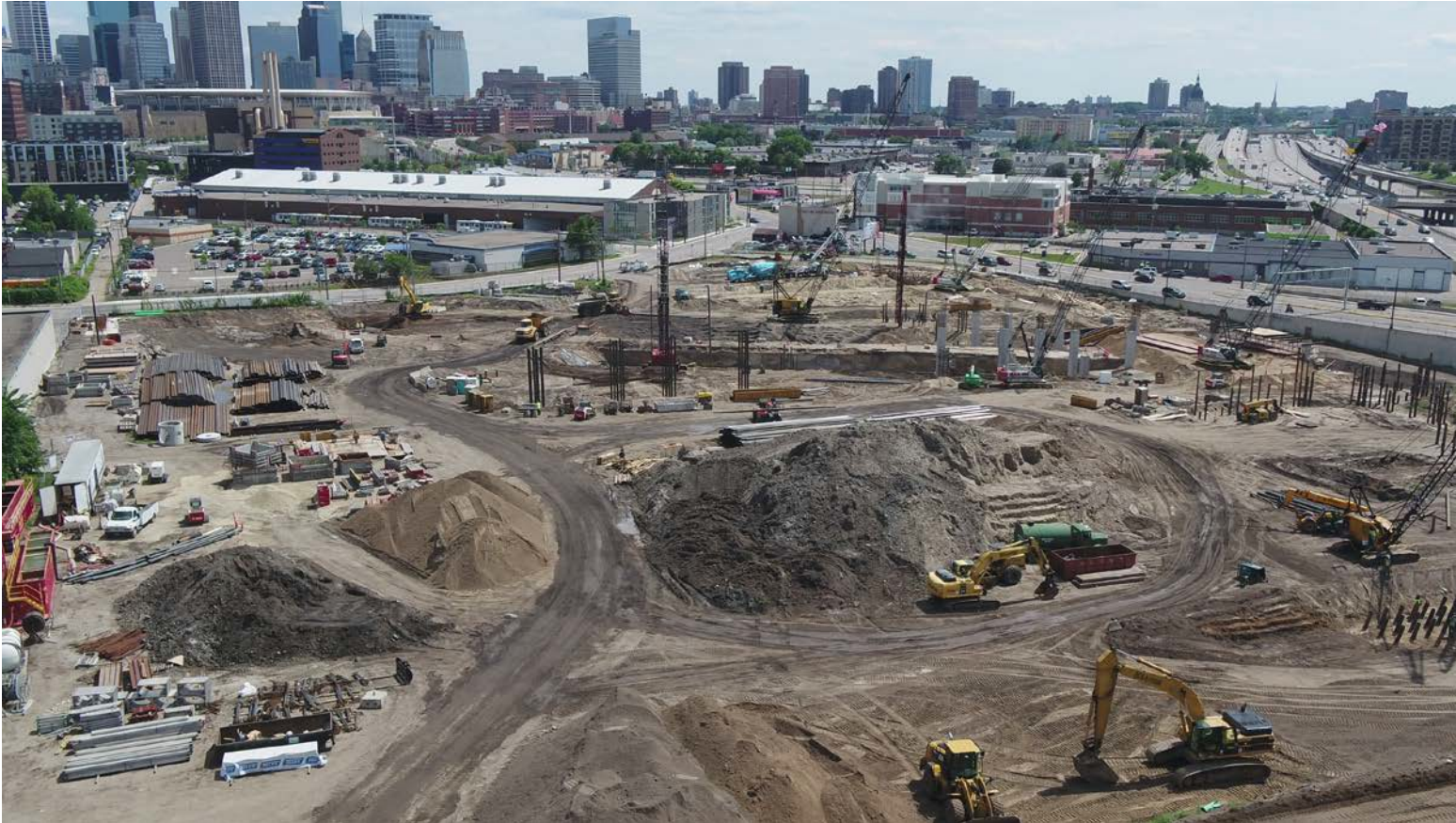
Earthmoving, pile driving, construction over Bassett Creek stormwater tunnel
