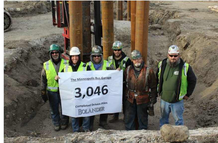
Pile driving construction crew
