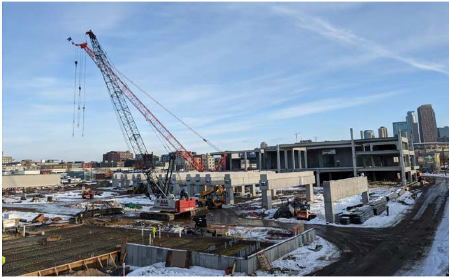
Precast wall panel and column erection for the operations building
