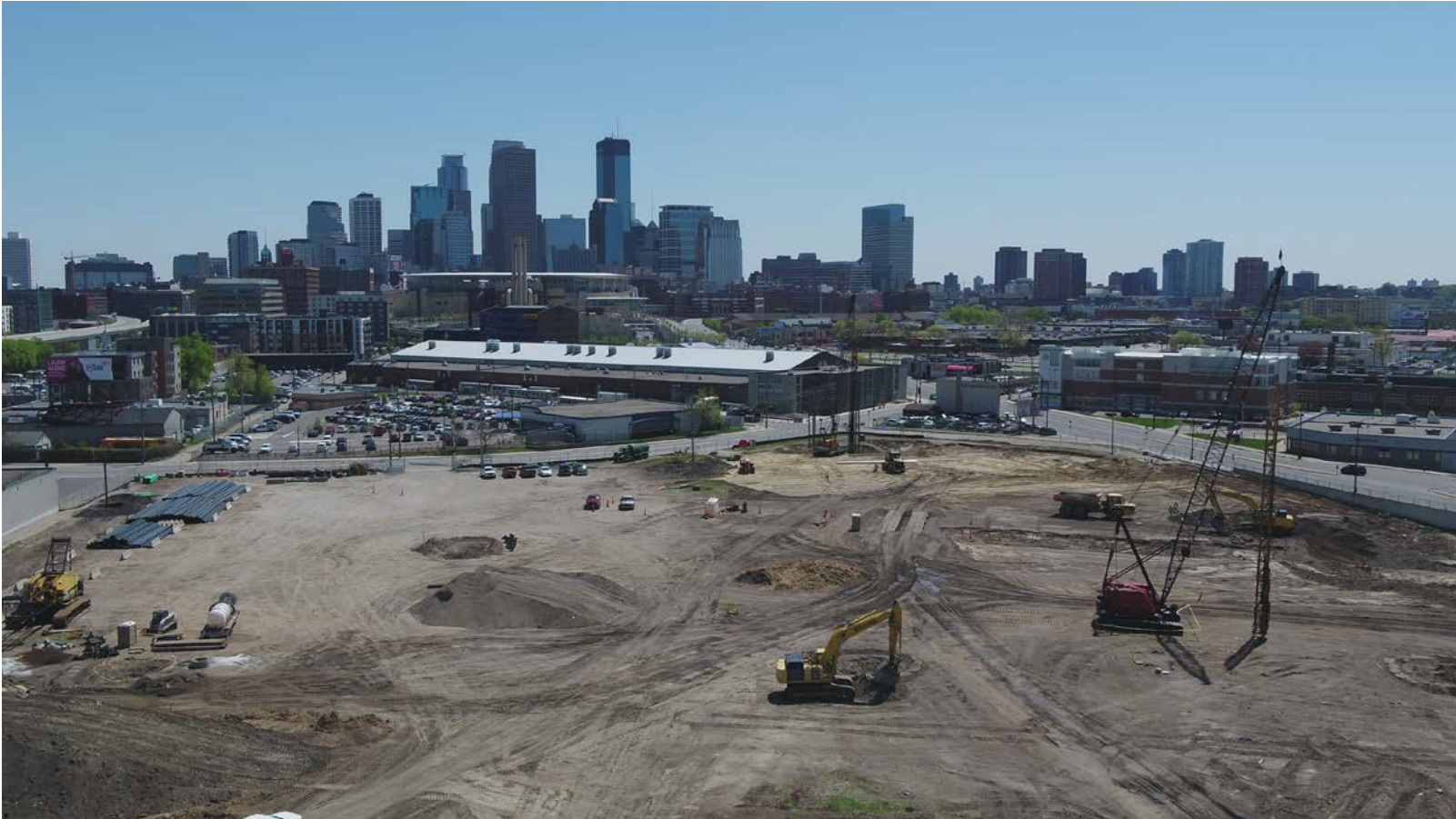
Week 2 of construction
