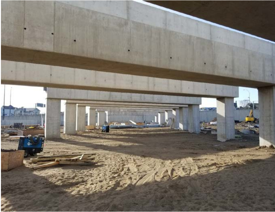
Transfer girders over Bassett Creek stormwater tunnel
