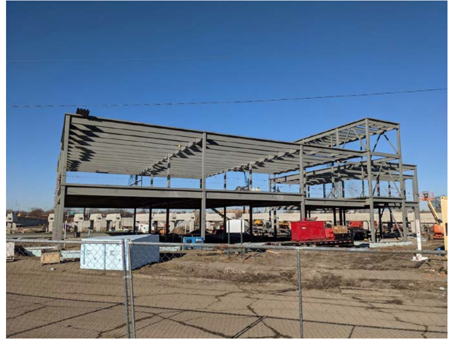
Floor slab forming, geothermal loop installation, steel erection for operations and admin building
