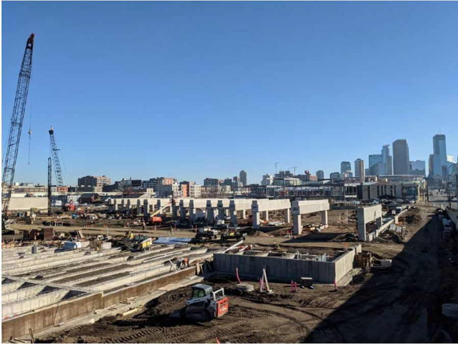
Floor slab forming, geothermal loop installation, steel erection for operations and admin building
