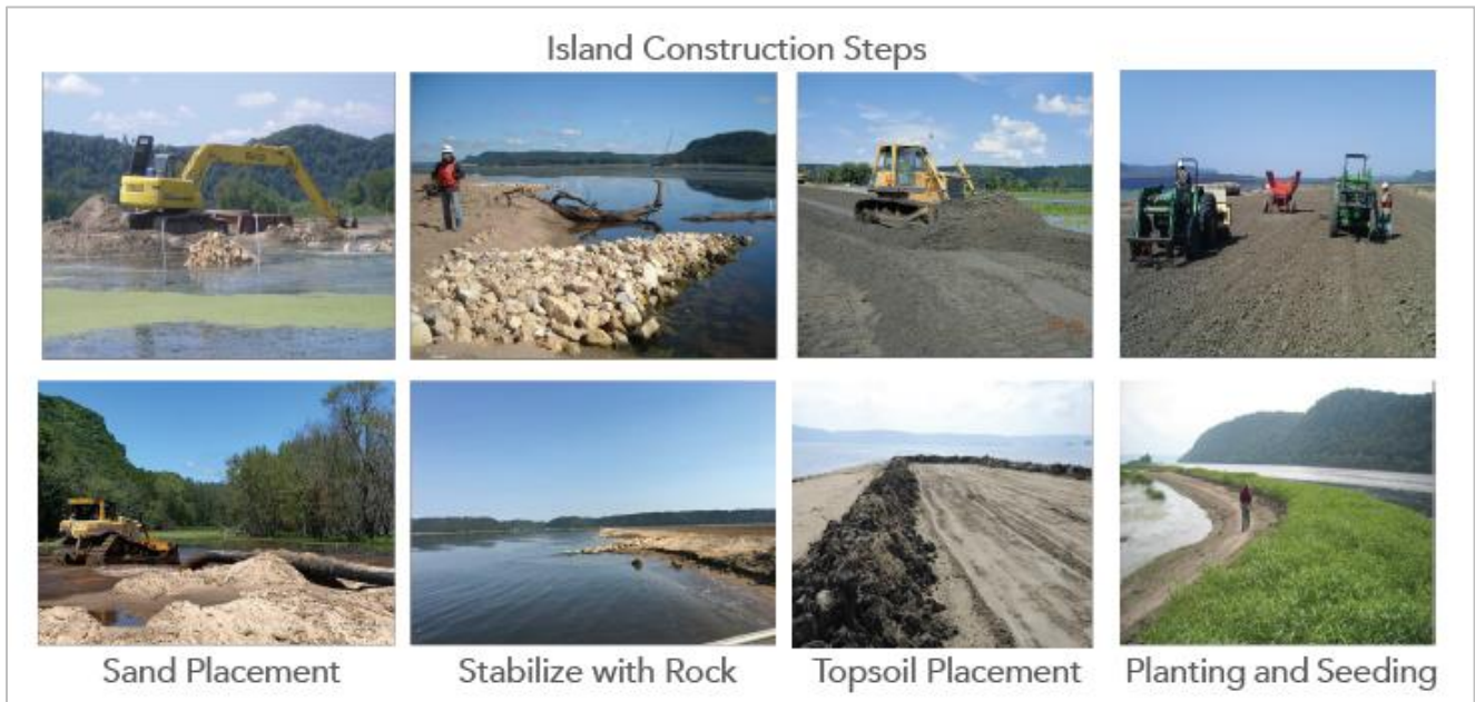
Figure 4: Island Construction Steps (MPA pg. 6)
