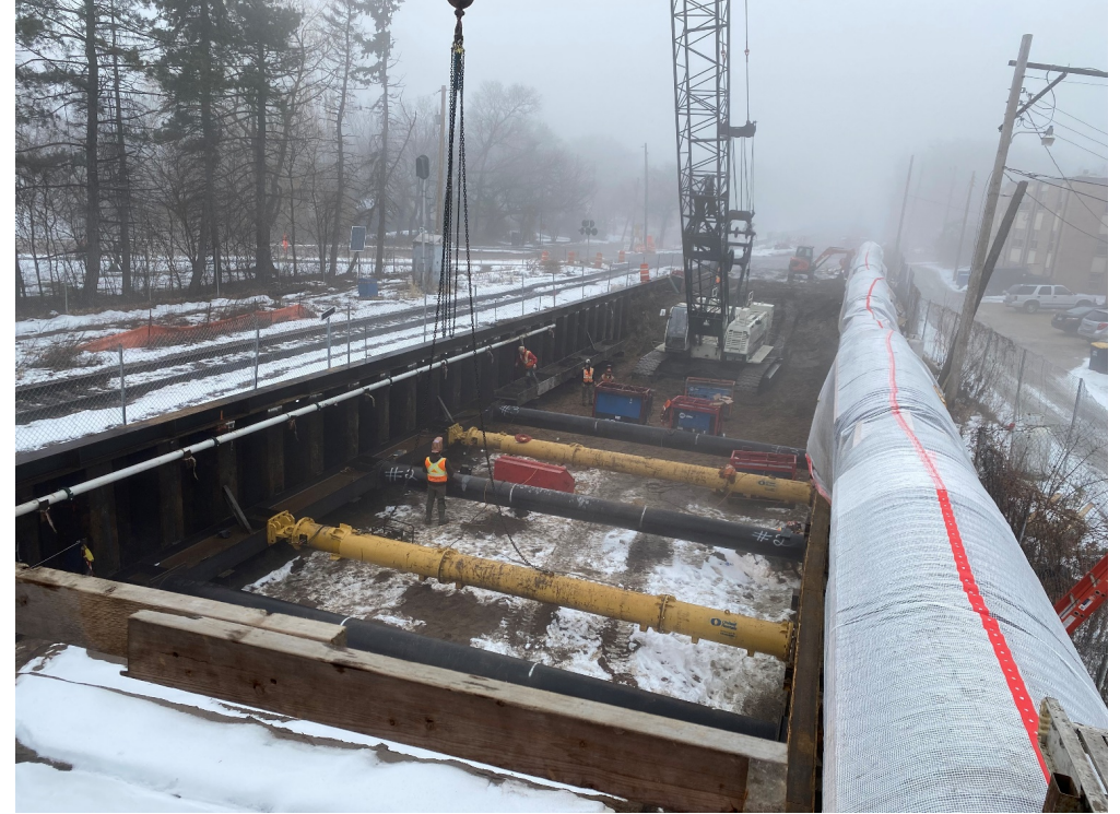
Kenilworth LRT tunnel excavation
