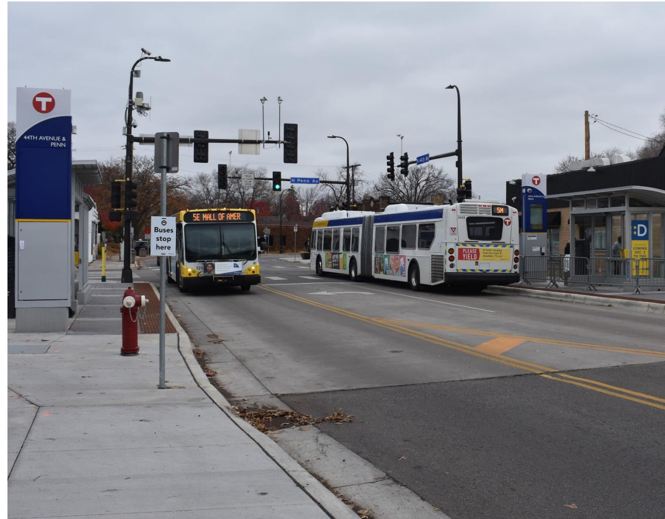
44th Avenue & Penn Station, built in coordination with Hennepin County's Webber 44 reconstruction project
