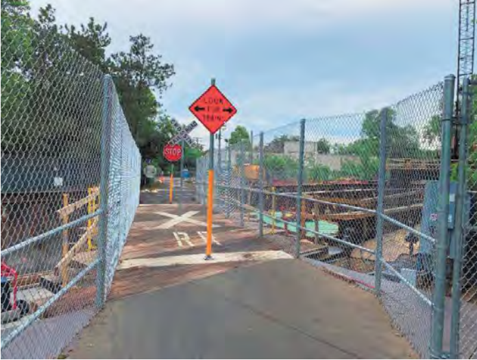
Temporary ped bridge over tunnel
