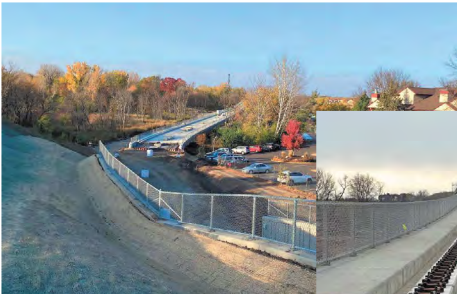
View to the North
