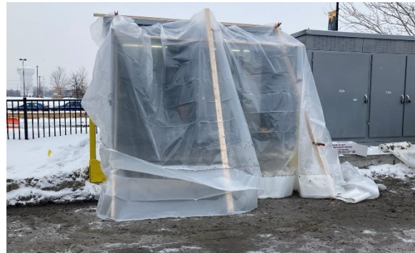
Figure 17: Temporary charger structure
