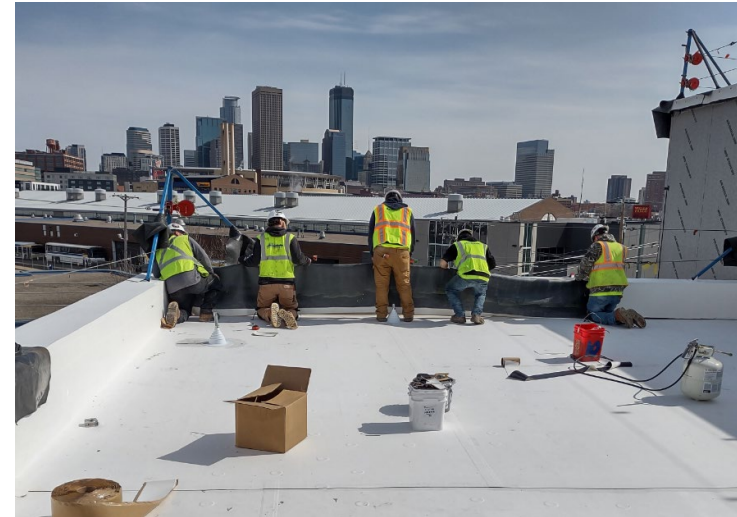
Roofing installation - DBE
