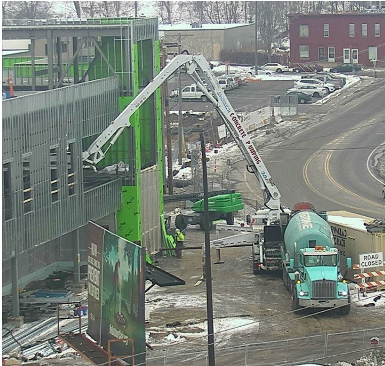
Concrete Pumping – DBE
