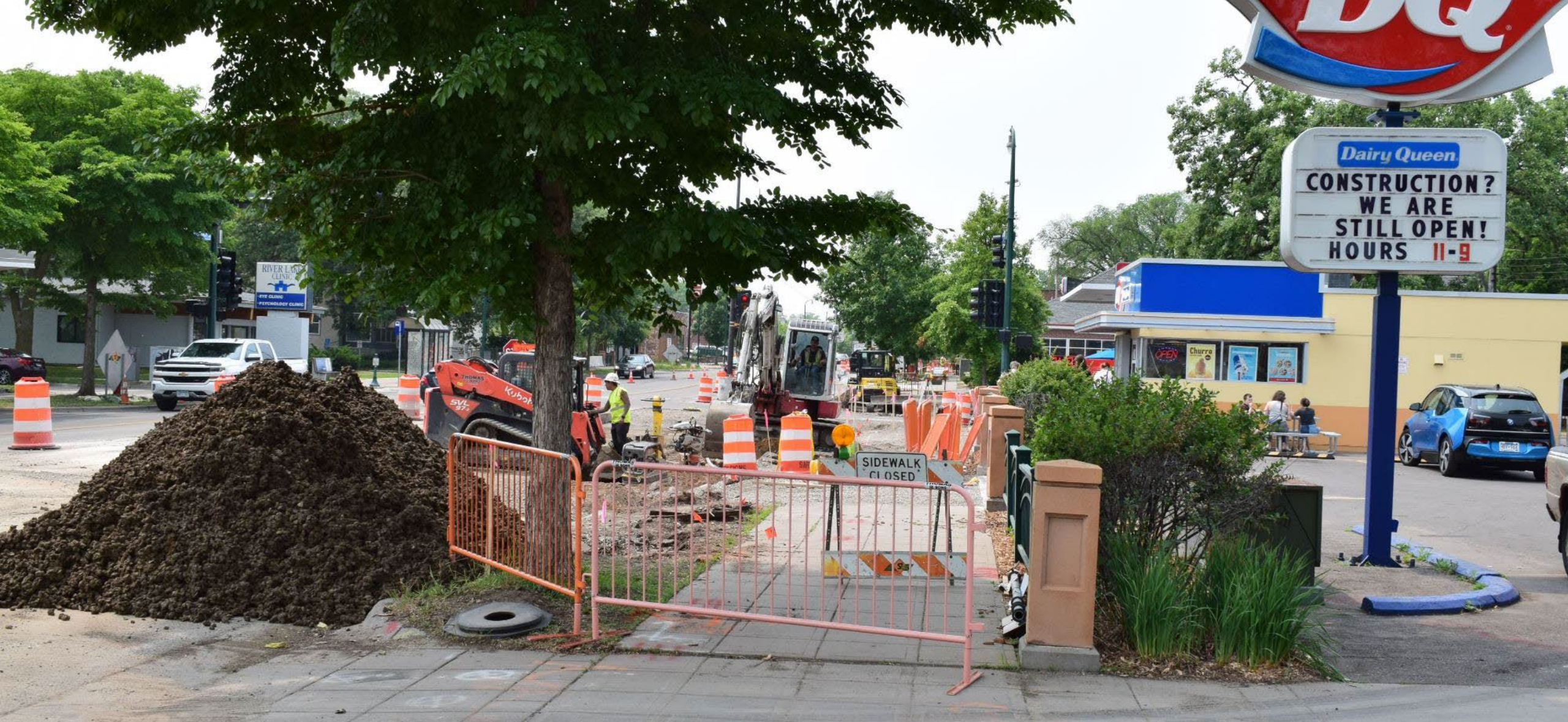
Station construction – Lake & 44th Avenue
