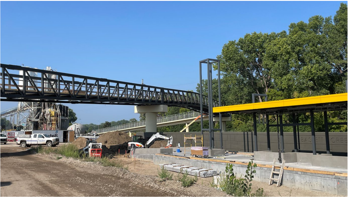
Luce Line Trail Bridge at Bassett Creek Valley Station
