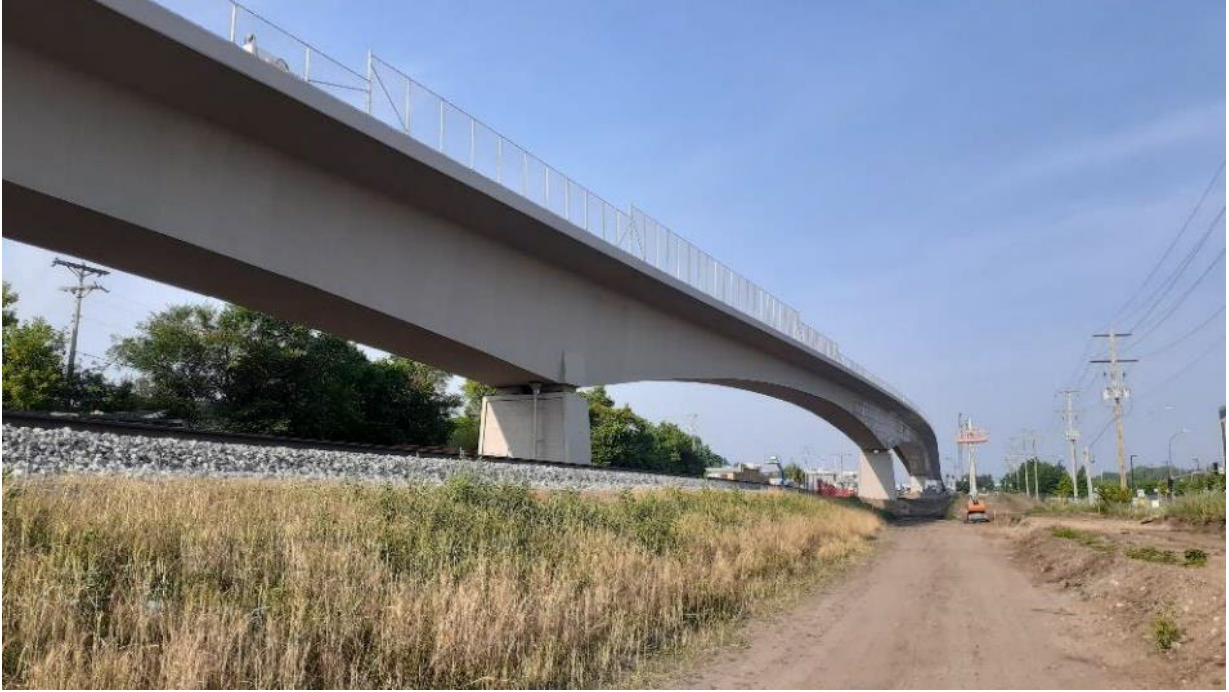
Excelsior Boulevard LRT Bridge
