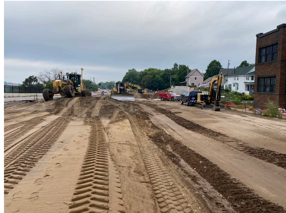
Guideway grading near Mounds Blvd
