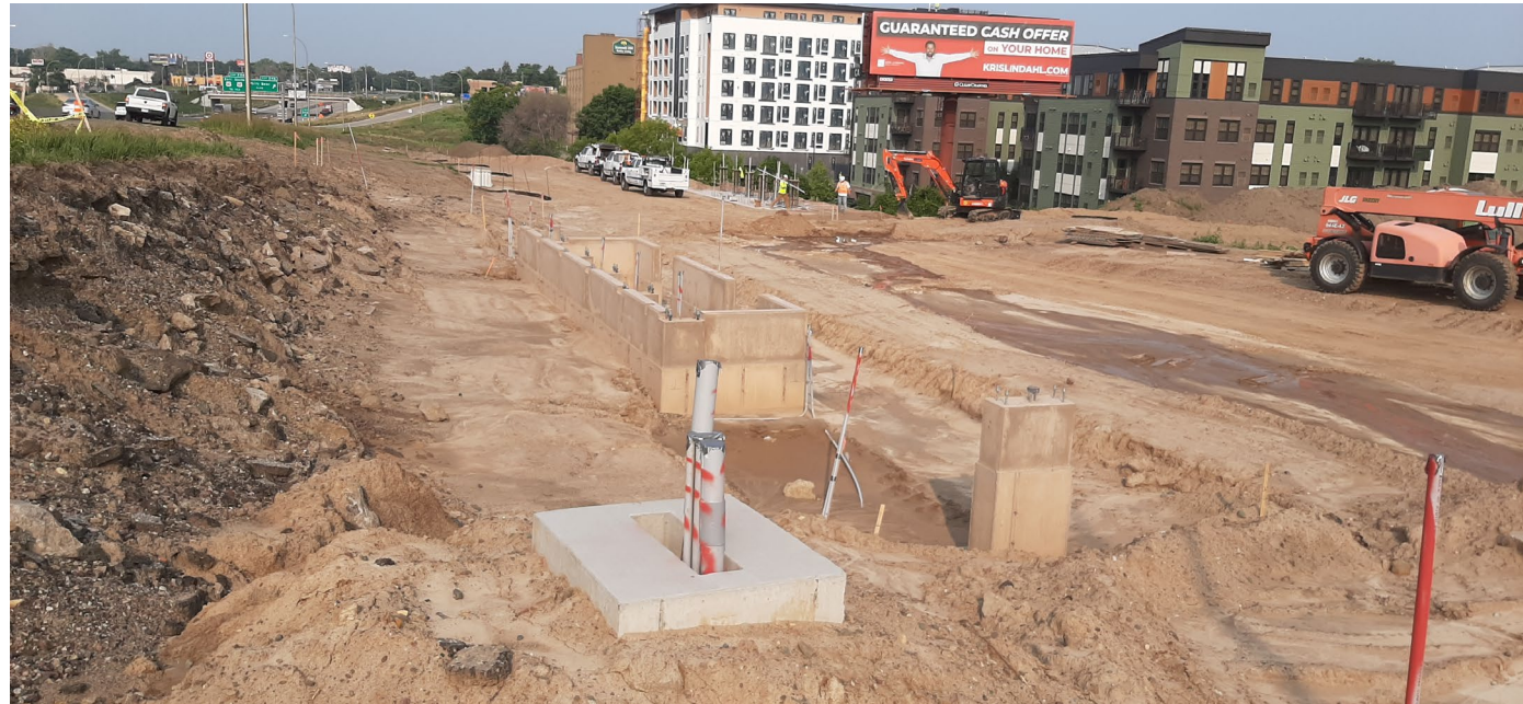
Hazel Station and Guideway grading
