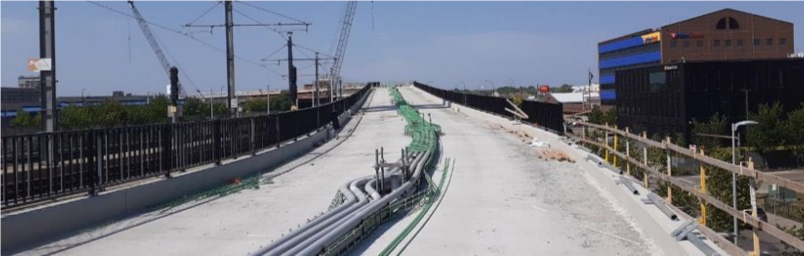
LRT Bridge over 5 th Avenue/7 th Street
