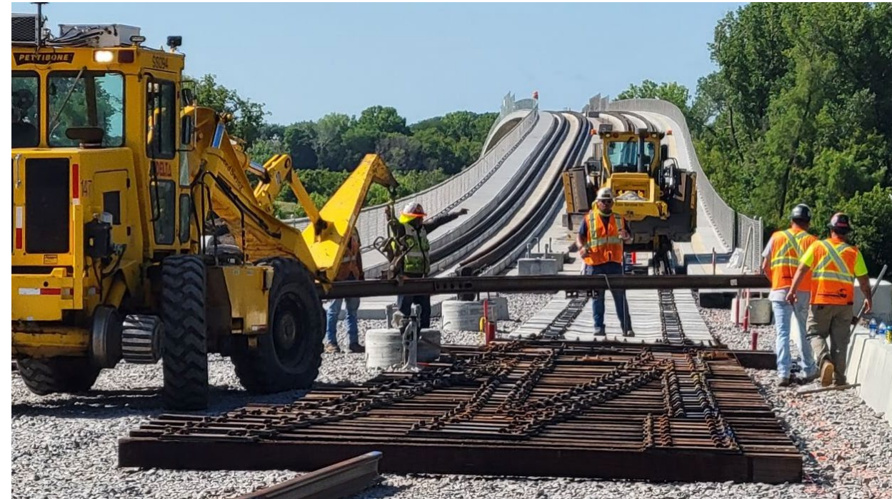
Special Trackwork at Minnetonka-Hopkins LRT Bridge
