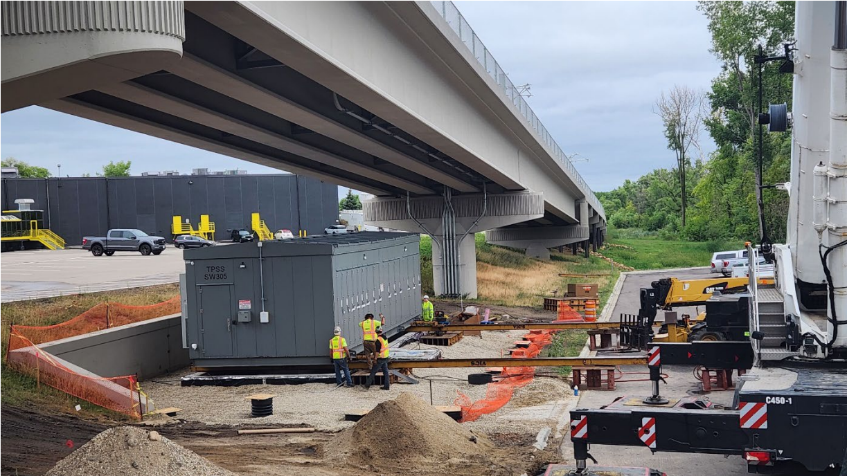
TPSS SW305 Installation in Eden Prairie
