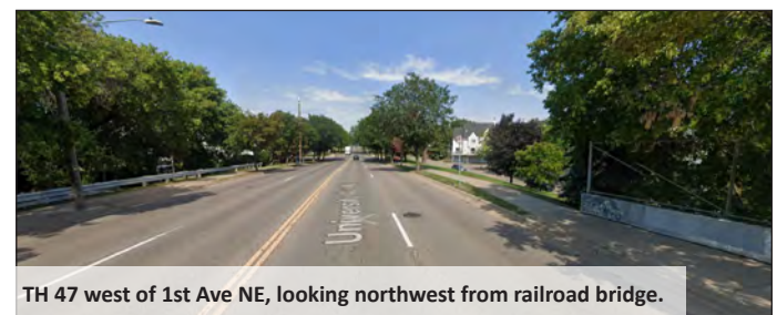
Unsignalized intersection of TH 47 and 7th Ave, looking east.
