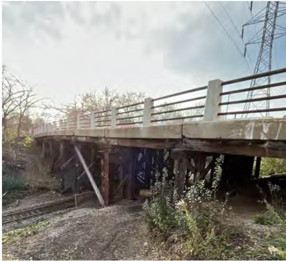
Cedar Lake Road Bridge 90471 over BNSF RR
