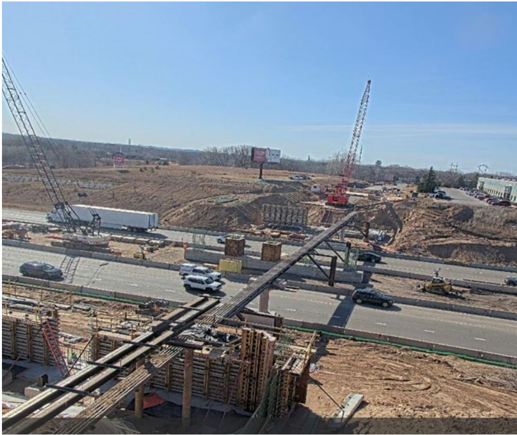
Temporary Utility Supports
