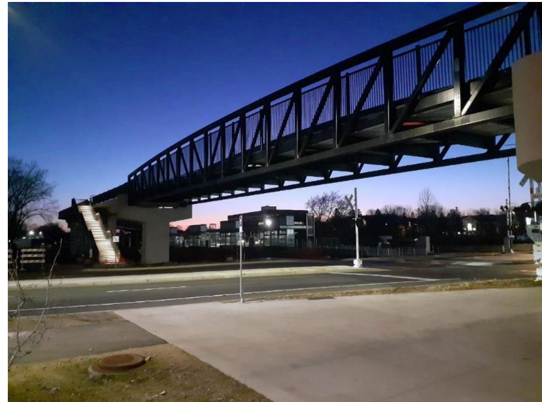
South Cedar Lake Trail Bridge adjacent to Beltline Boulevard Station
