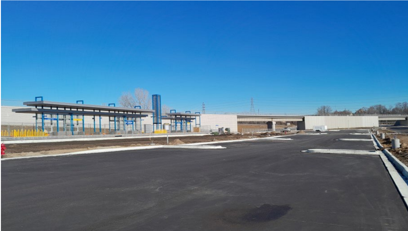
Louisiana Avenue Station
