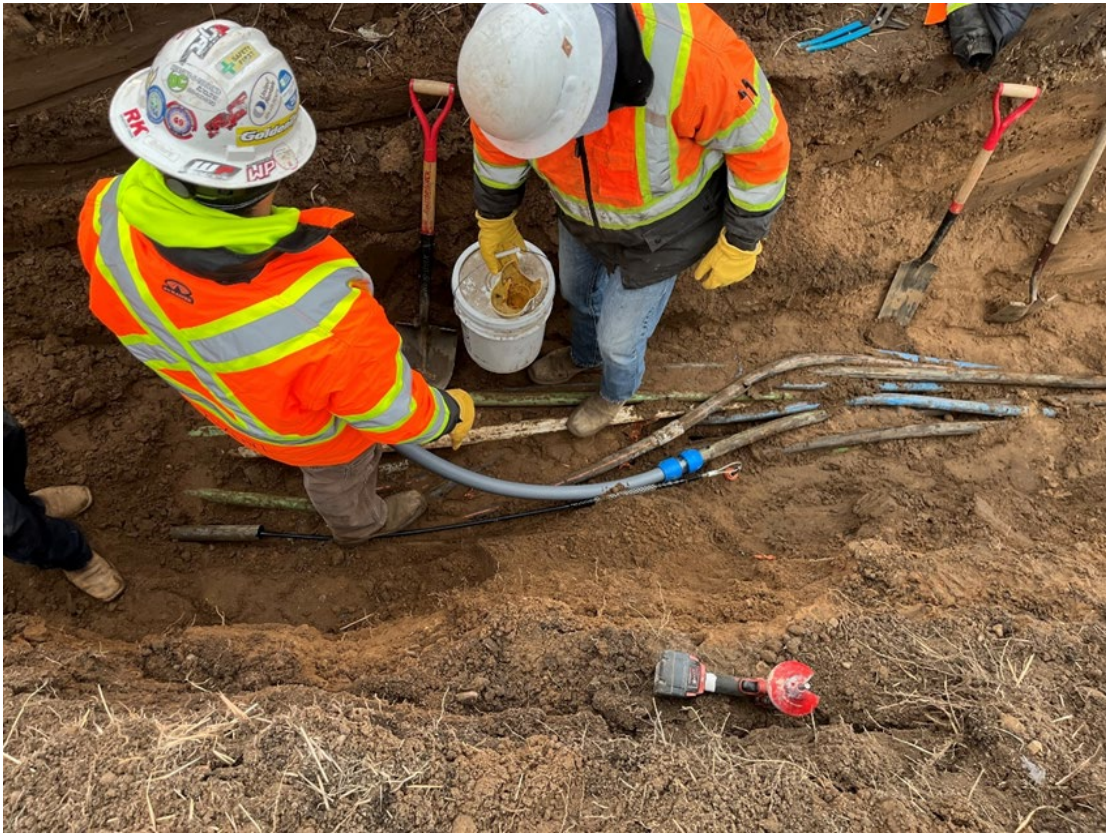
Oakdale—fiber install/splicing
