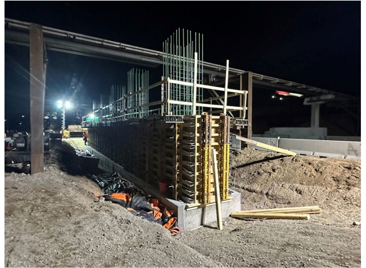
Median Bridge Piers
