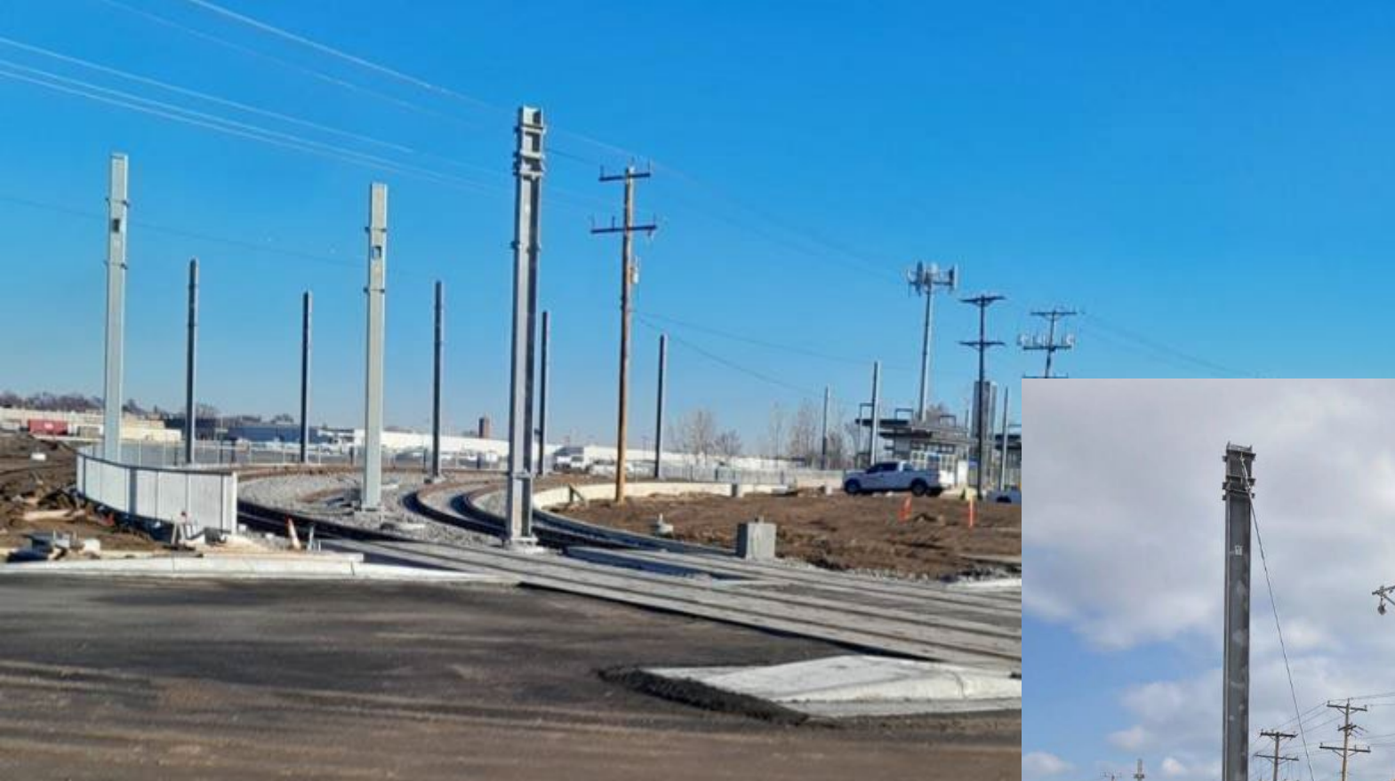
Overhead catenary pole installation near Shady Oak Station
