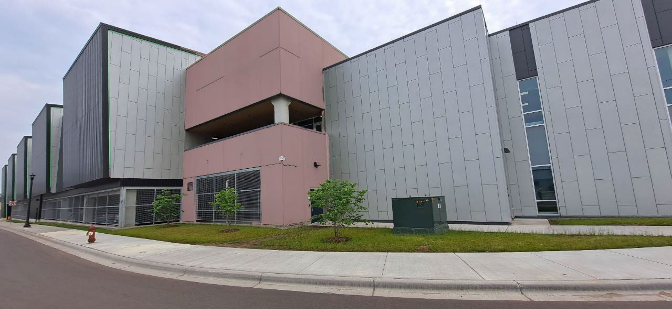
2025 North Loop Garage
