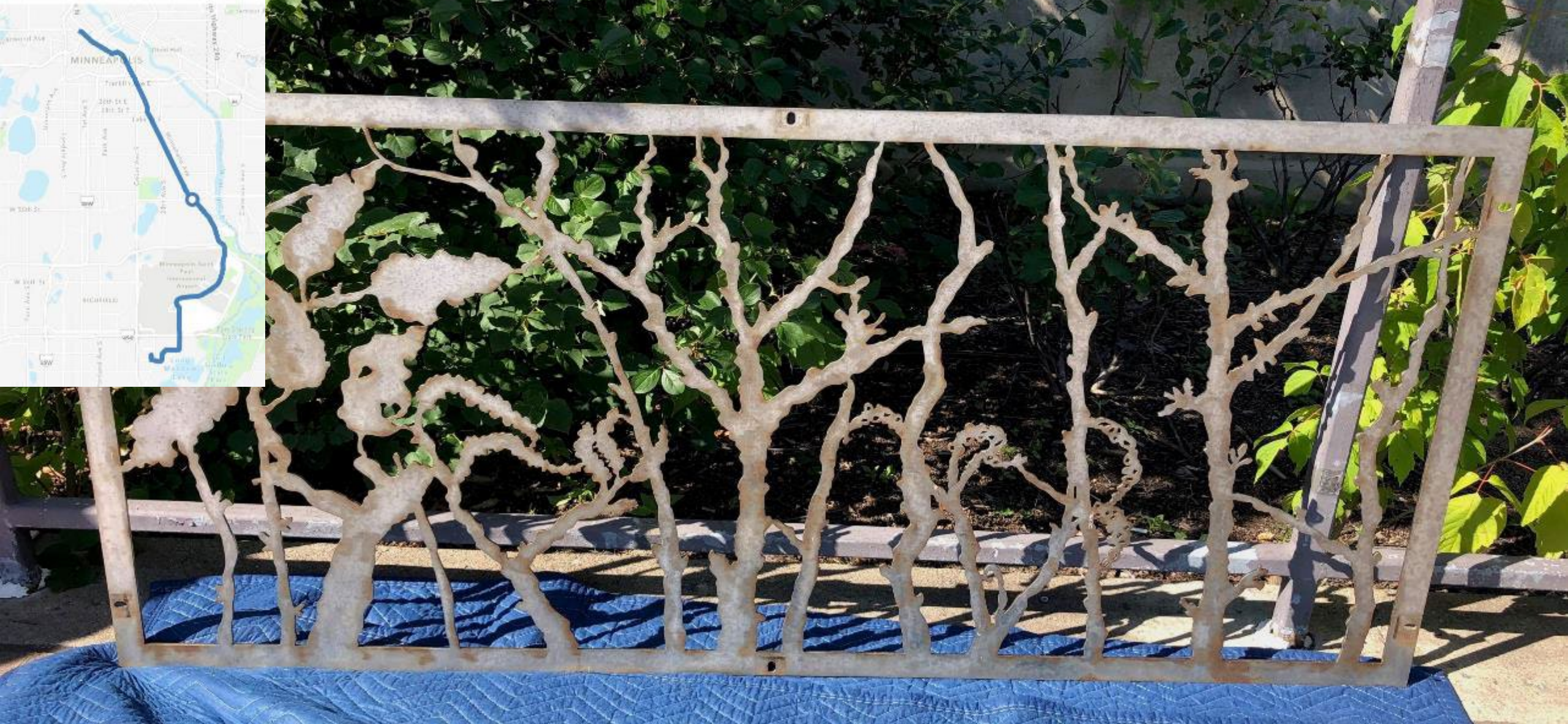
Stainless Steel Fence Repair – 50 th Street Station
