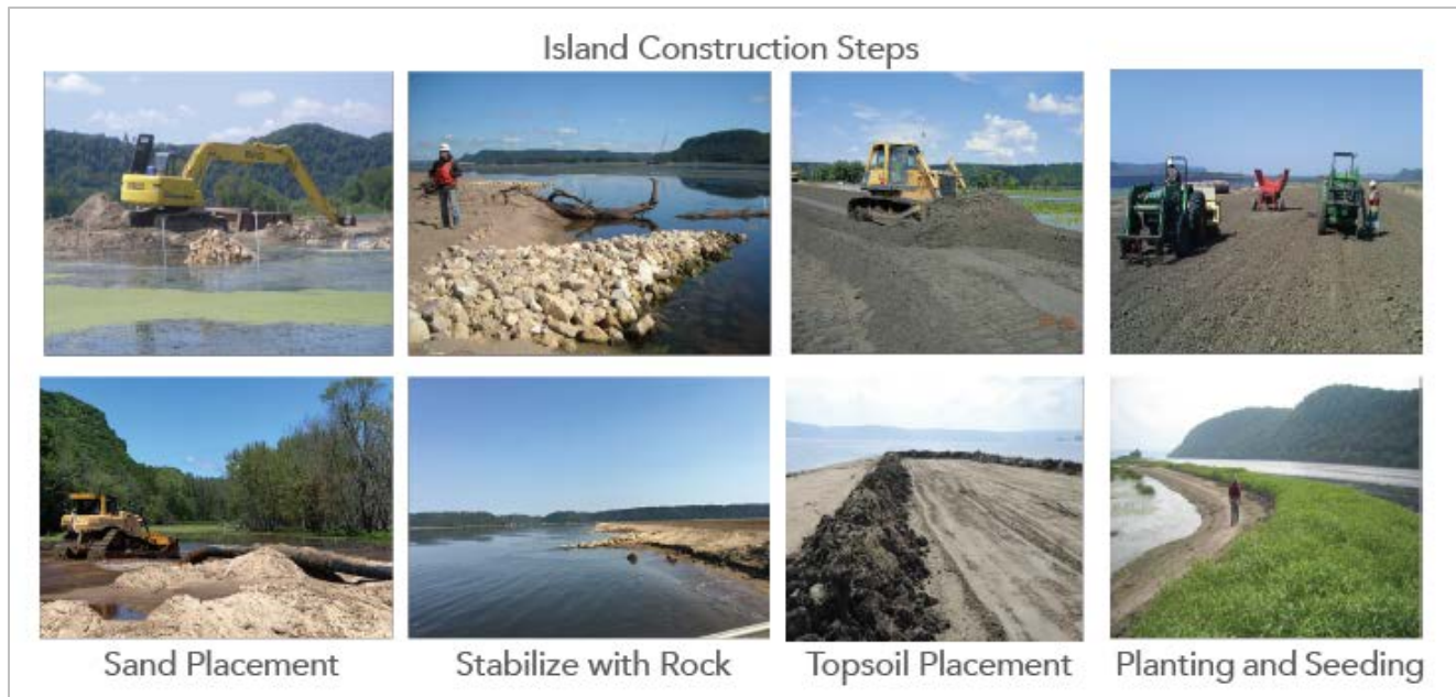
Figure 4: Island Construction Steps (MPA pg. 6)
