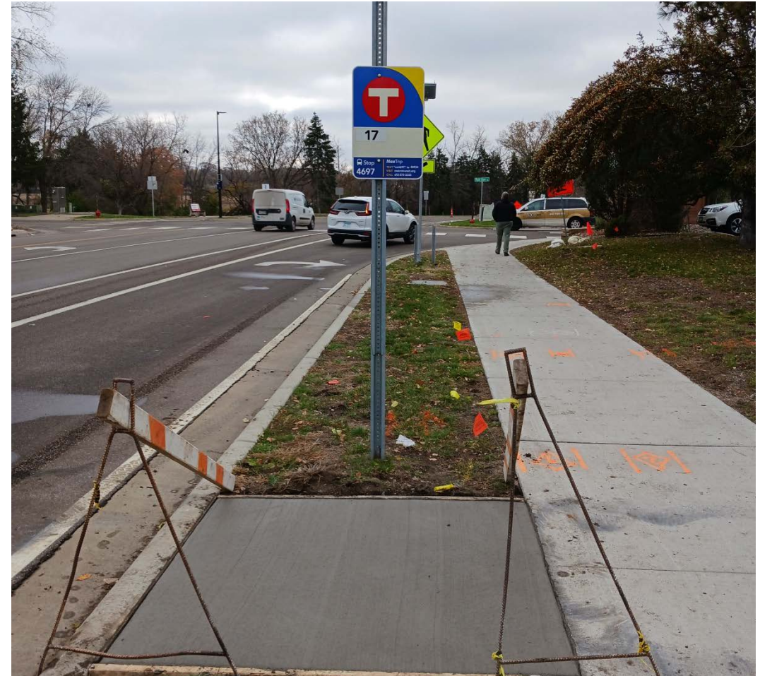
Construction of an accessible boarding area
