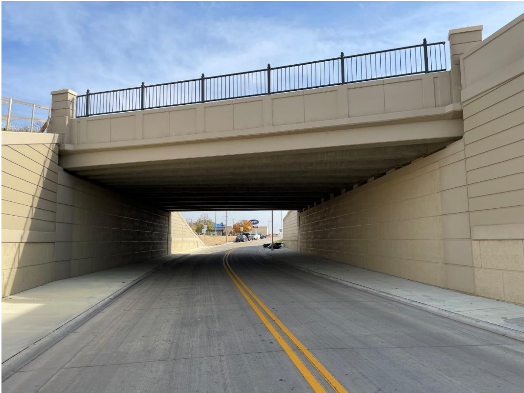
Ruth BRT Underpass, St. Paul
