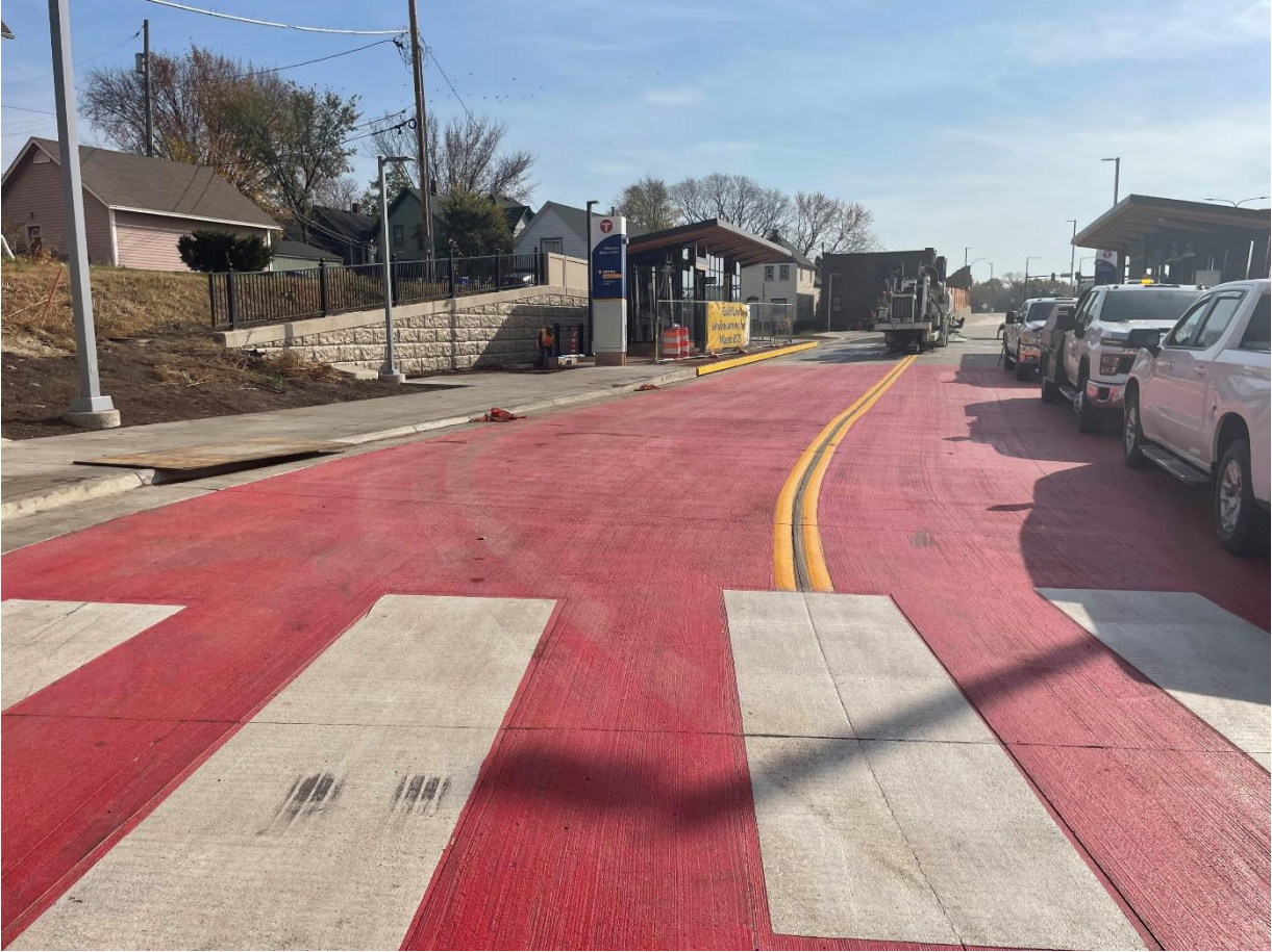
Mounds Blvd Station and BRT guideway, St. Paul
