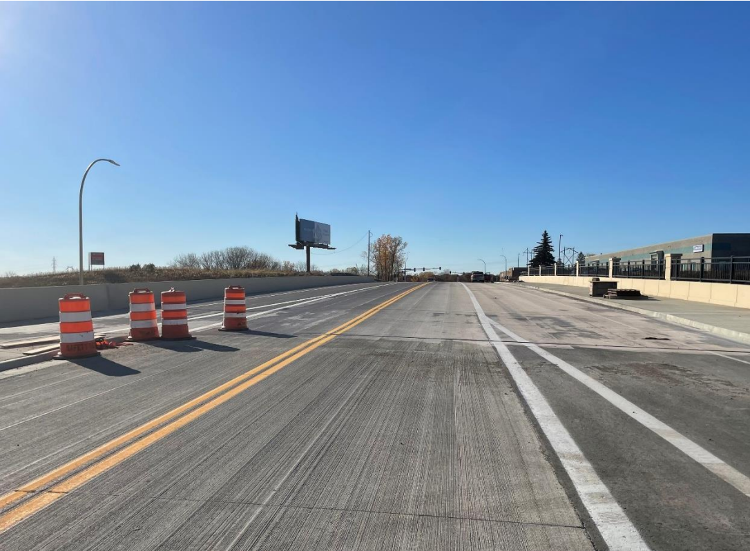
4 th Street Bridge, Oakdale
