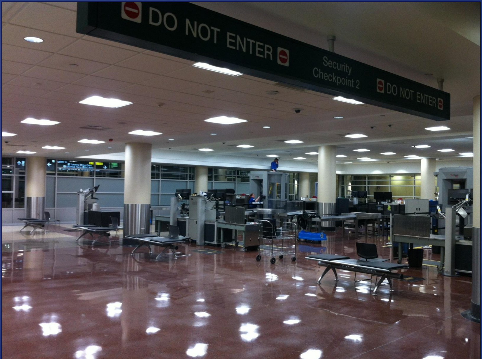
T2 - Humphrey Checkpoint #2 - Remodel
