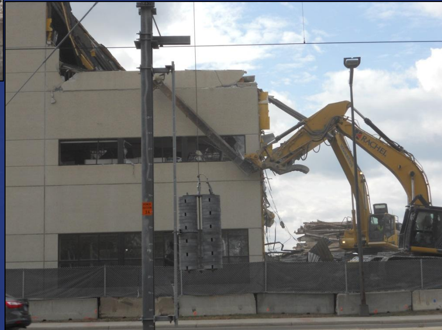
Building F Tower Demolition
