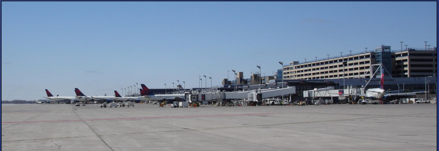
T1 - Lindbergh G Concourse Roof Replacement
