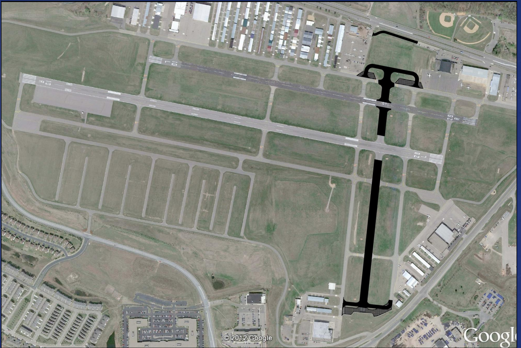
Flying Cloud Runway 18-36 Shift / Extension and Perimeter Road Construction
