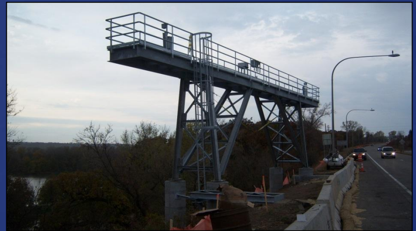
Runway 30R MALSF Approach Lighting System
