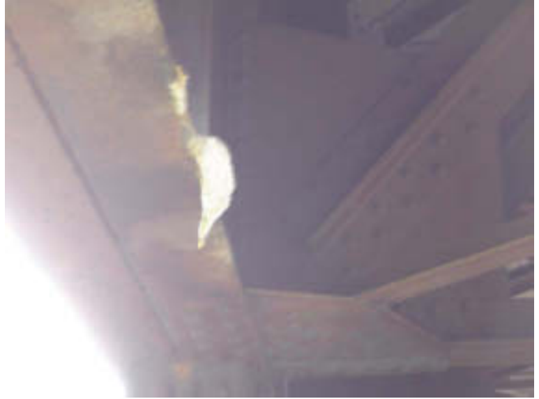
Span 5: Calcium Carbonate Built
