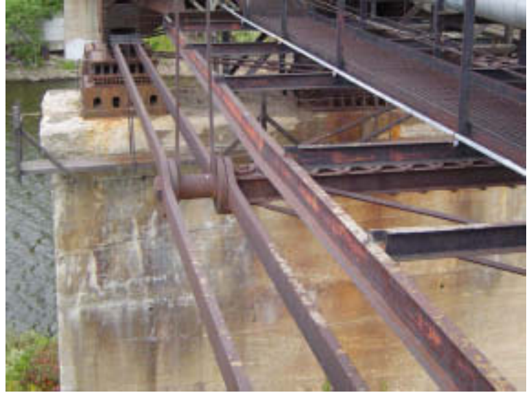
Span 4: Lower Chords
