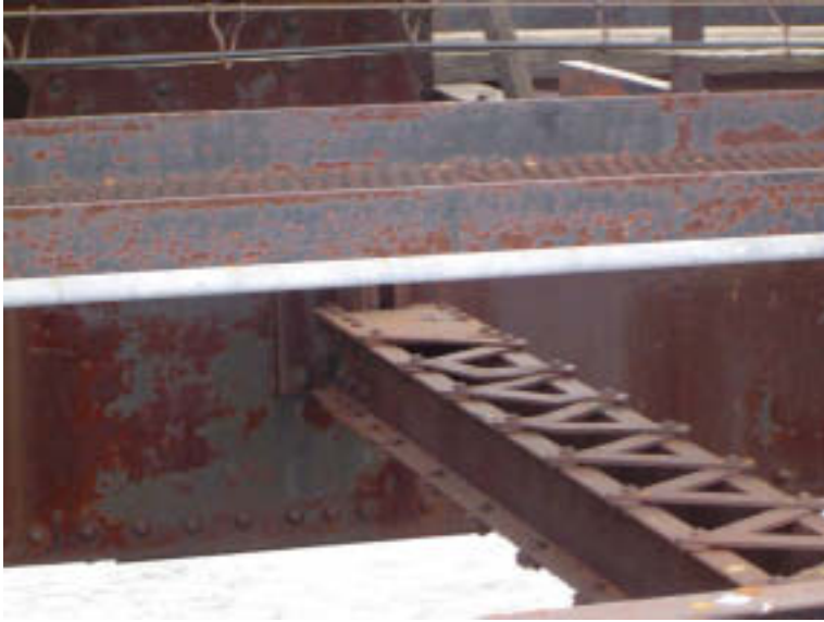
Span 4: Lower Chord Transverse Bracing
