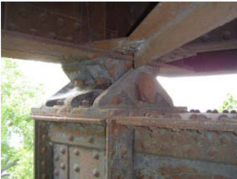
Pier 3: Steel Cap and Girder Span Bearing
