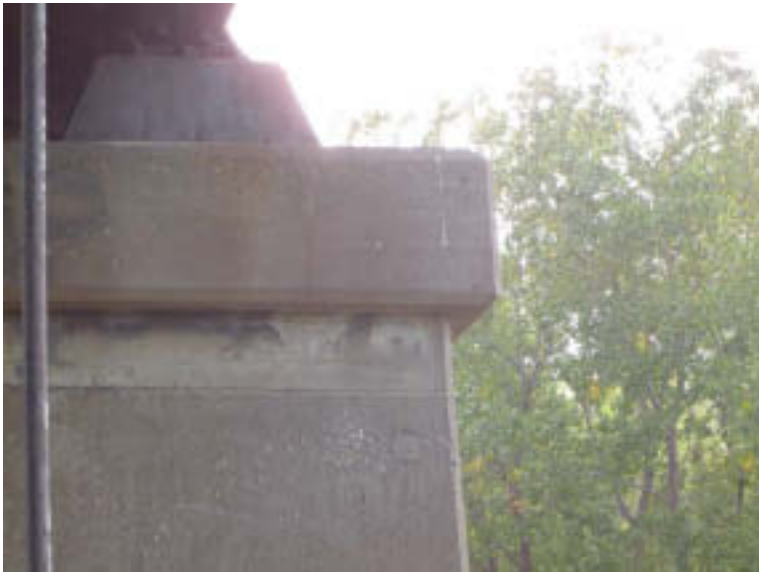
Pier 6: Pier Cap
