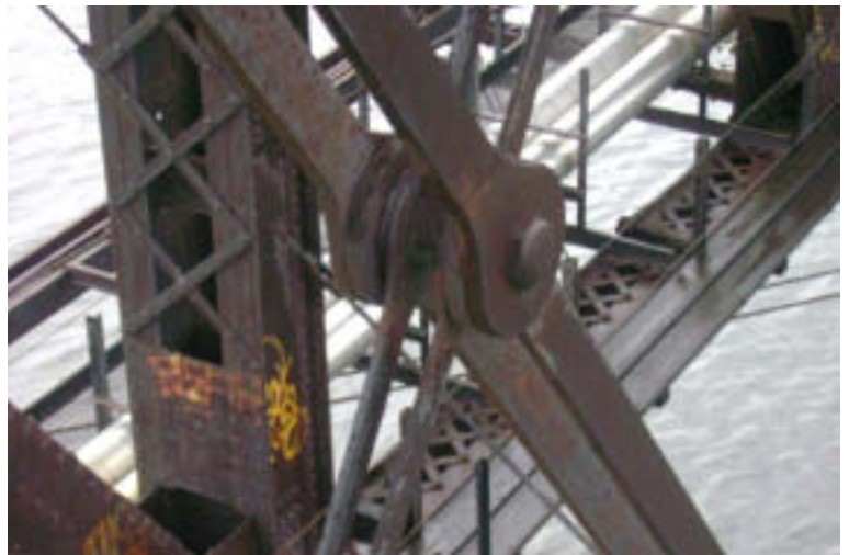
Span 4: Outside Truss Bracing
