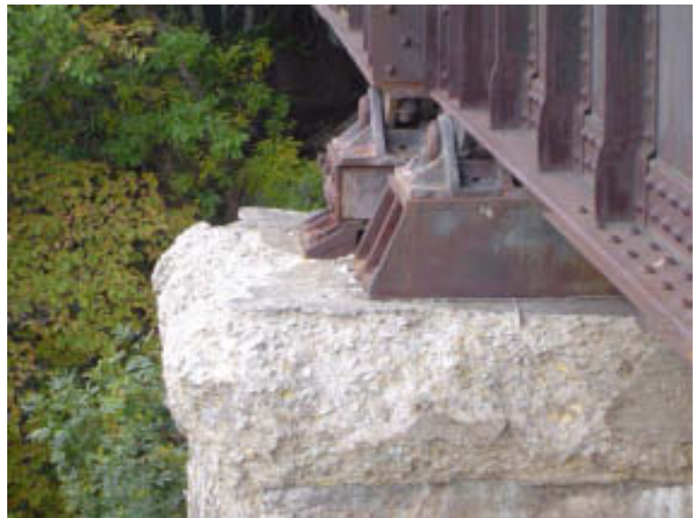
Pier 2: Pier Cap
