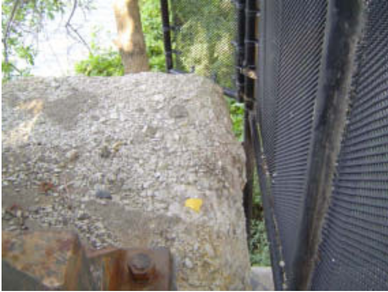
Pier 3: Lower Concrete Cap
