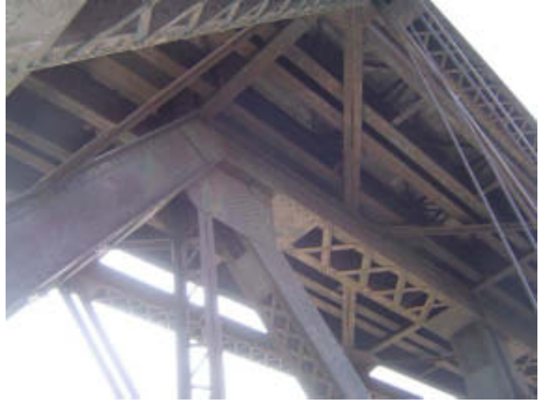
Span 3: Upper Chords
