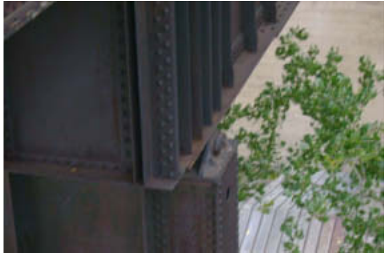
Pier 3: Upper Bearing
