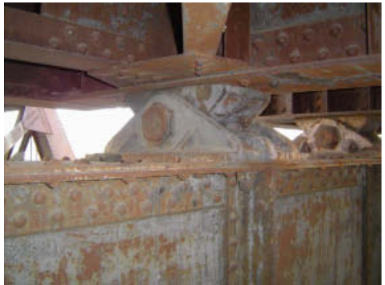
Pier 3: Steel Cap and Girder Span Bearing
