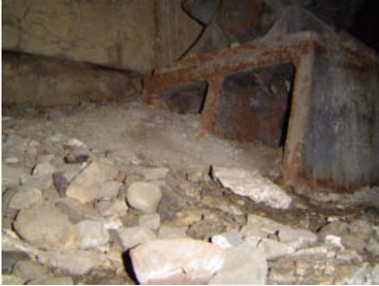
Abutment 1: Abutment Seat
