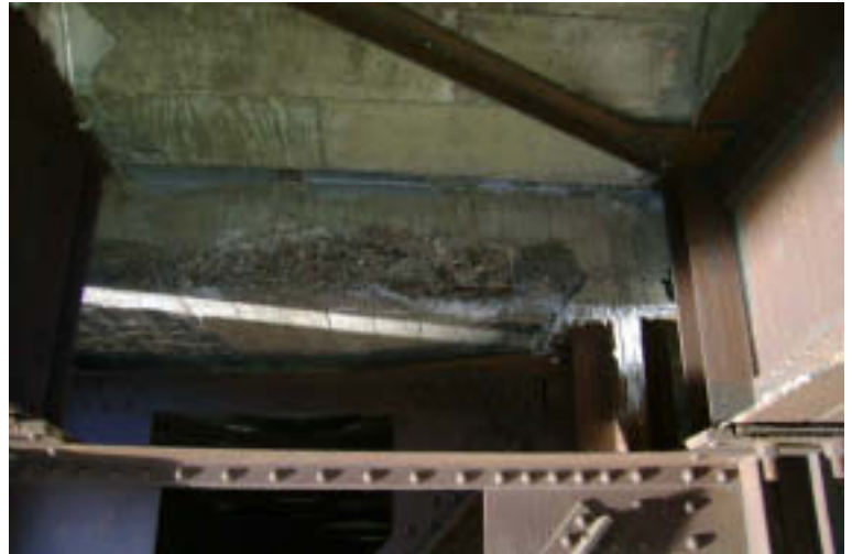
Pier 5: Expansion Joint
