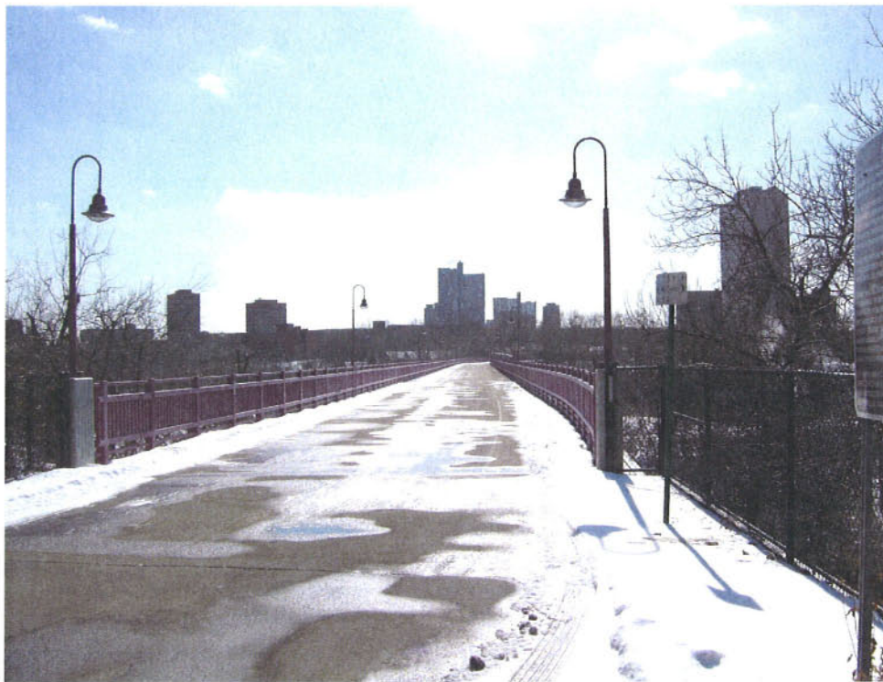
Looking West at East Abutment of Bridge No. 9
