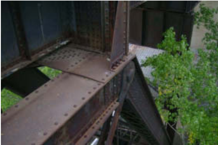
Span 3: Upper Chords Members
