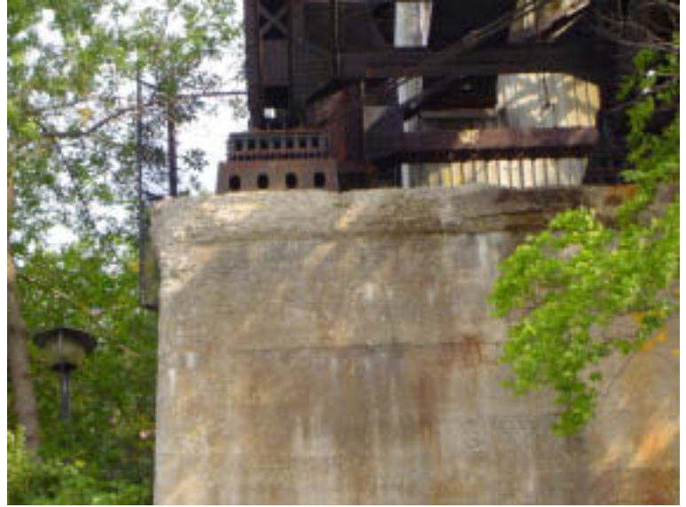
Pier 3: Concrete Pier
