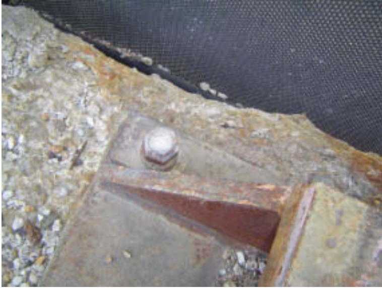
Pier 5: Concrete Cap Edge and Bearing
