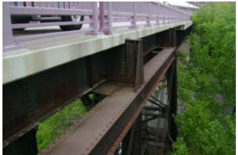
Span 3: Upper Chords
