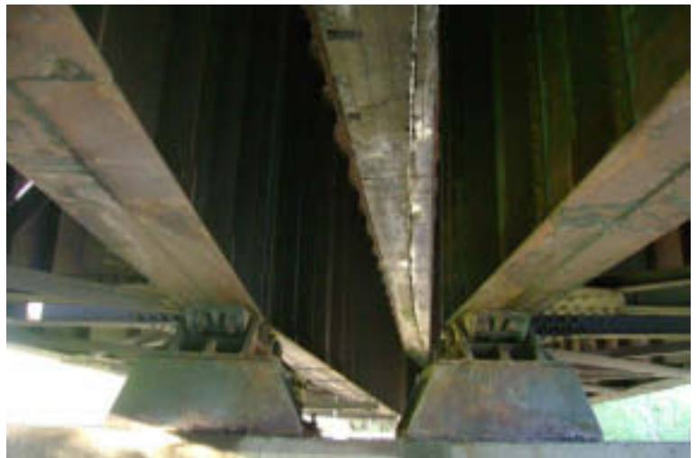
Span 6: Center Line of Deck
