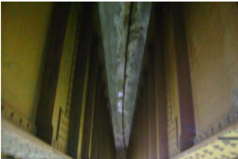
Span 7: Center of the Deck
