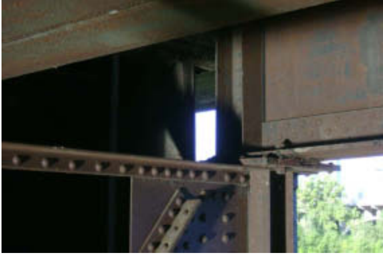
Pier 5: Truss Span Bearing
