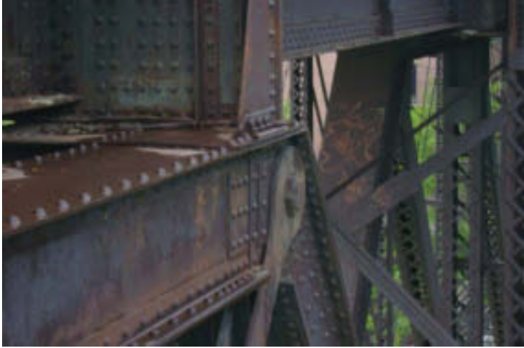
Span 3: Upper Chord
