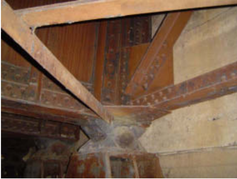
Abutment 1: Bearing
