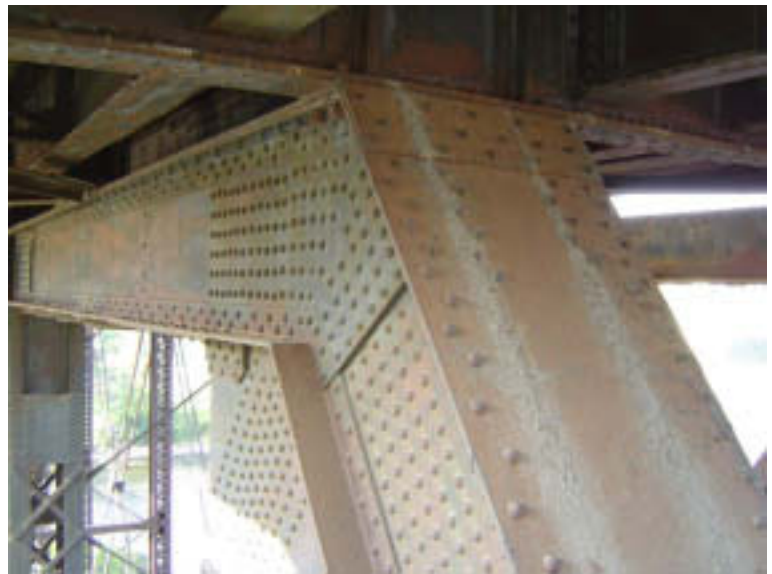
Span 3: Center Truss
