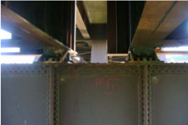
Pier 5: Steel Cap
