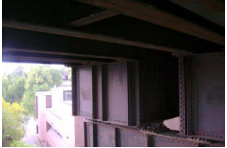
Pier 3: Upper Steel Cap
