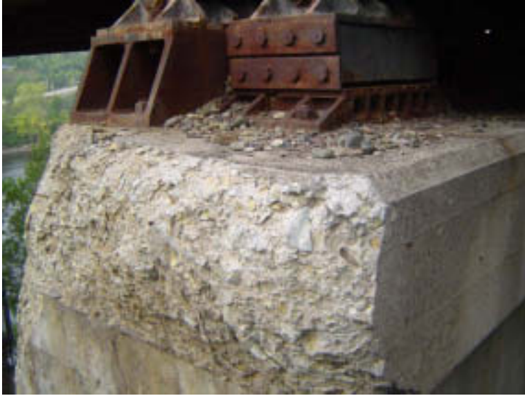
Pier 2: Pier Cap
