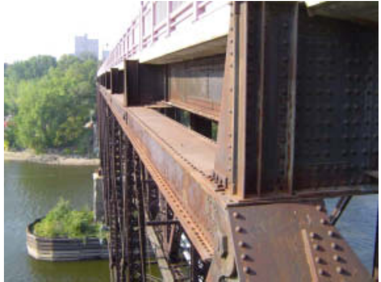
Span 3: Upper Truss Members
