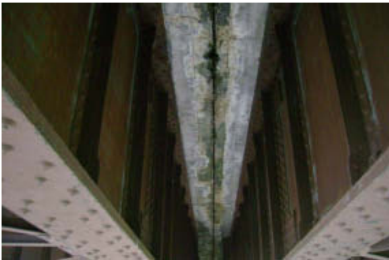
Span 2: Under Side Center of Deck
