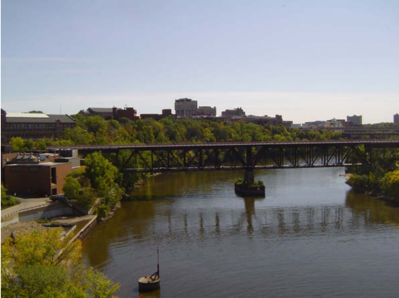
Elevation Photo: Looking South Towards Bridge No. 9
