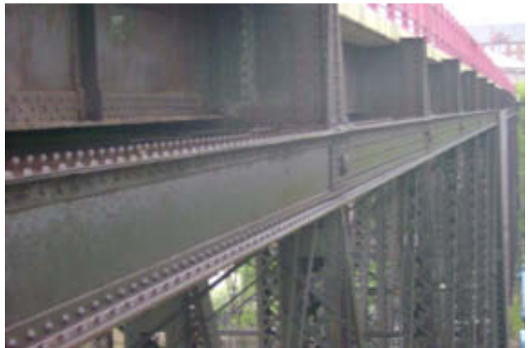
Span 4: Upper Chords: Floor Beams and Stringers
