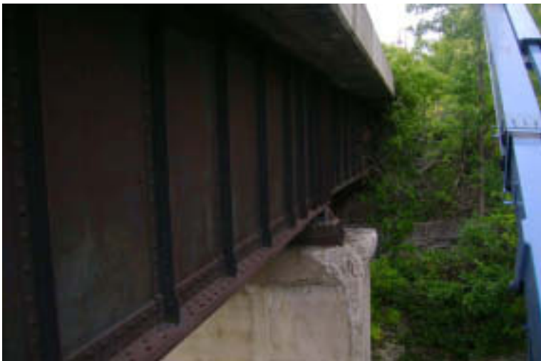
Pier 2: Pier Cap
