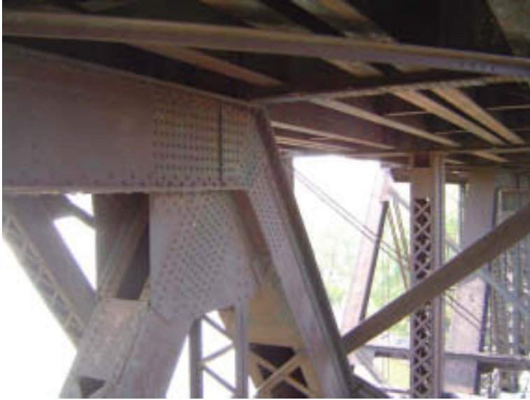
Span 3: Center Truss
