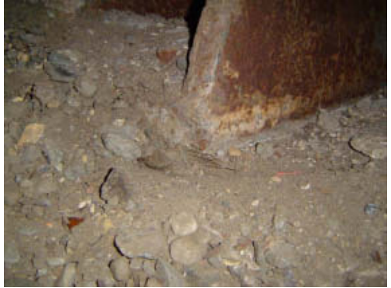
Abutment 1: Abutment Seat
