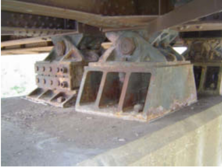
Pier 6: Pier Cap
