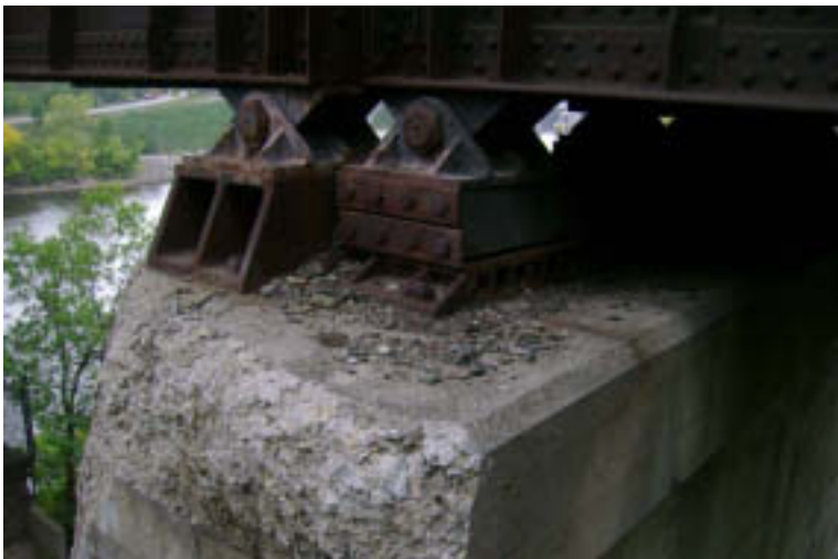
Pier 2: Pier Downstream Side
