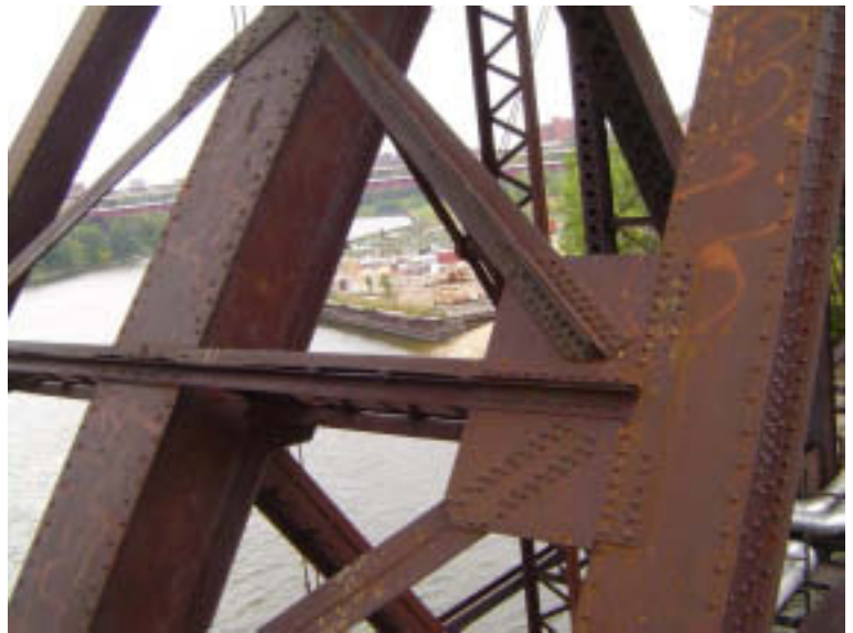
Span 4: Diagonal Members
