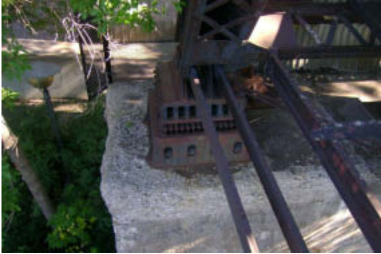
Pier 3: Concrete Cap and Bearing
