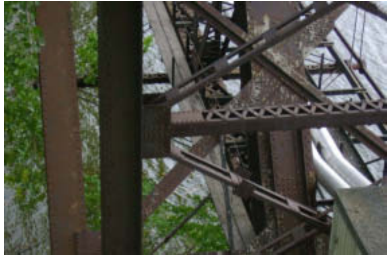
Pier 3: Steel Column Bracing
