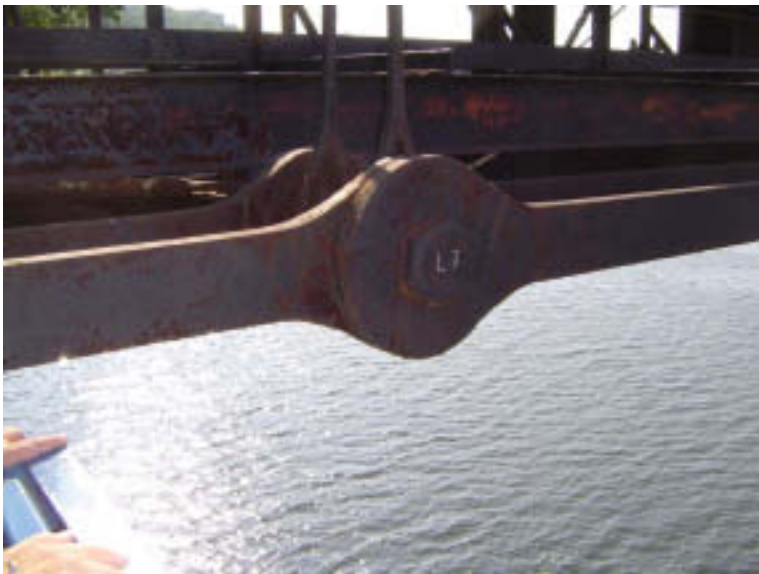
Span 3: Bottom Chords
