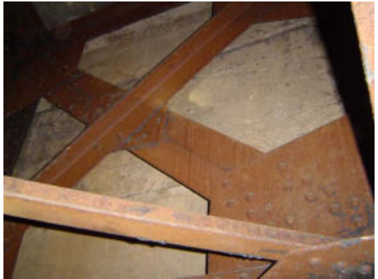
Abutment 1: Stem Wall
