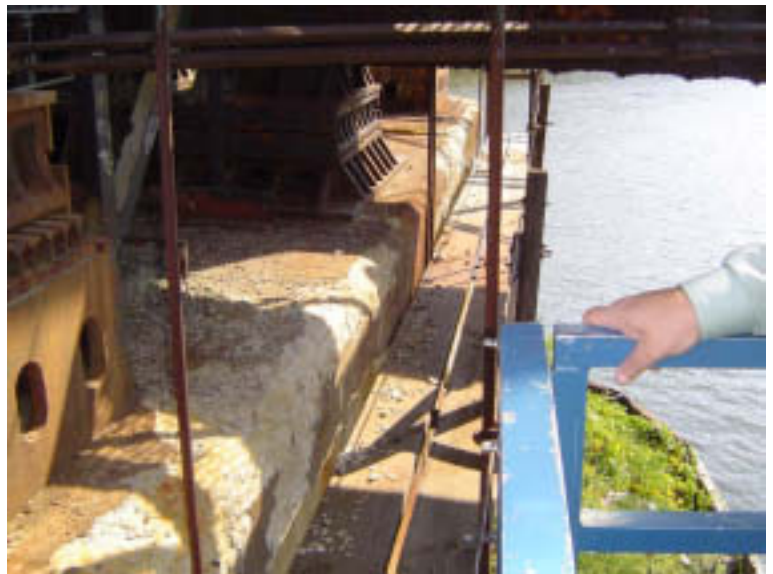
Pier 4: Pier Cap
