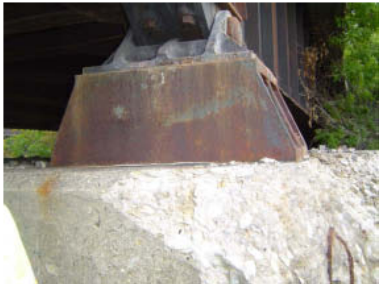
Pier 2: Pier Cap
