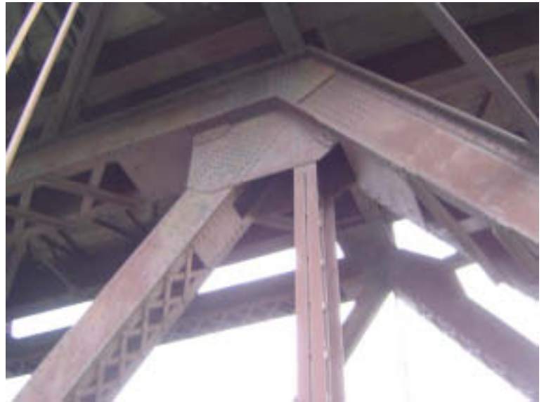
Span 4: Center Truss
