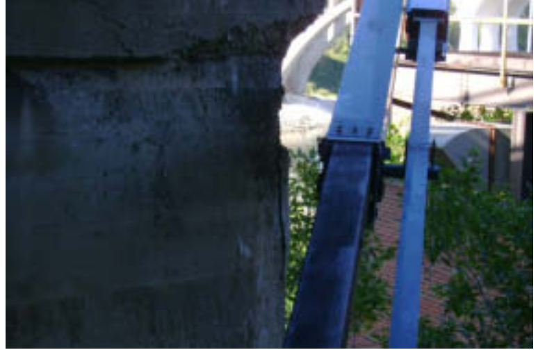
Pier 2: Pier Column Upstream
