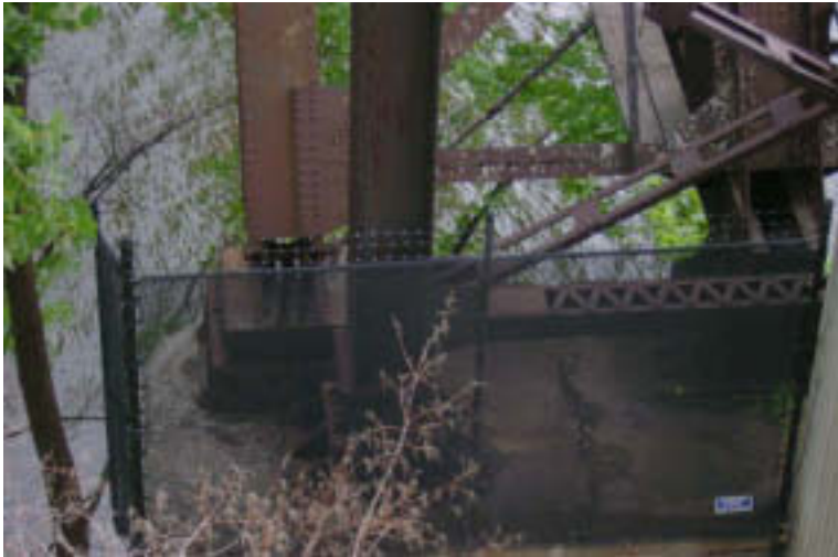
Pier 3: Lower Concrete Cap
