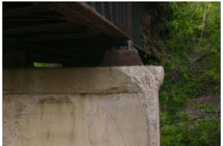
Pier 2: Pier Cap
