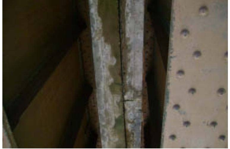
Span 5: Center Line of Deck
