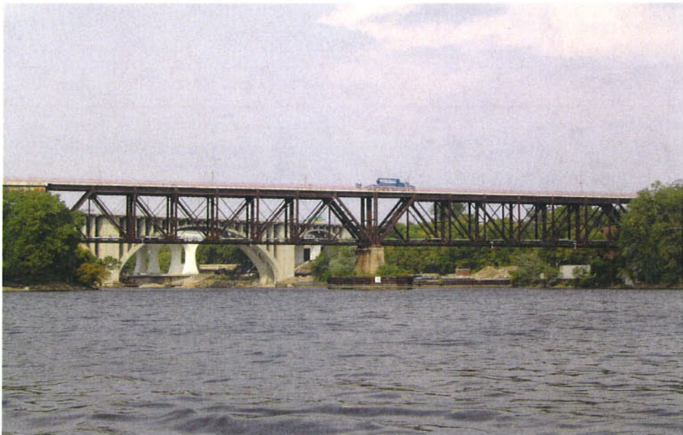
Looking North Towards Bridge No. 9
