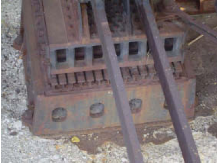
Pier 3: Concrete Cap and Bearing
