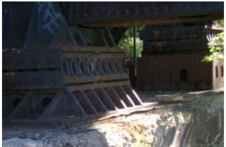
Pier 3: Bearing and Concrete Cap
