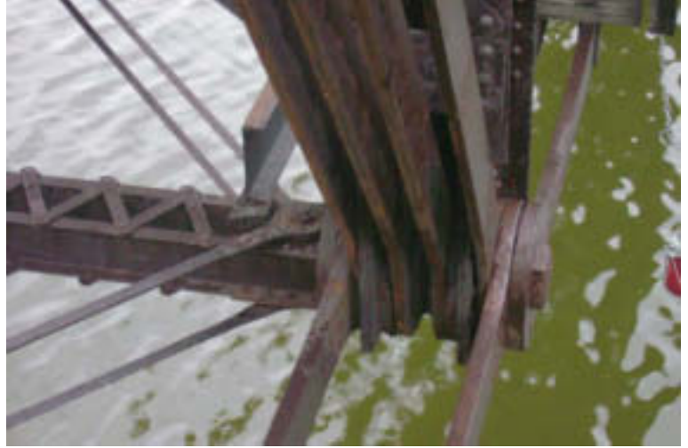
Span 4: Bottom Chord Connection
