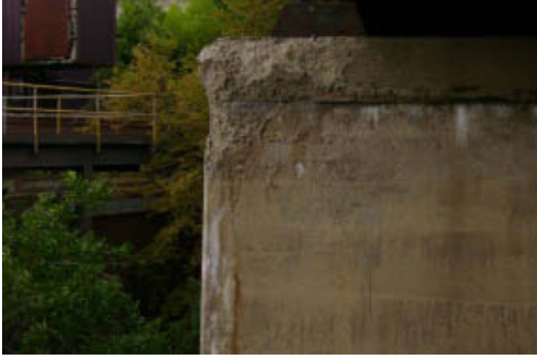
Pier 2: Pier Cap
