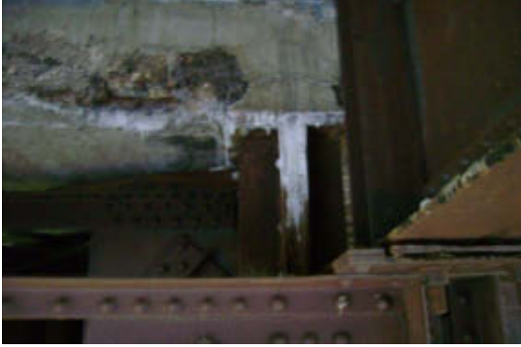
Pier 5: Expansion Joint
