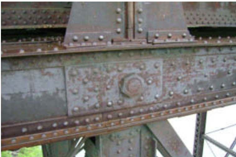
Span 4: Upper Chord Connection
