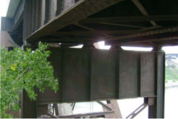
Pier 3: Steel Cap
