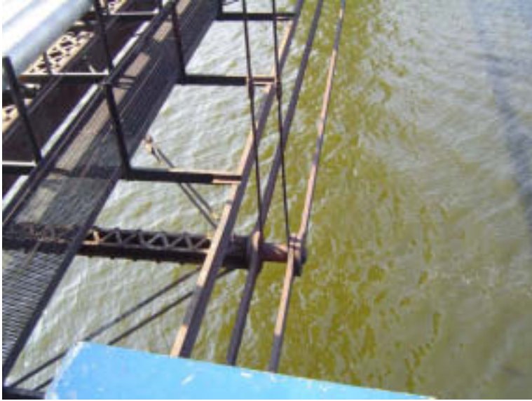
Span 3: Bottom Chords
