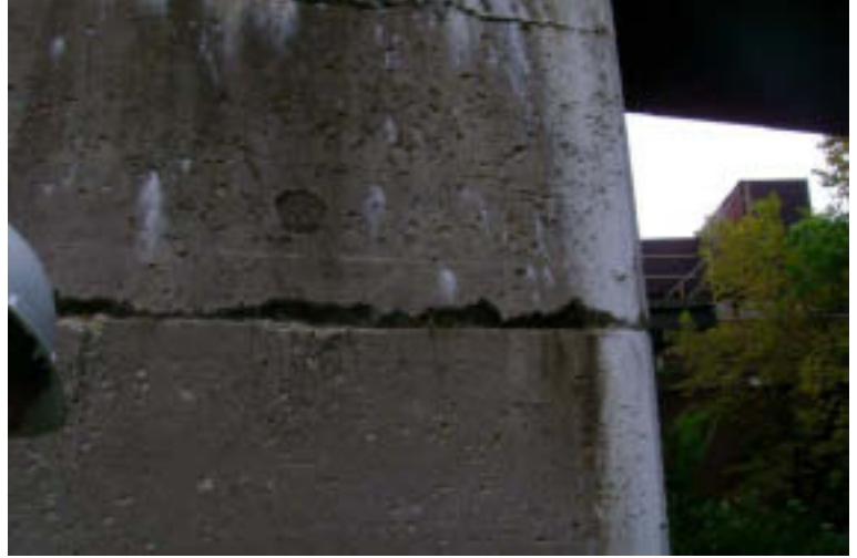
Pier 2: Pier Column
