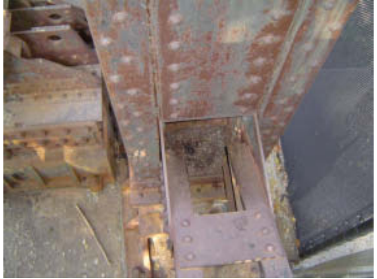
Pier 3: Concrete Cap
