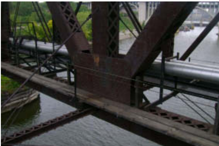
Span 3: Center Truss Lower Connection
