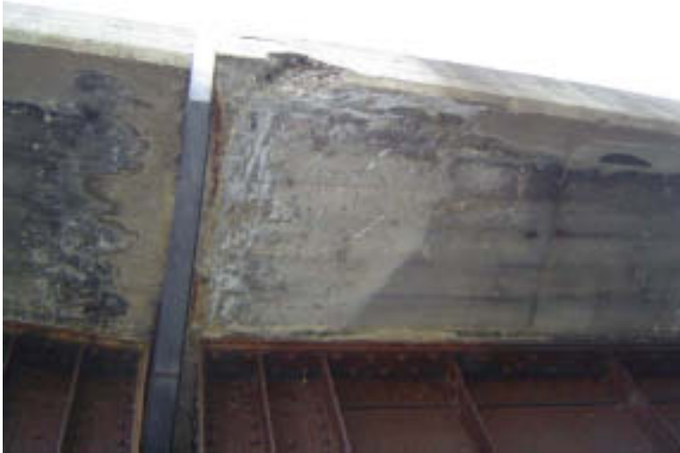
Span 7: Joint near Pier 7
