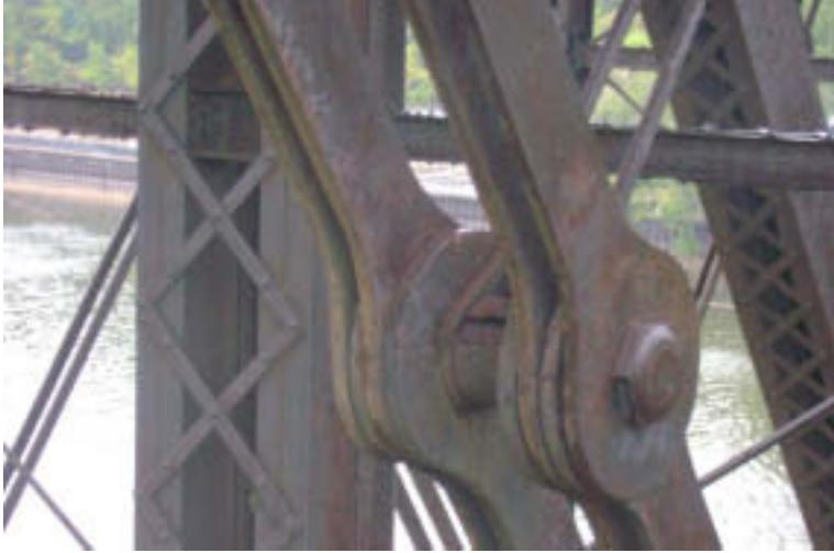
Span 4: Outside Truss Bracing
