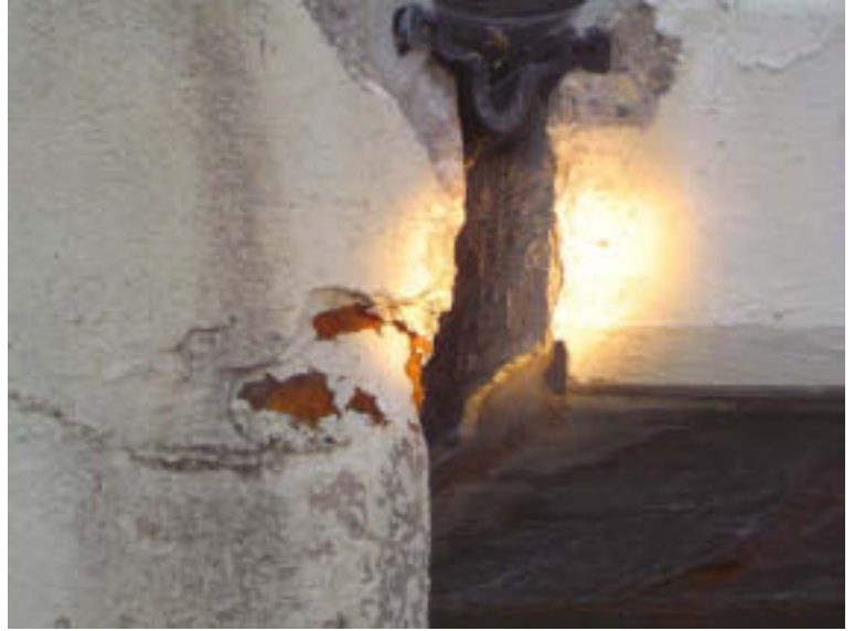
Span 2: Expansion Joint
