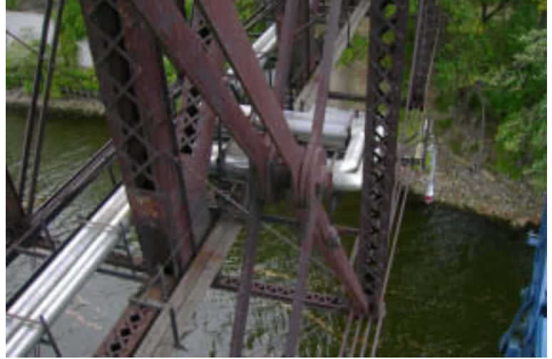
Span 3: Lower Chords
