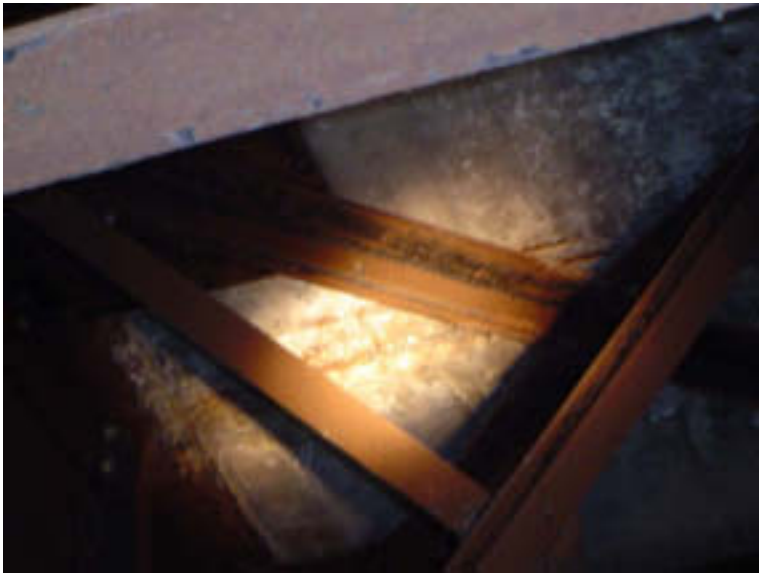
Span 7: Expose Reinforcement
