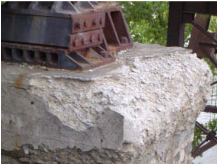
Pier 2: Pier Cap
