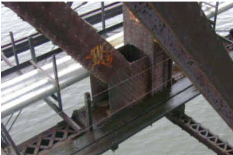
Span 3: Center Truss L1
