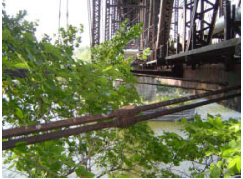
Span 3: Transverse Bracing
