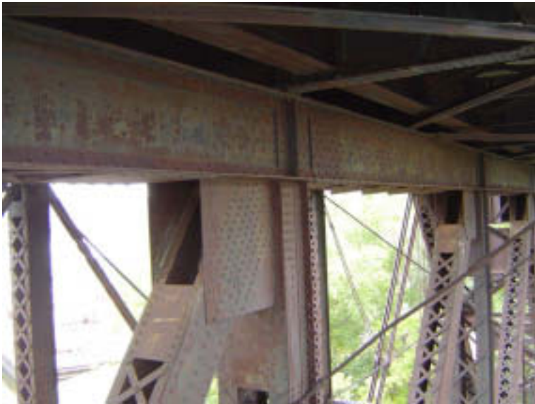
Span 4: Center Truss Upper Connection
