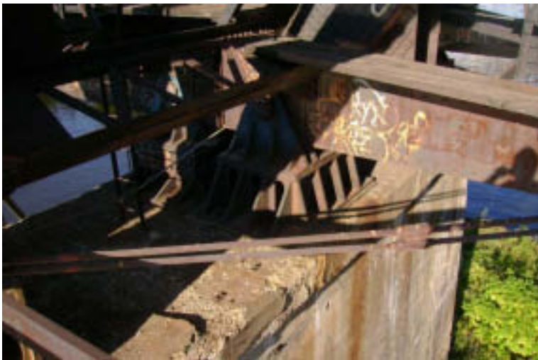
Pier 4: Center Bearing
