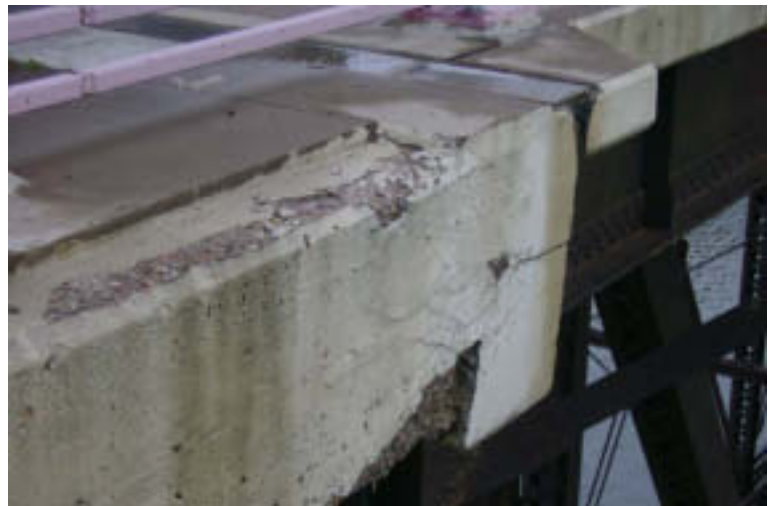
Span 5: Deck at Expansion Joint
