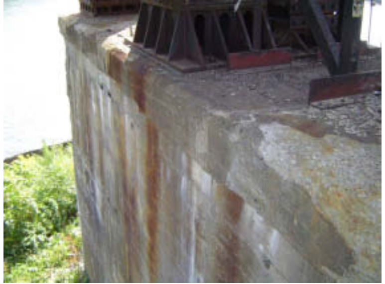
Pier 4: Cap and Column Wall
