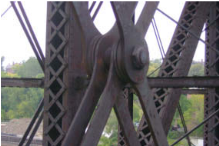
Span 4: Diagonal Members
