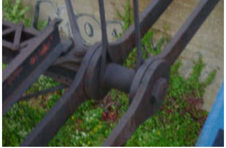
Span 4: Lower Chord Connection
