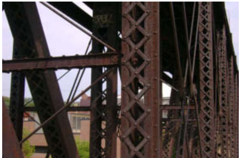
Span 3: Vertical Members
