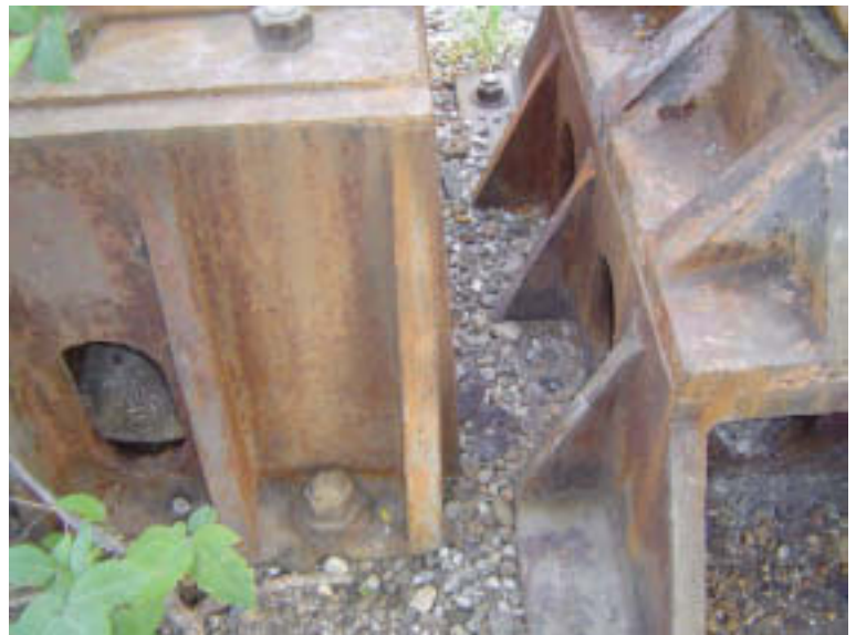
Pier 5: Concrete Cap and Bearing
