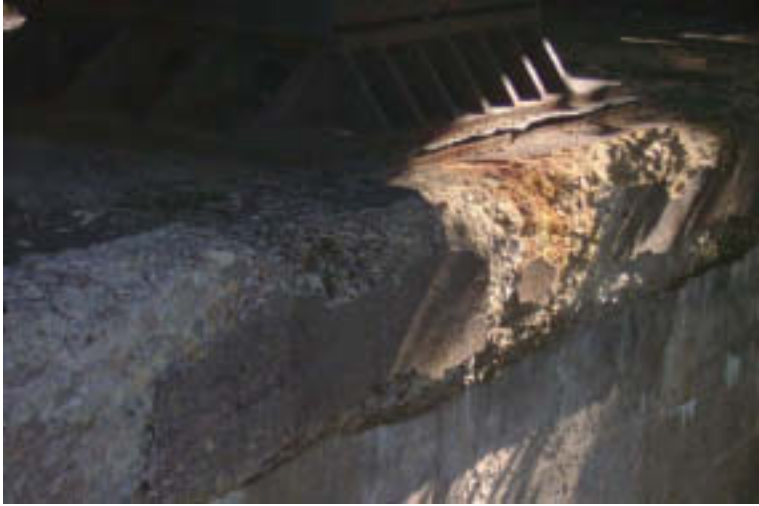
Pier 3: Concrete Cap
