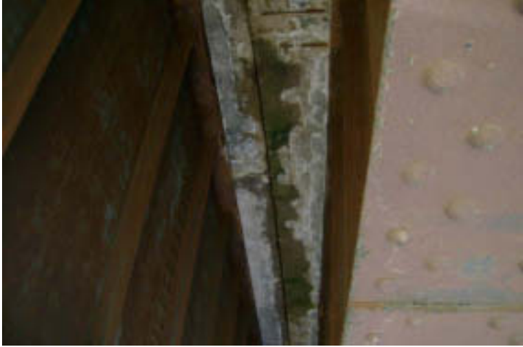
Span 5: Center Line of Deck
