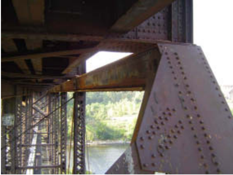
Span 3: Upper Chords
