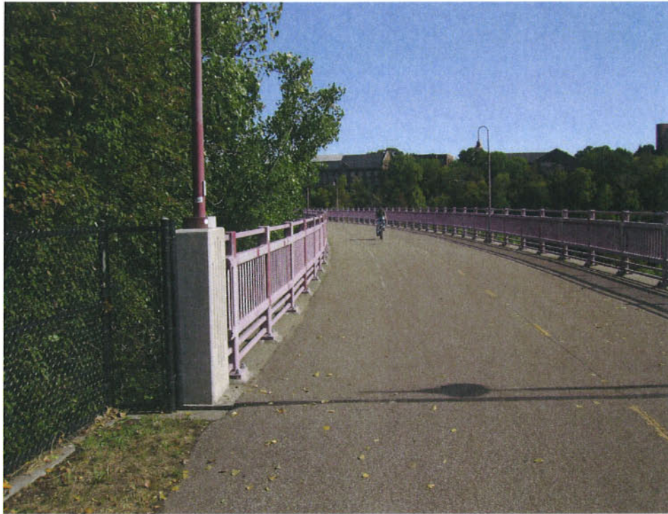
Looking East at West Abutment of Bridge No. 9
