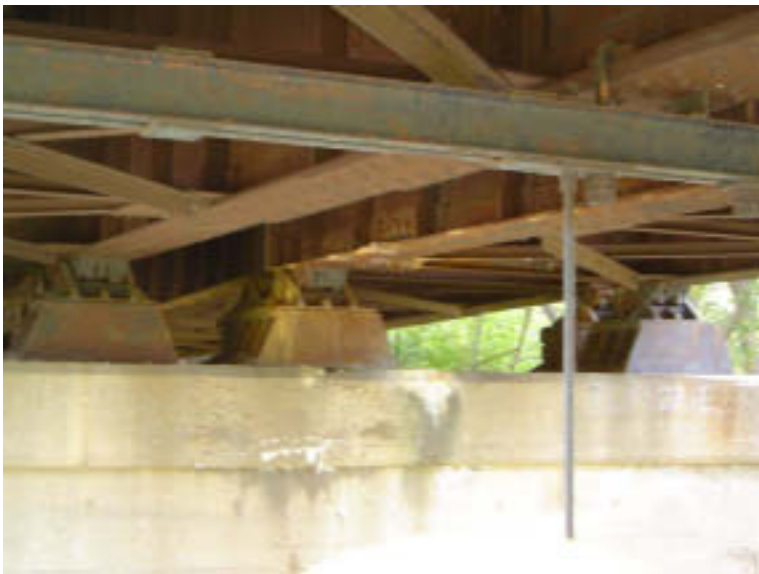
Pier 7: Pier Cap
