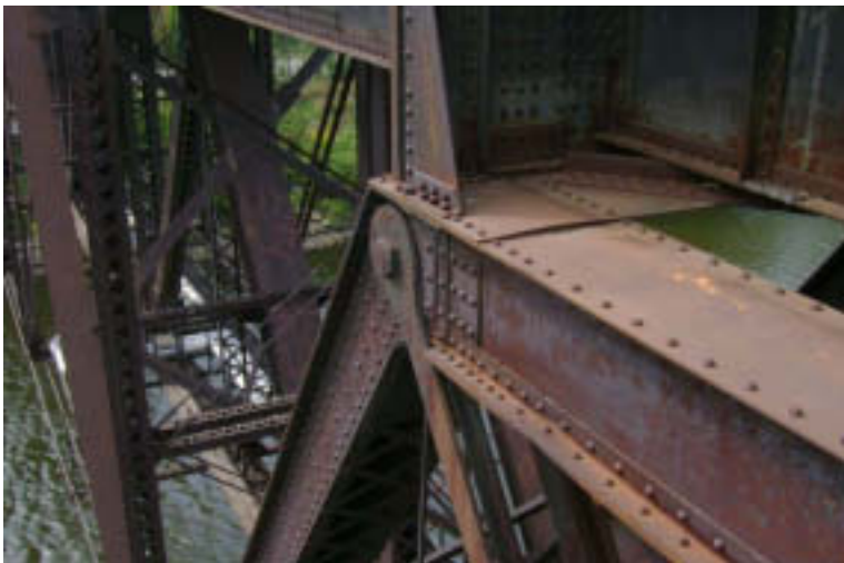
Span 3: Upper Chord and Floor Beam
