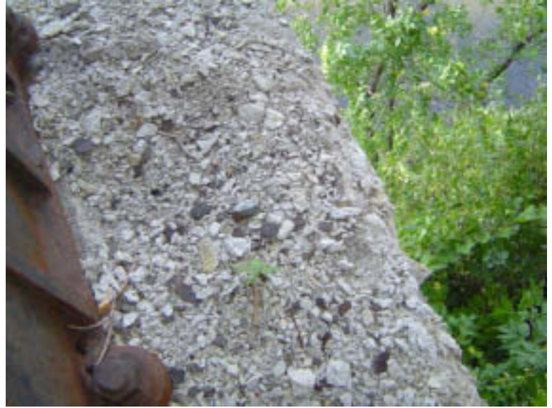
Pier 3: Lower Concrete Cap
