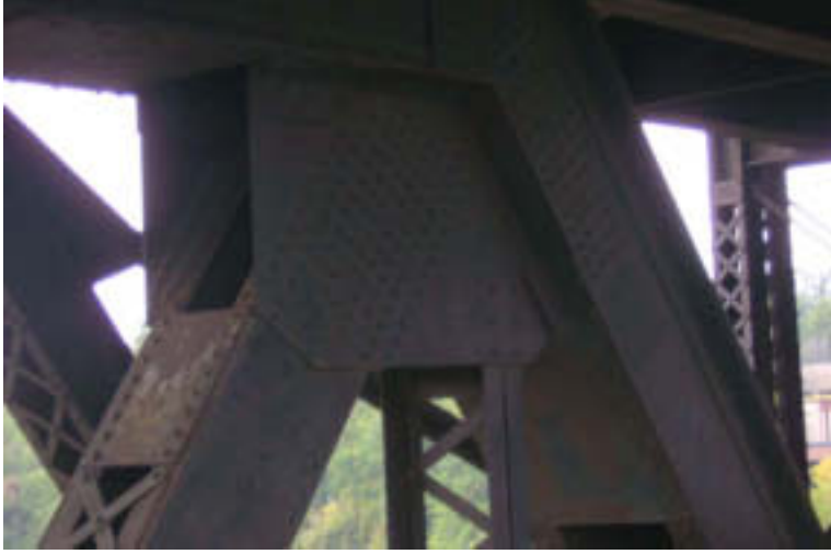
Span 4: Center Truss Connection
