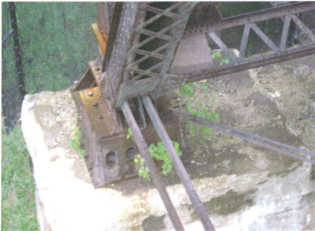
Truss Bearing of Bridge No. 9
