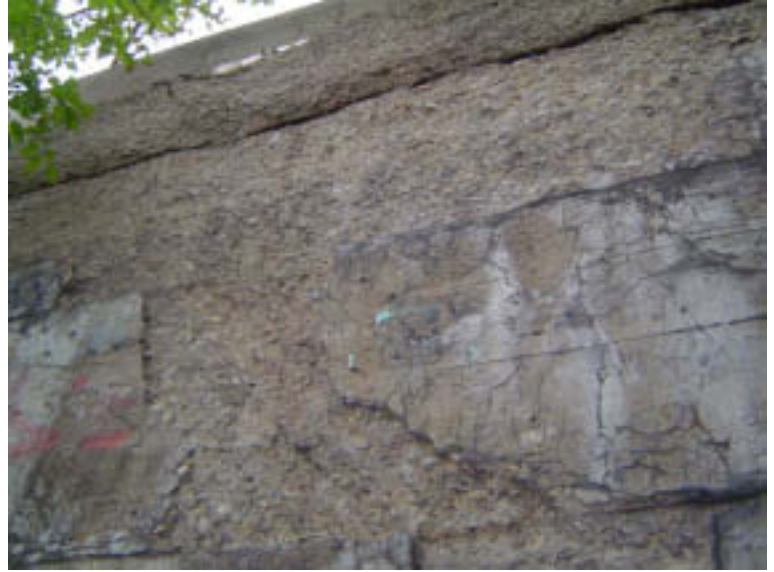
Abutment 1: North Wingwall
