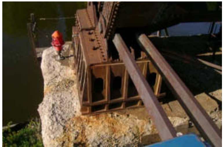
Pier 4: Side Bearing
