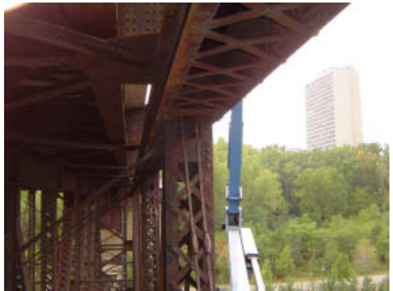
Span 4: Vertical Members
