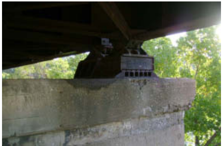
Pier 6: Pier Cap and Bearing
