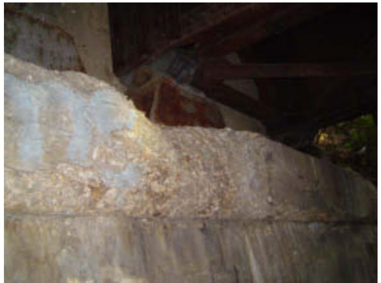
Abutment 1: Abutment Seat
