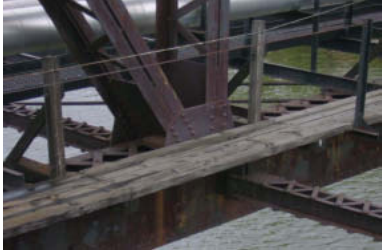
Span 3: Center Truss Lower Connection
