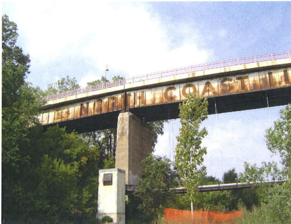
West Approach Spans of Bridge No. 9
