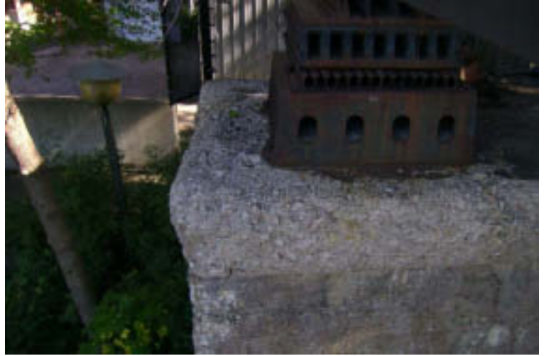
Pier 3: Concrete Cap and Bearing
