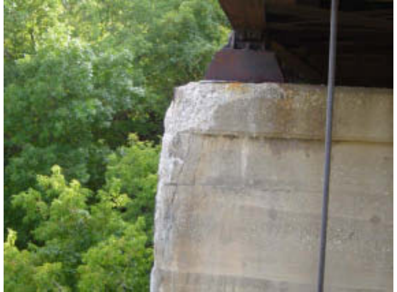
Pier 7: Pier Cap
