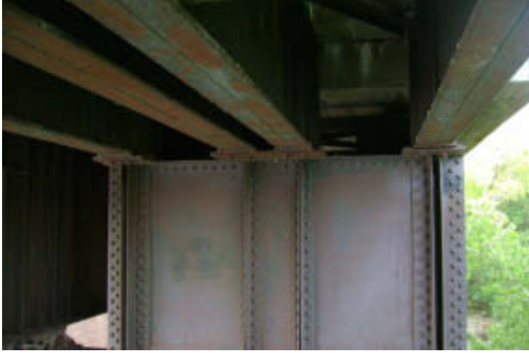
Pier 3: Upper Steel Cap
