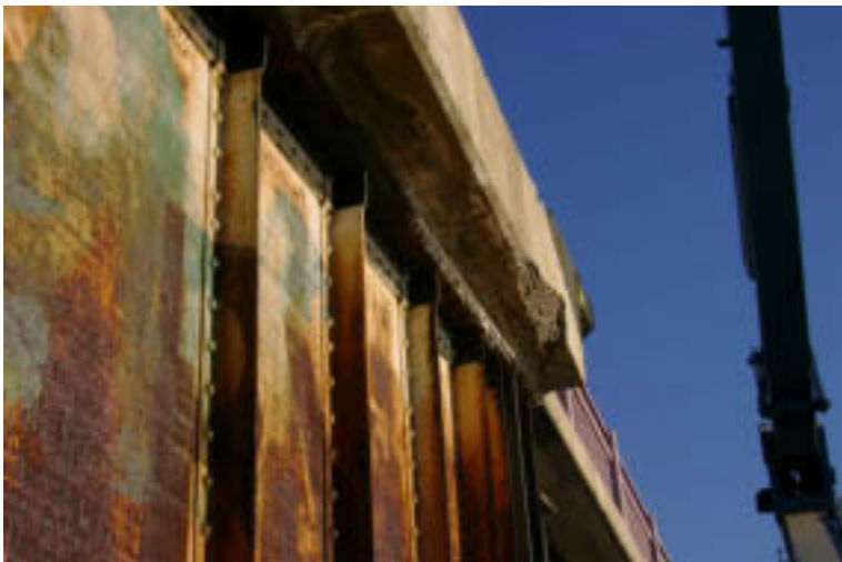
Span 5: Deck and Girder at the Expansion
