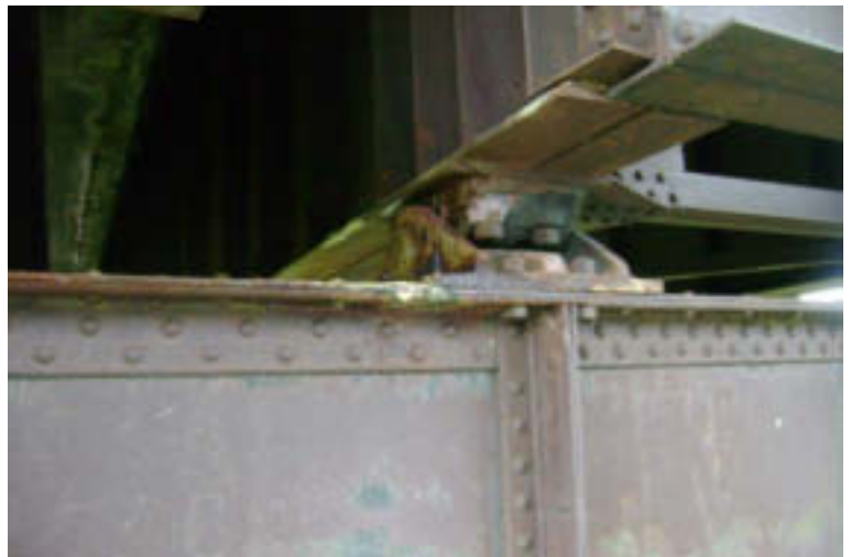
Pier 5: Steel Cap Bearing
