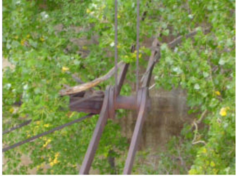
Span 3: Lower Chords
