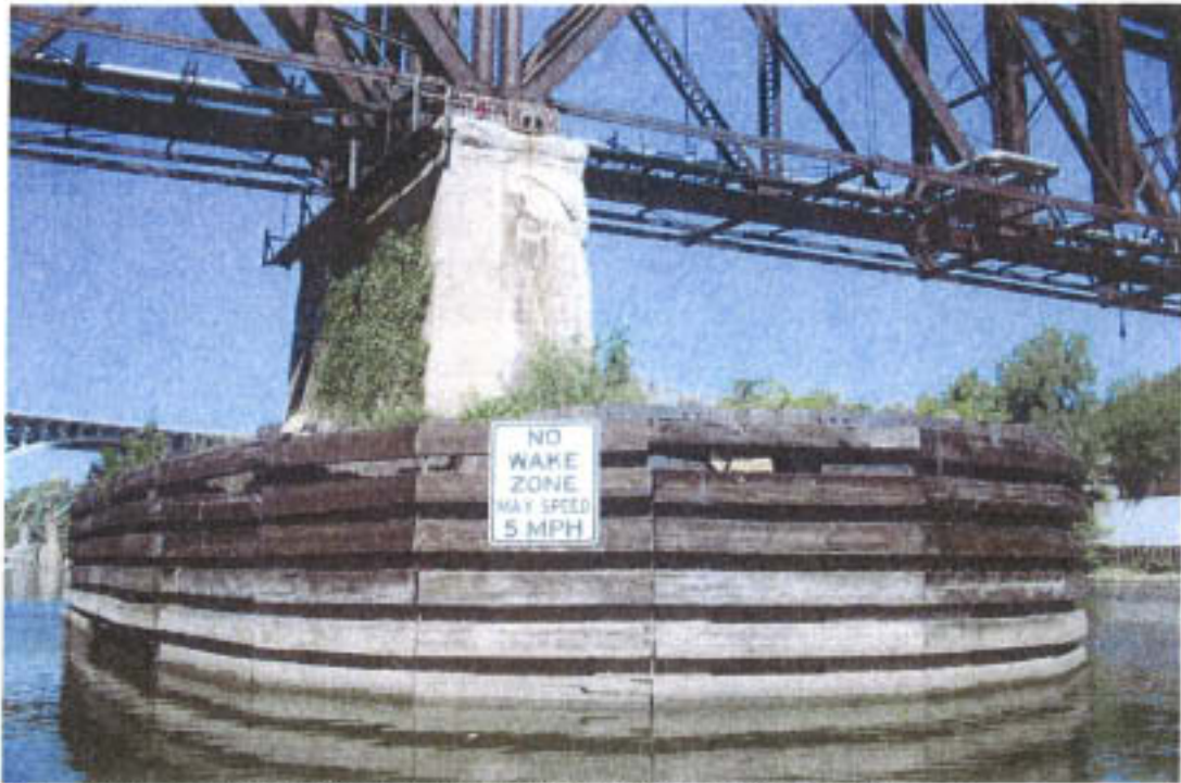
Photograph 1. View of Downstream End of Pier 4, Looking North.
