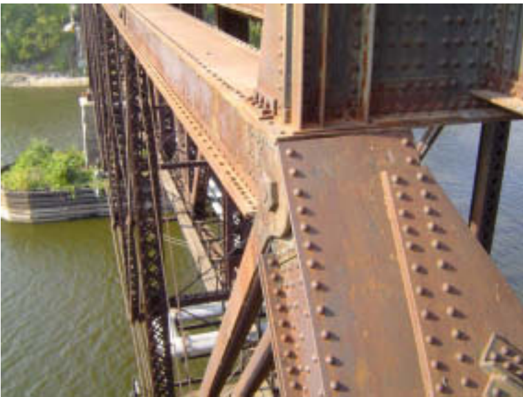
Span 3: Upper Truss Connections
