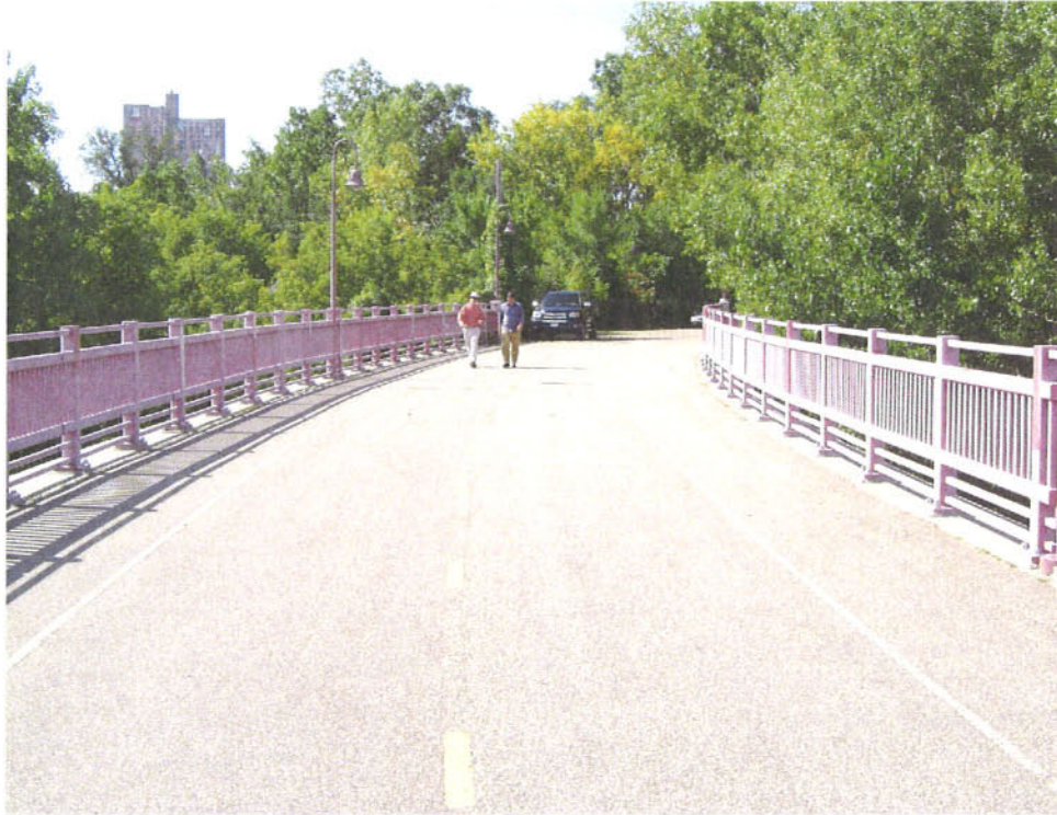
Looking West Towards West Abutment of Bridge No. 9
