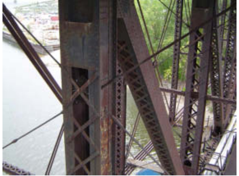
Span 4: Center Truss
