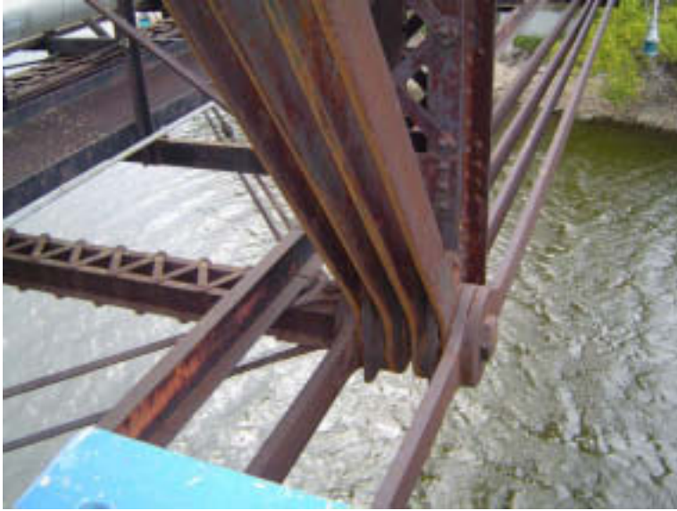
Span 4: Lower Chord Connection
