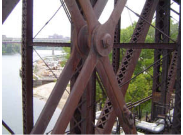
Span 3: Outside Truss Bracing
