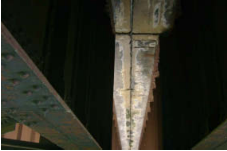
Span 1: Center of Deck
