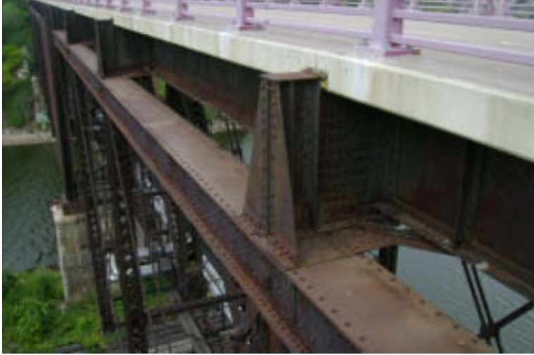
Span 3: Upper Chords
