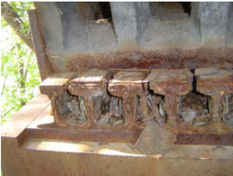
Pier 3: Lower Concrete Bearing
