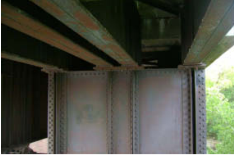
Pier 3: Upper Steel Cap
