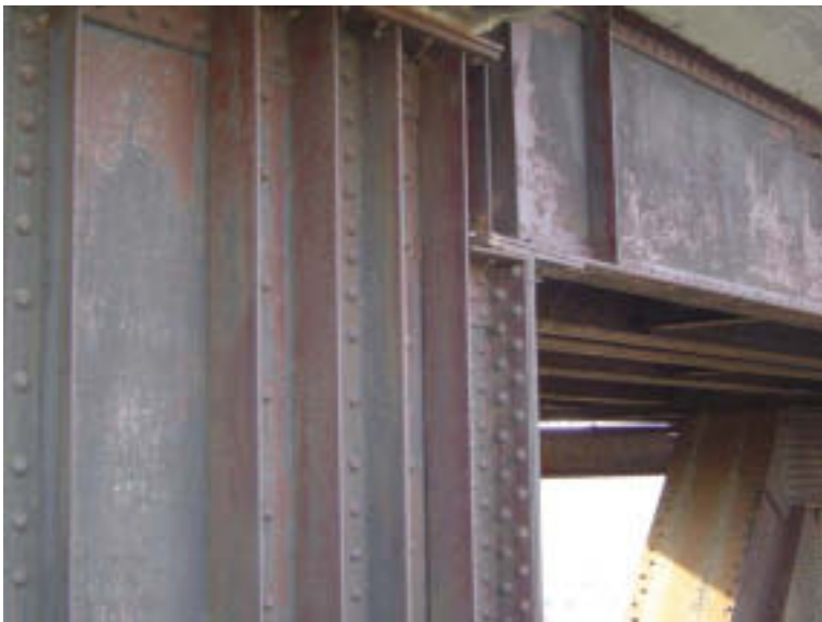
Pier 3: Steel Cap and Girder Span Bearing
