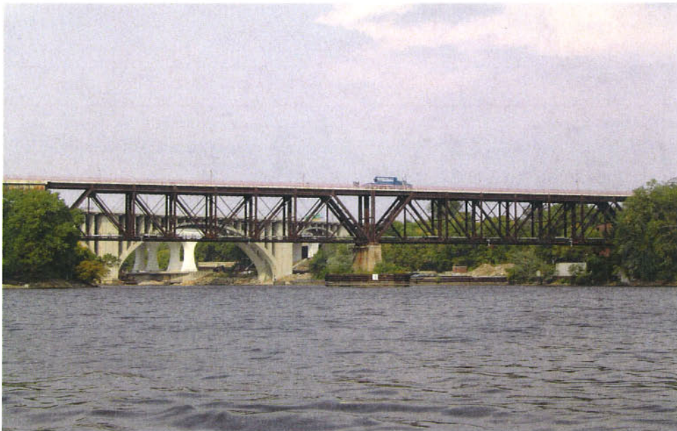
Looking North Towards Bridge No. 9
