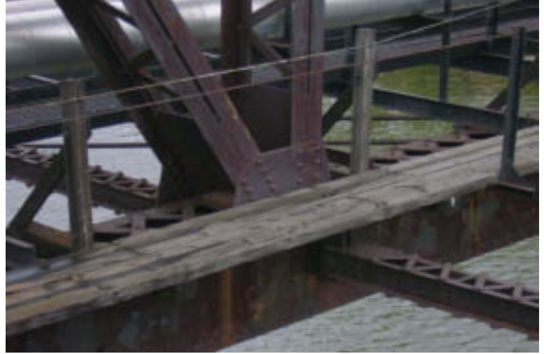
Span 3: Center Truss Lower Connection
