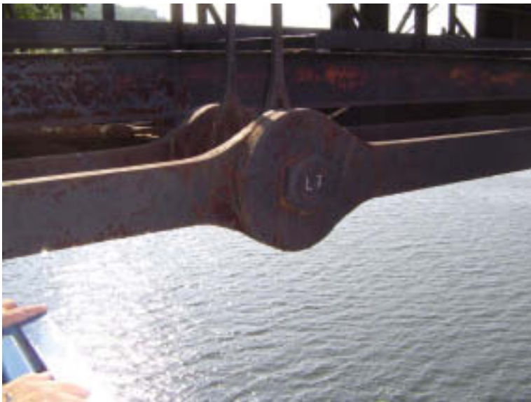
Span 3: Bottom Chords
