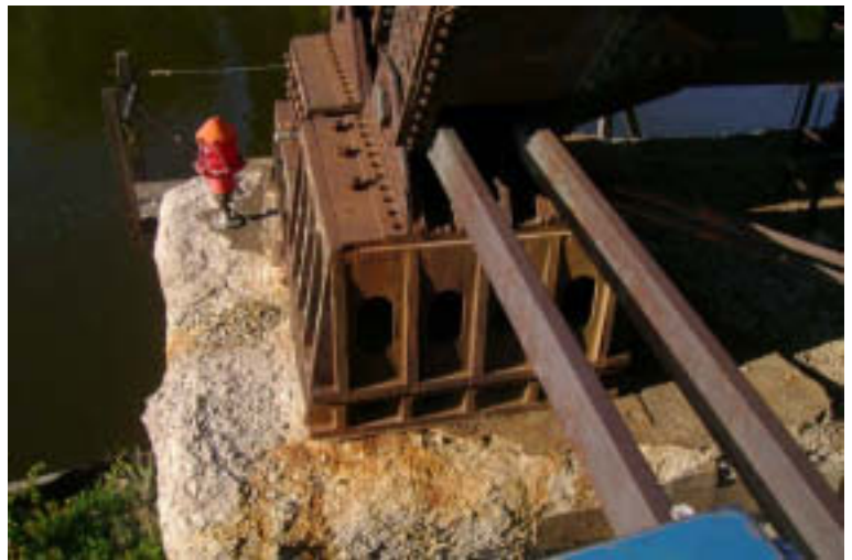
Pier 4: Side Bearing
