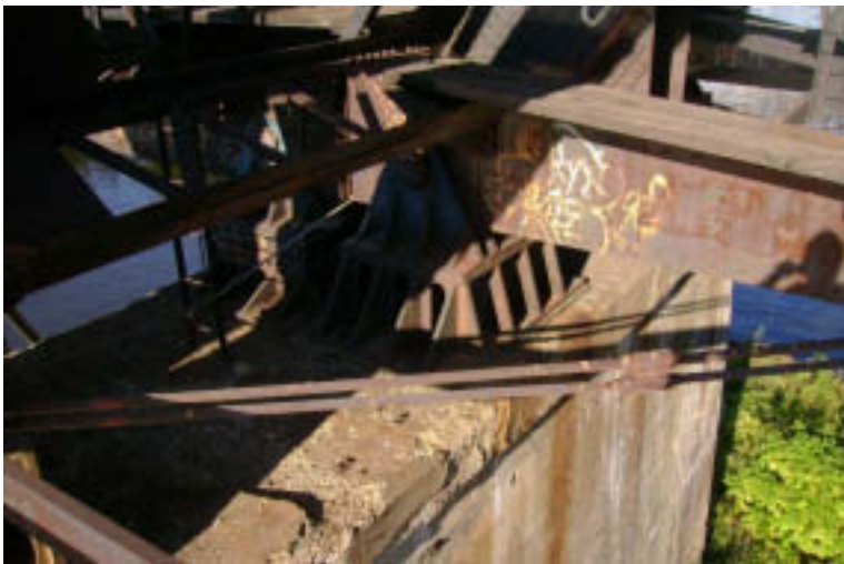
Pier 4: Center Bearing
