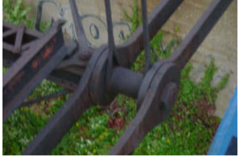
Span 4: Lower Chord Connection
