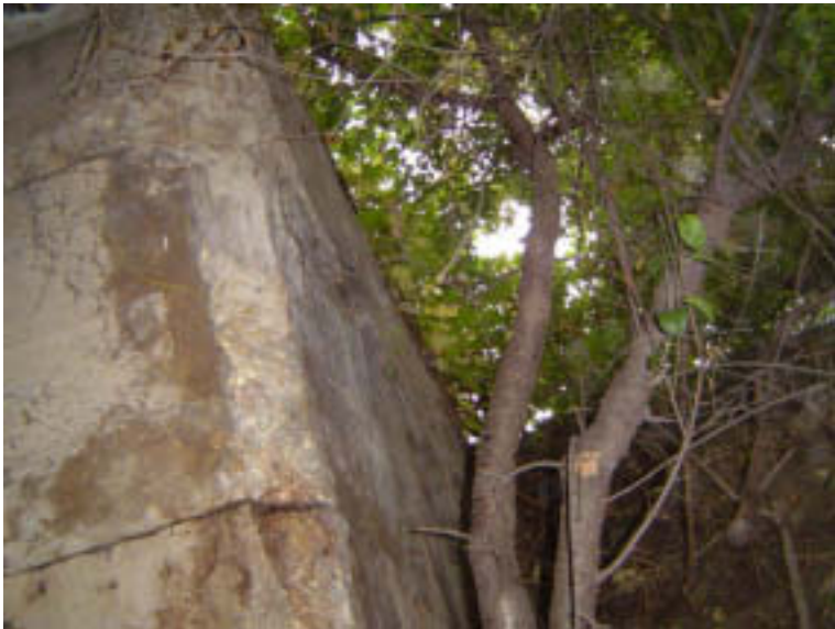
Abutment 1: South Wingwall
