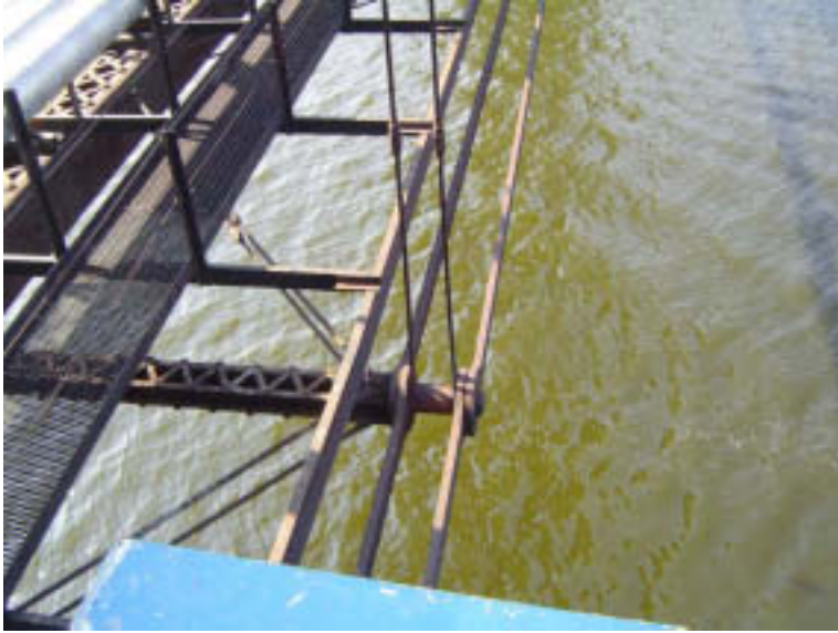
Span 3: Bottom Chords
