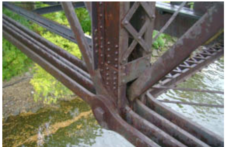
Span 3: Outside Truss L1
