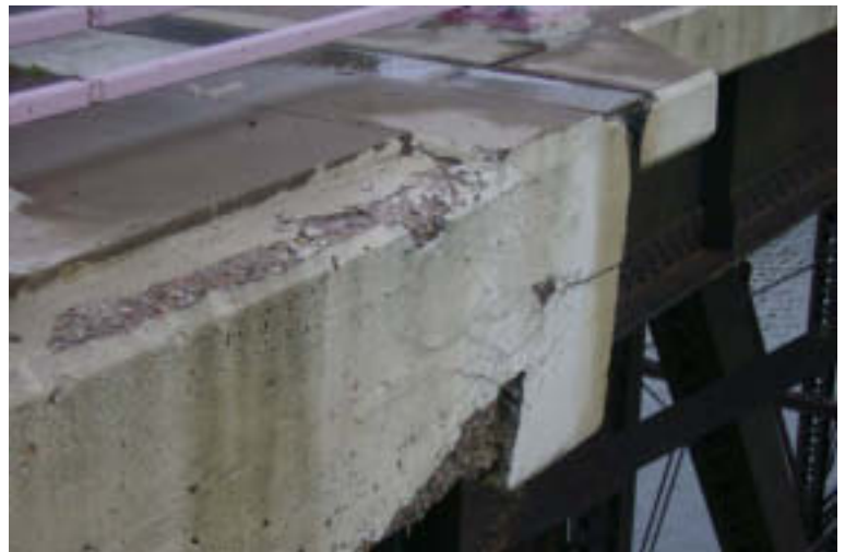
Span 5: Deck at Expansion Joint
