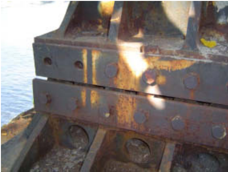
Pier 3: Lower Concrete Bearing
