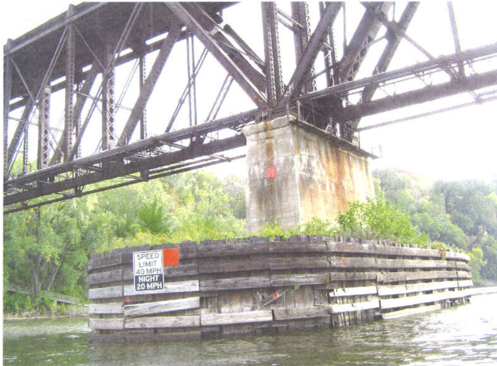
Looking Towards River Pier Fender of Bridge No. 9
