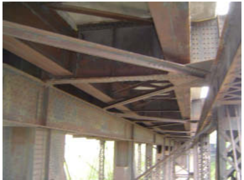
Span 4: Center Truss: Floor Beams and Stringers
