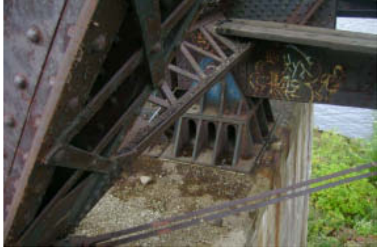
Pier 4: Center Bearing
