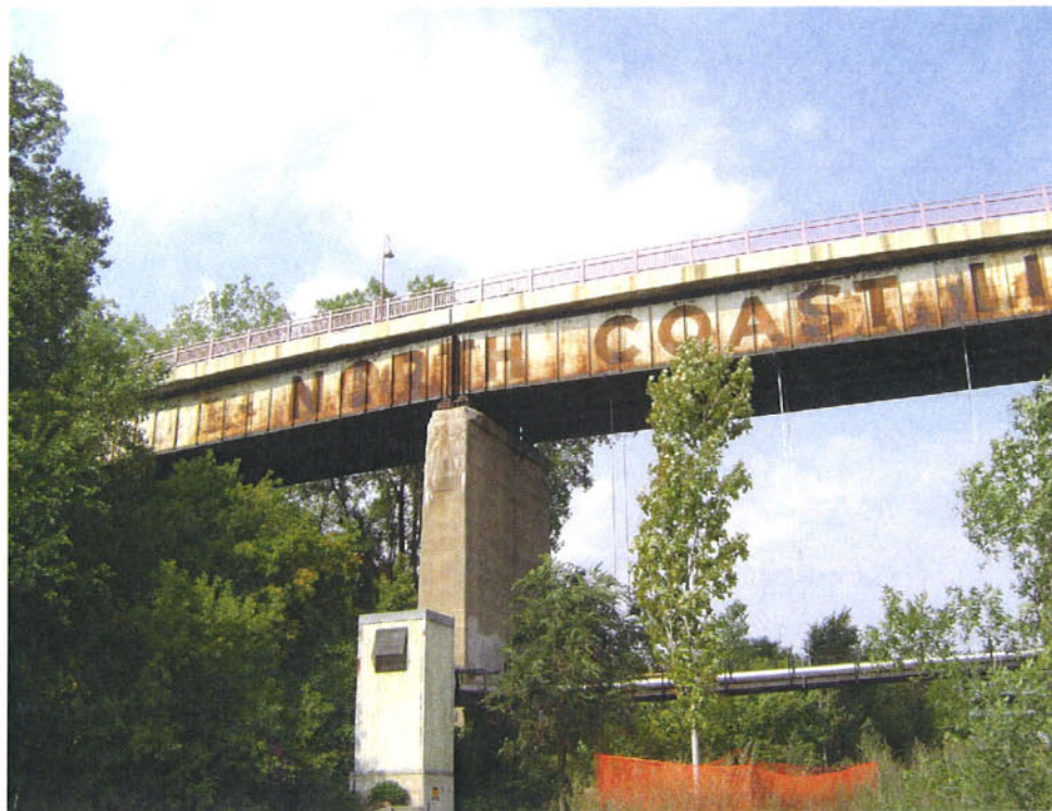
West Approach Spans of Bridge No. 9
