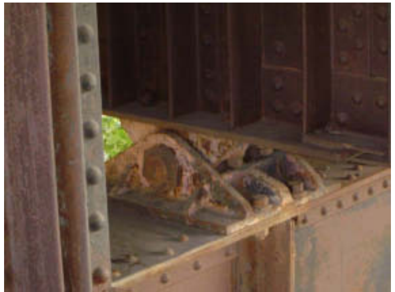
Pier 3: Steel Cap and Girder Span Bearing
