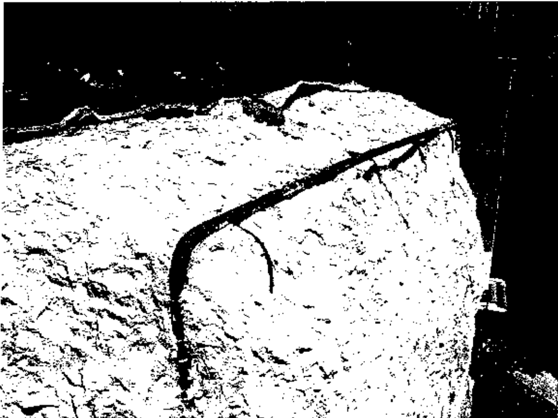
Exposed Rebar and Spalled Concrete at End of Cap
