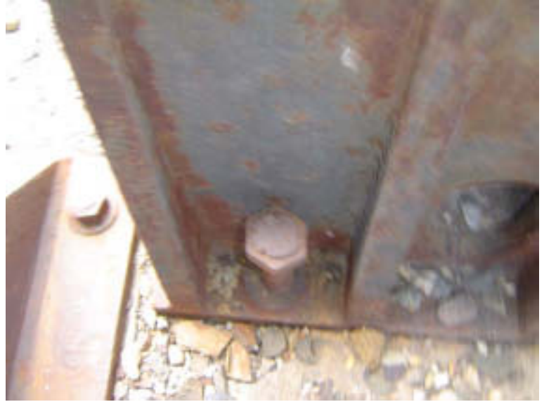
Pier 5: Concrete Cap
