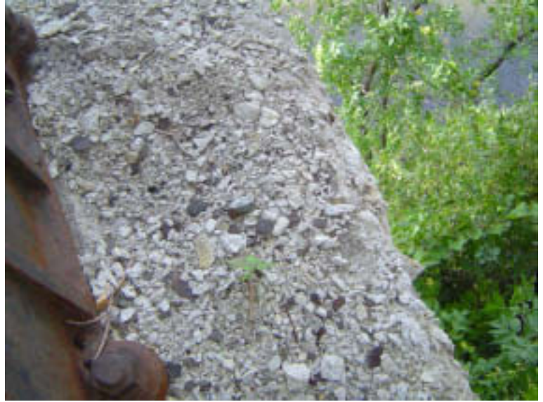
Pier 3: Lower Concrete Cap
