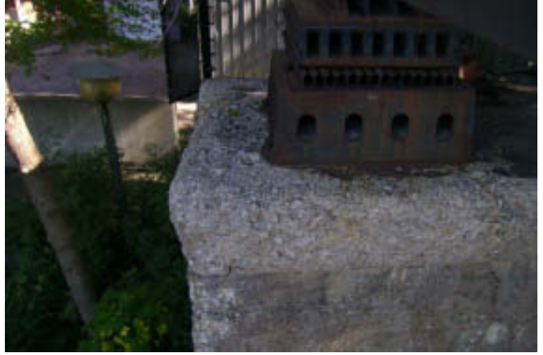
Pier 3: Concrete Cap and Bearing
