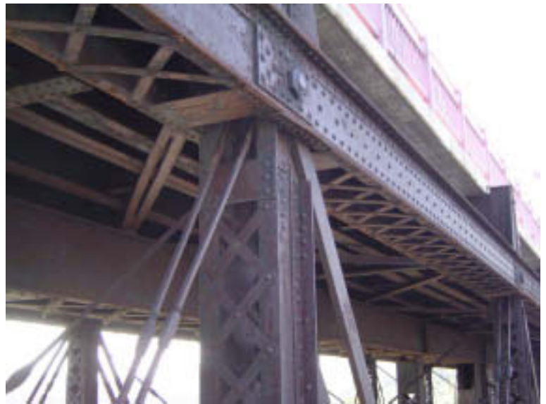
Span 3: Top Chords and Vertical Members
