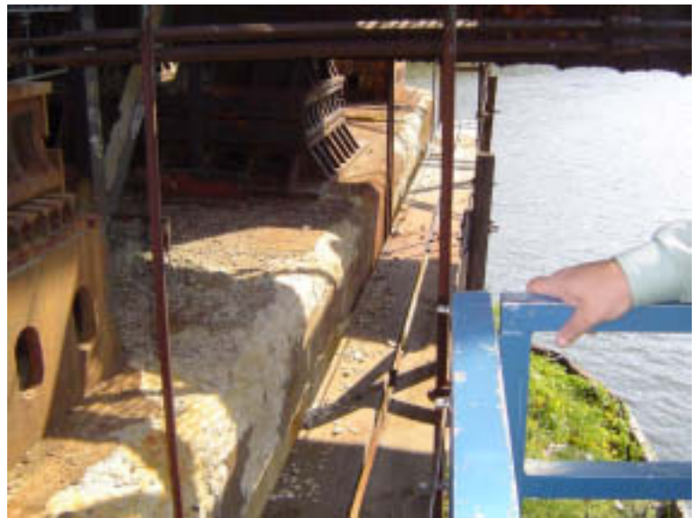
Pier 4: Pier Cap
