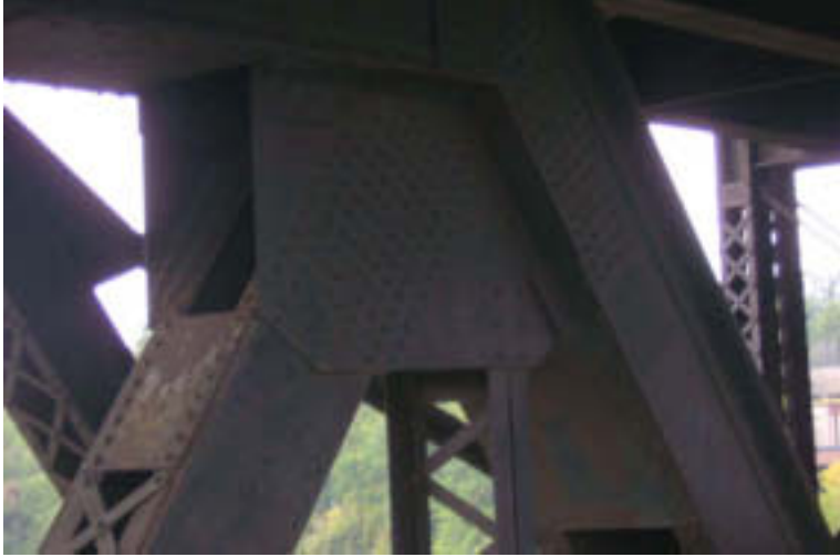
Span 4: Center Truss Connection
