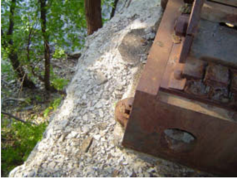
Pier 3: Lower Concrete Cap
