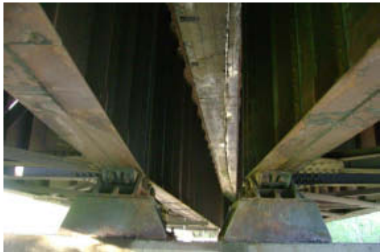
Span 6: Center Line of Deck
