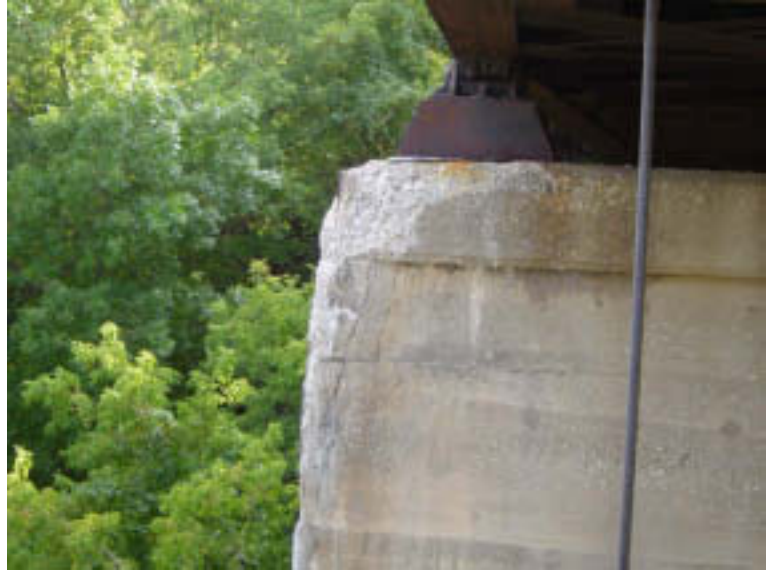
Pier 7: Pier Cap
