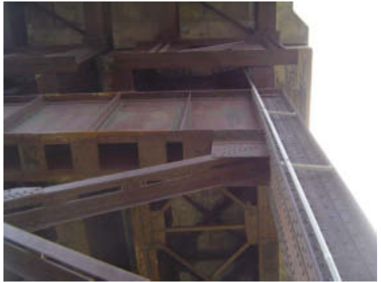
Pier 5: Steel Column
