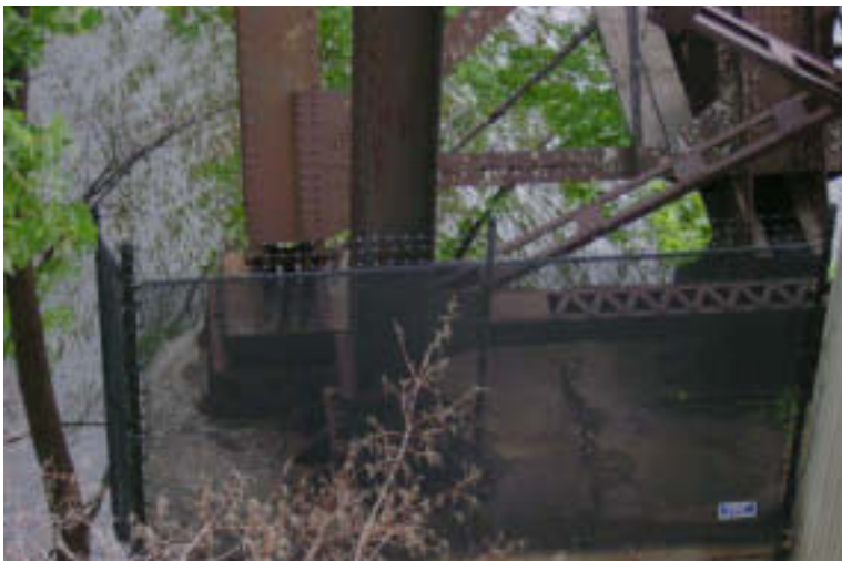
Pier 3: Lower Concrete Cap
