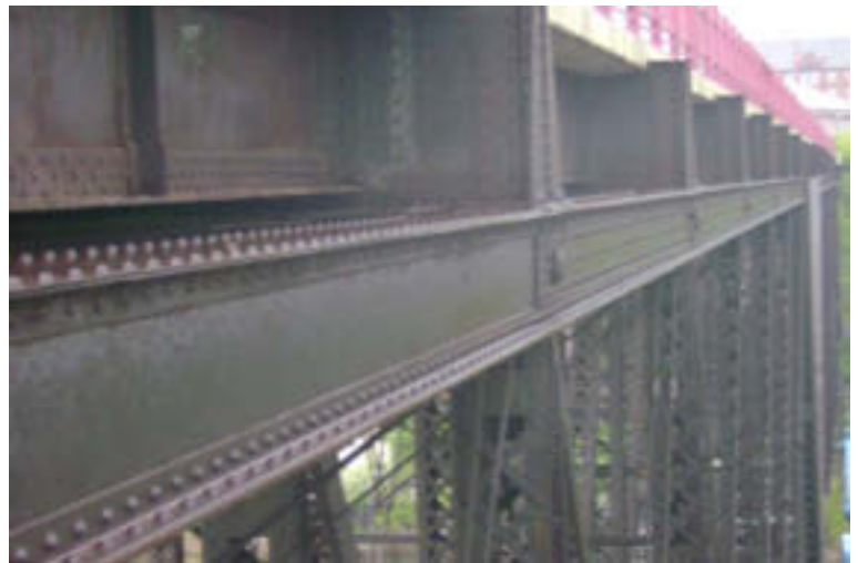
Span 4: Upper Chords: Floor Beams and Stringers
