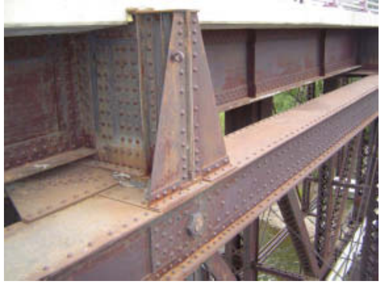
Span 4: Upper Chord: Floor Beams and Stringers
