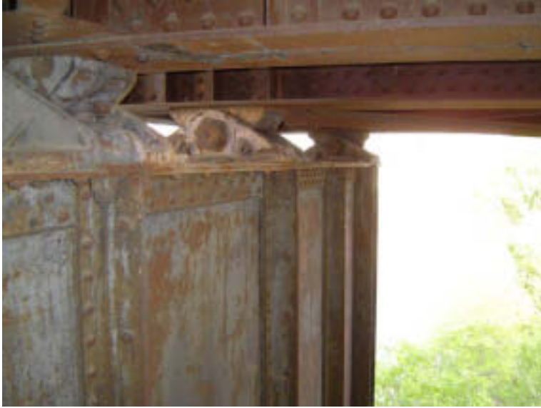
Pier 3: Steel Cap and Girder Span Bearing
