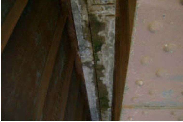
Span 5: Center Line of Deck
