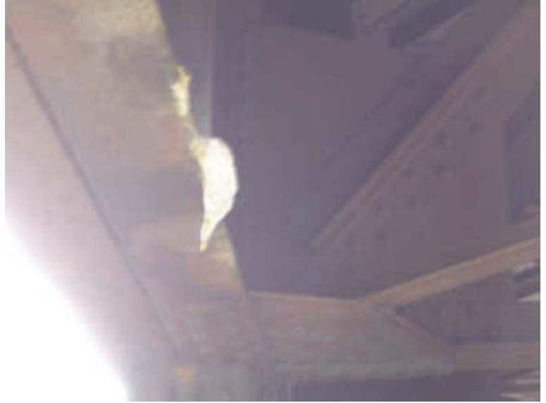
Span 5: Calcium Carbonate Built
