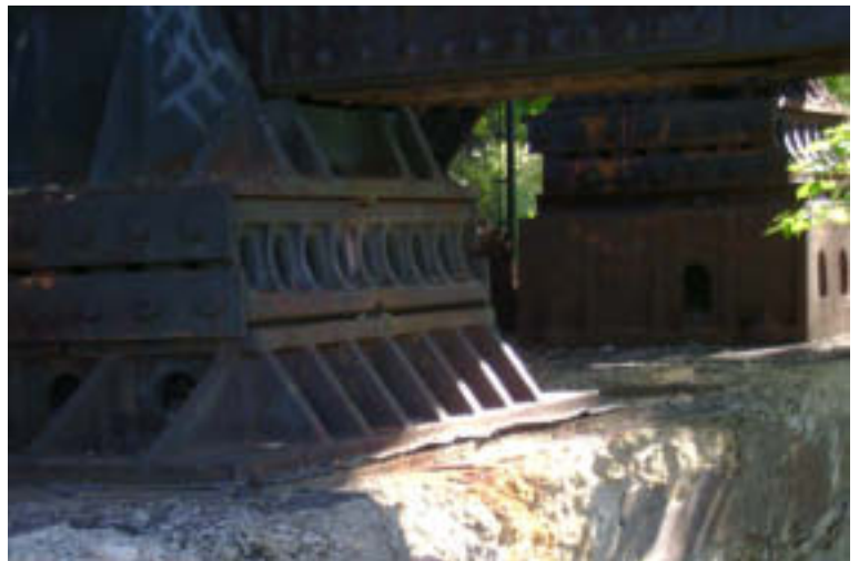
Pier 3: Bearing and Concrete Cap
