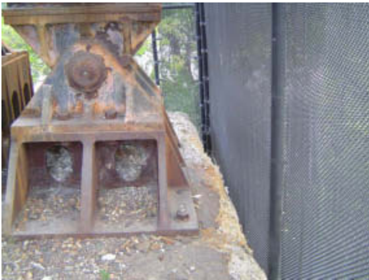
Pier 5: Concrete Cap
