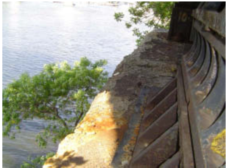
Pier 3: Lower Concrete Cap
