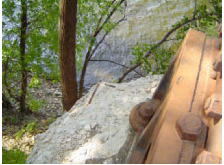
Pier 3: Lower Concrete Cap
