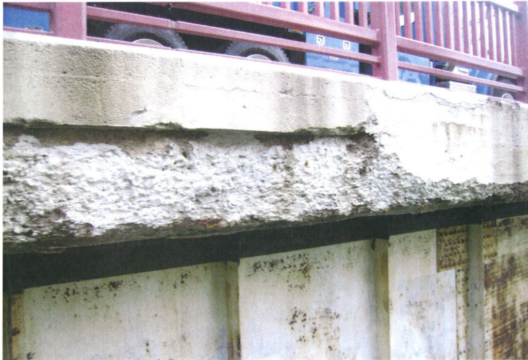
Looking Towards South Deck Edge in End Span of Bridge No. 9
