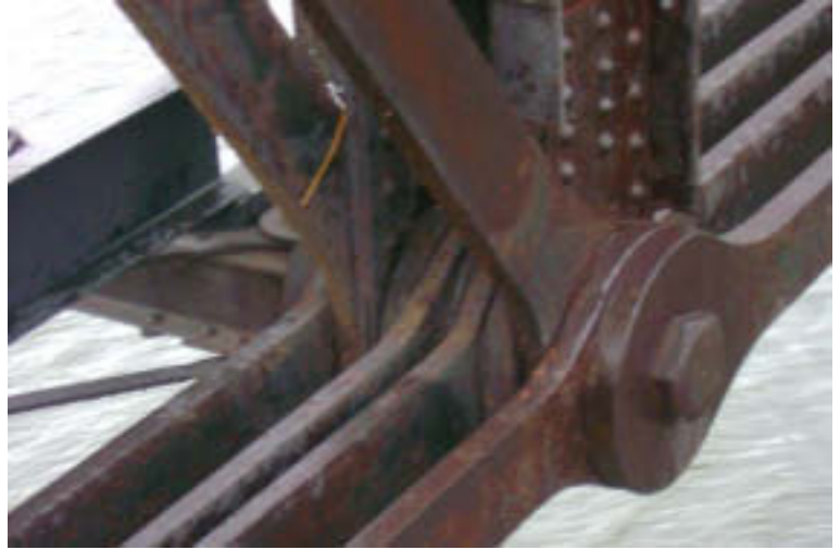
Span 4: Lower Chord Connection
