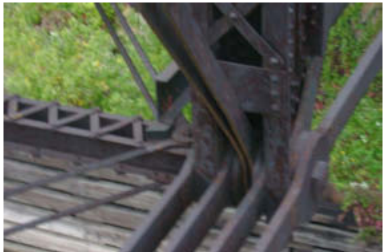
Span 4: Lower Chord Connection
