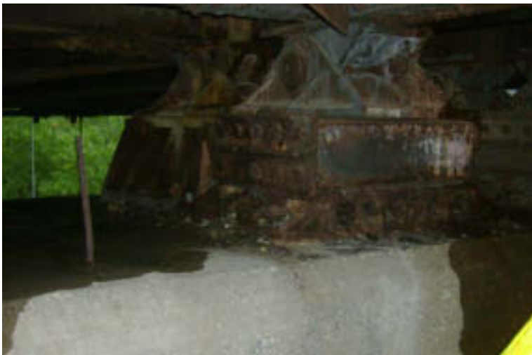
Pier 7: Drainage on Cap from Deck
