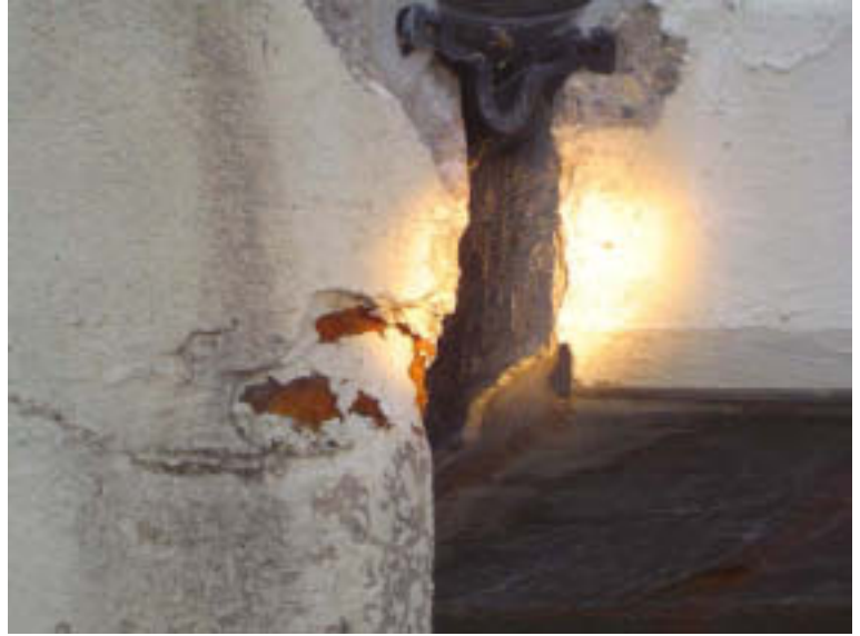
Span 2: Expansion Joint
