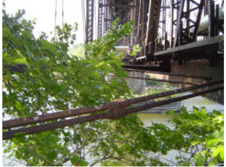
Span 3: Transverse Bracing
