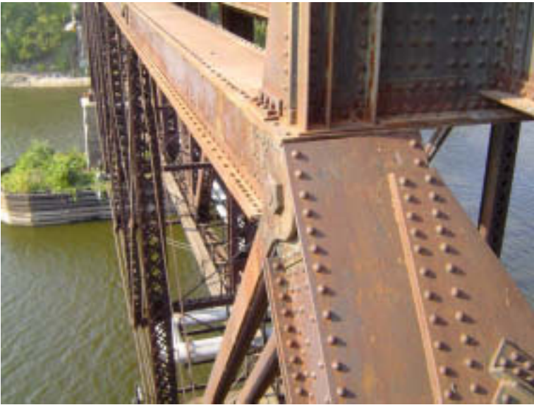
Span 3: Upper Truss Connections
