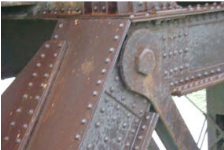
Span 4: Upper Chord
