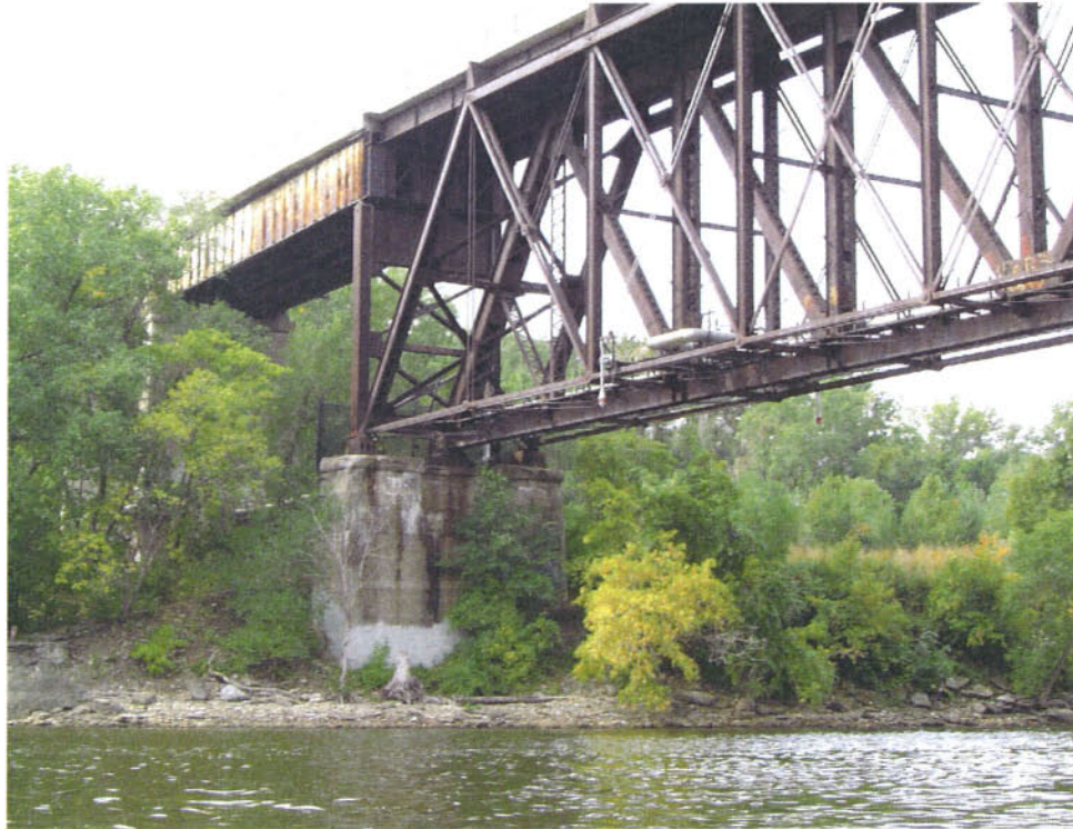
Looking Towards West Approach Spans of Bridge No. 9
