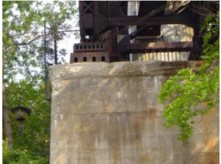
Pier 3: Concrete Pier
