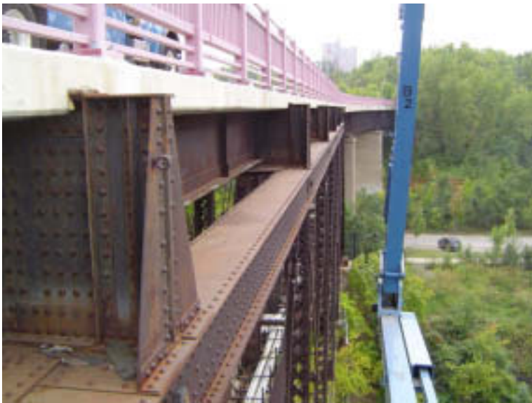
Span 4: Upper Chord: Floor Beams and Stringers
