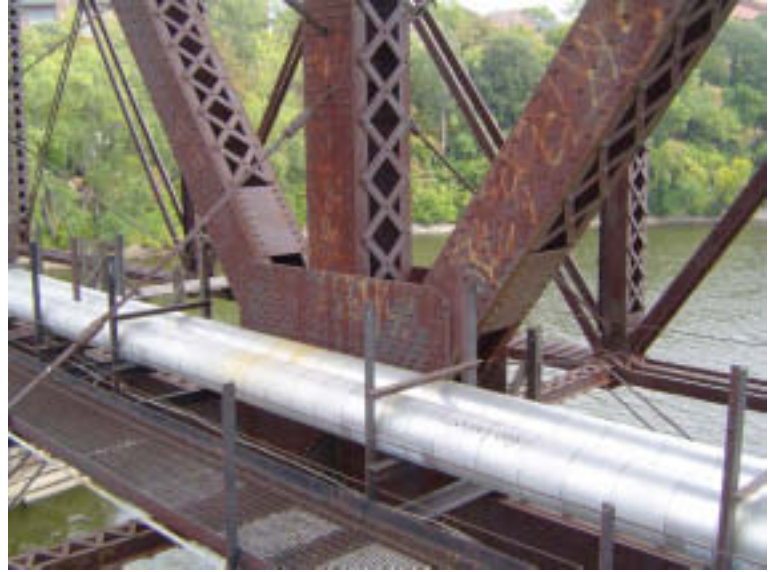
Span 4: Center Truss Lower Connection
