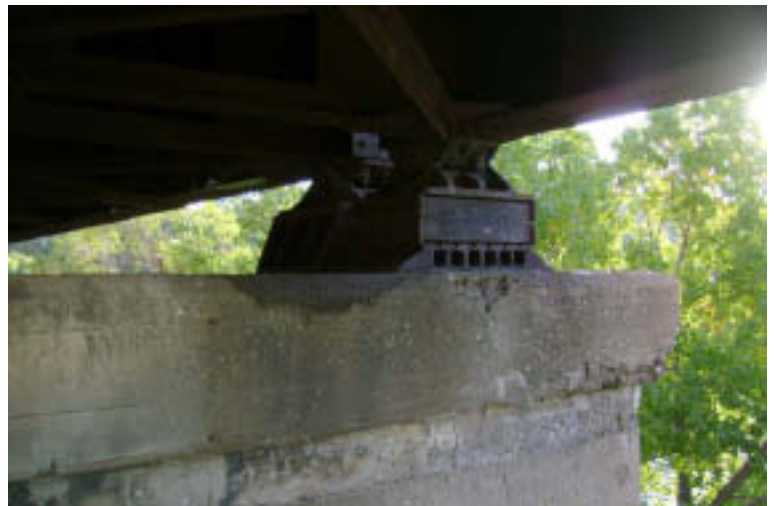
Pier 6: Pier Cap and Bearing
