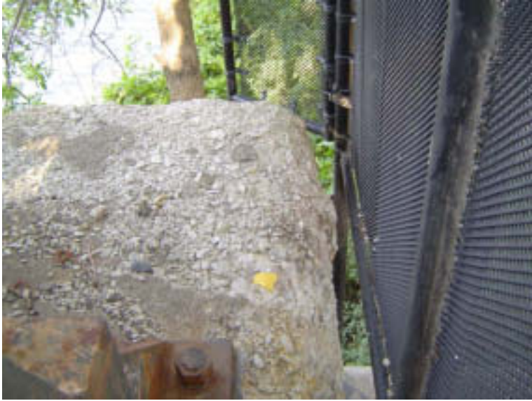
Pier 3: Lower Concrete Cap
