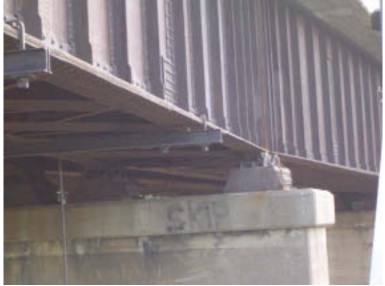
Pier 6: Pier Cap and Bearing
