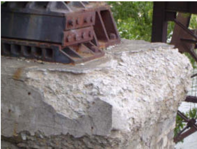
Pier 2: Pier Cap
