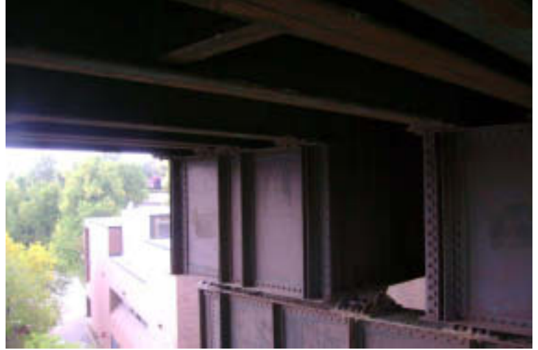
Pier 3: Upper Steel Cap
