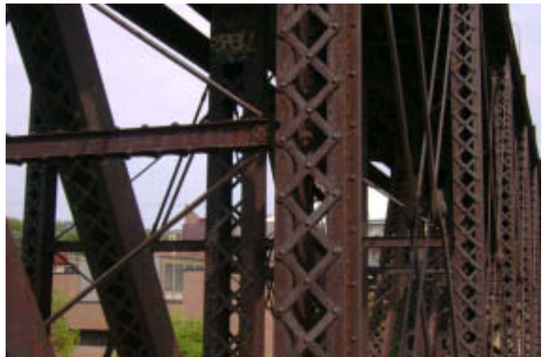
Span 3: Vertical Members
