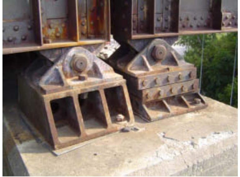
Pier 6: Pier Cap
