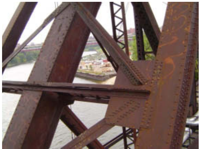
Span 4: Diagonal Members
