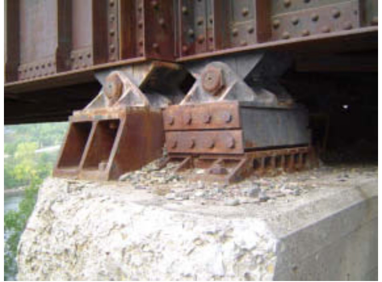
Pier 2: Pier Cap
