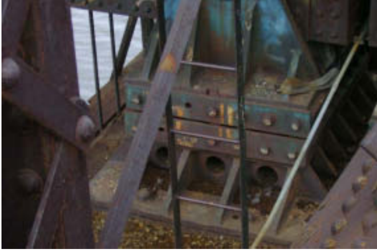
Pier 4: Center Bearing
