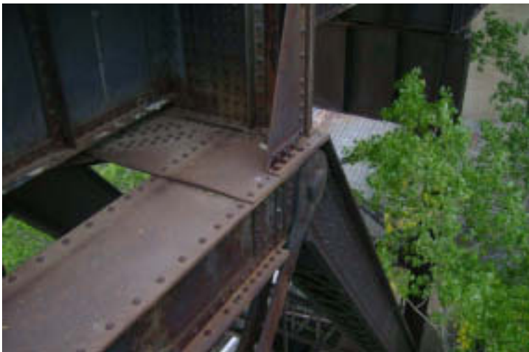
Span 3: Upper Chords Members
