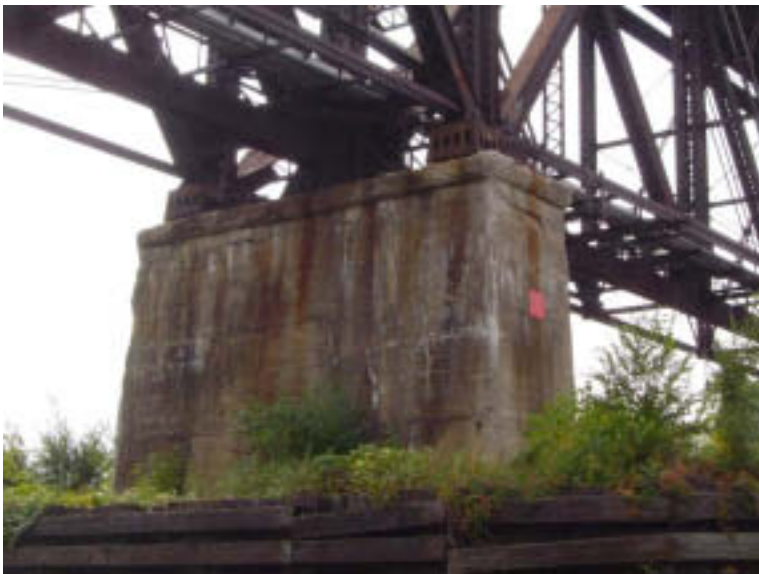
Pier 4: Side Bearing
