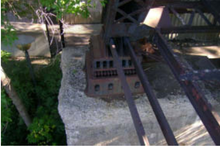
Pier 3: Concrete Cap and Bearing
