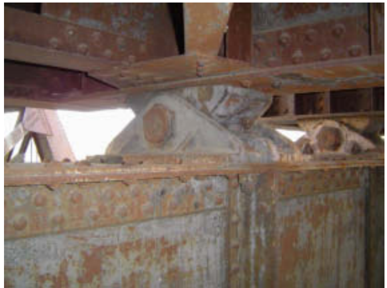
Pier 3: Steel Cap and Girder Span Bearing
