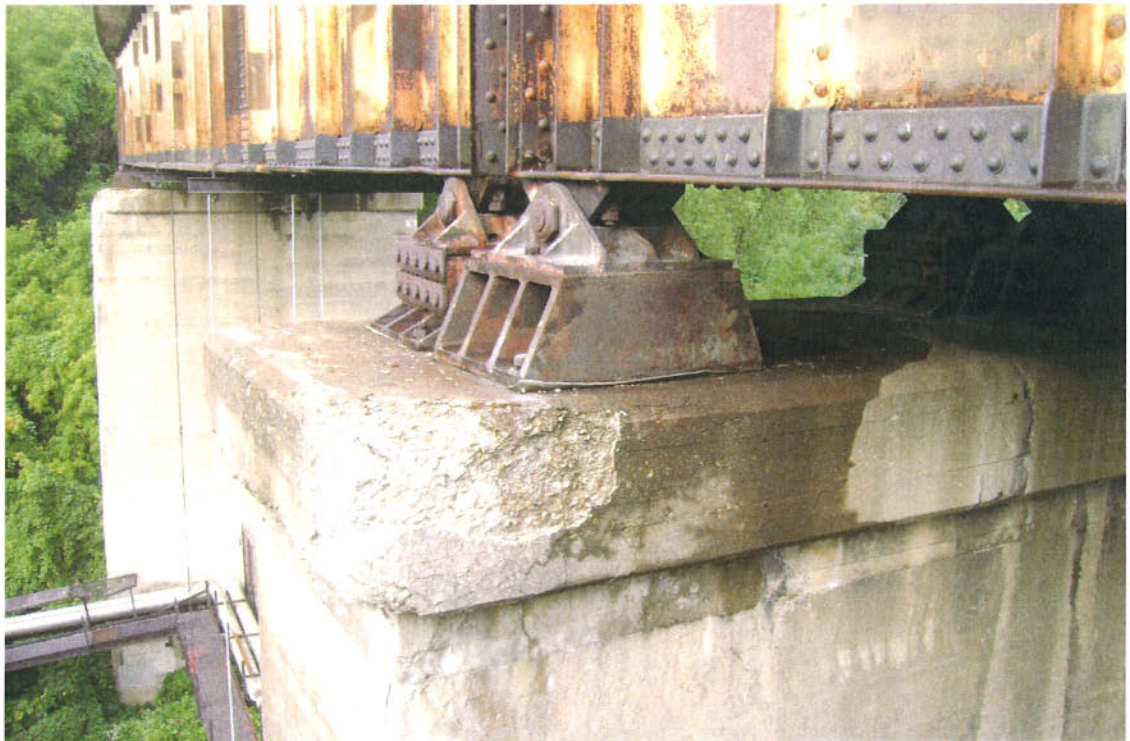
Looking Towards West Approach Bearings at Pier 6 of Bridge No. 9
