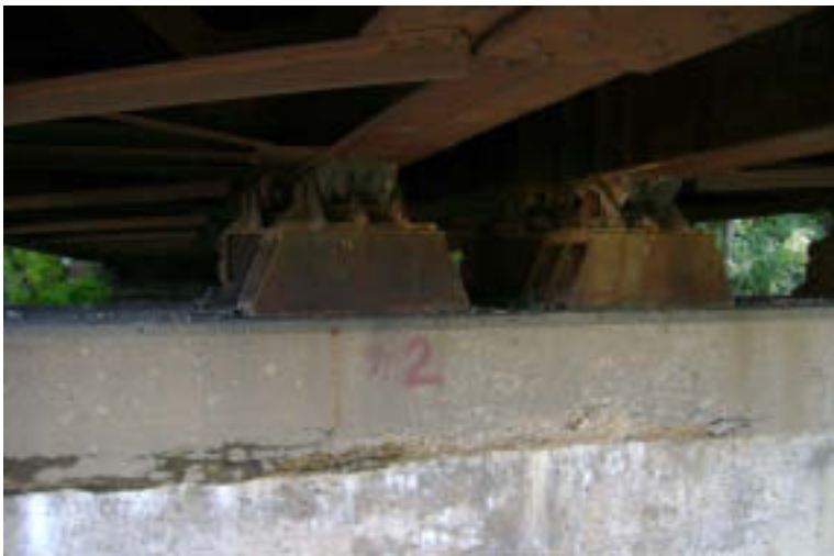
Pier 2: Pier Cap and Bearings
