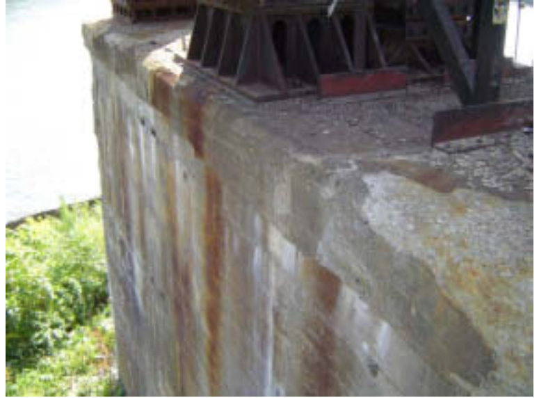
Pier 4: Cap and Column Wall
