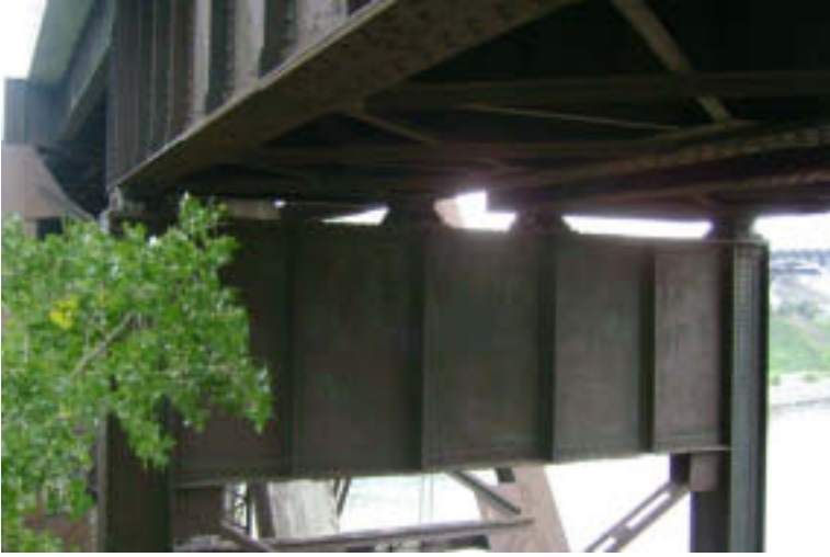
Pier 3: Steel Cap
