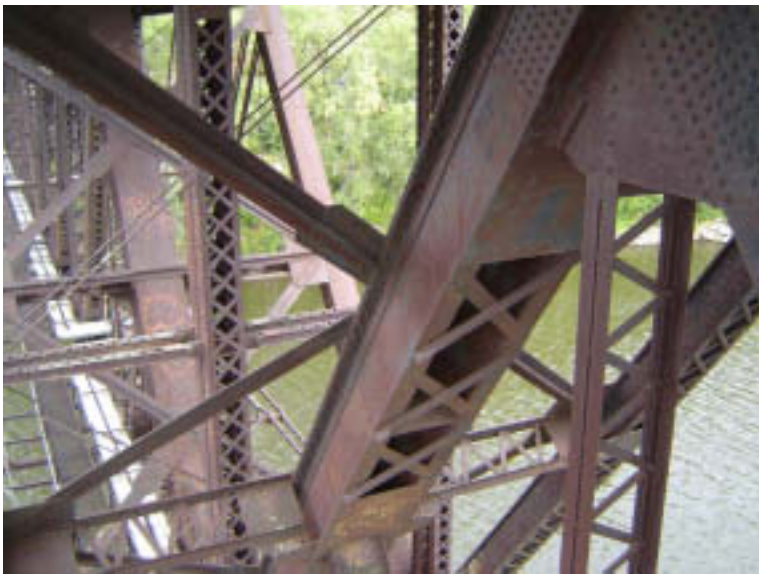
Span 4: Center Truss
