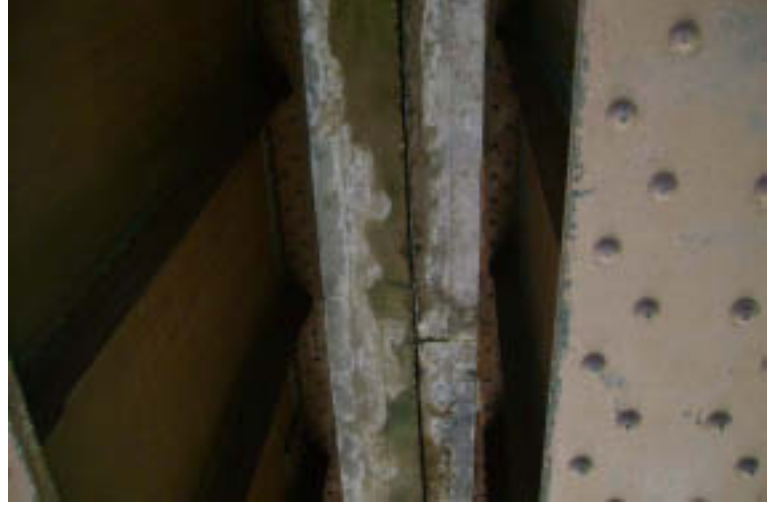
Span 5: Center Line of Deck
