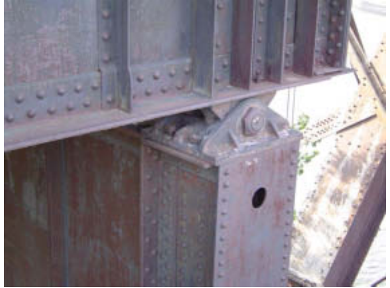
Pier 3: Steel Cap and Girder Span Bearing
