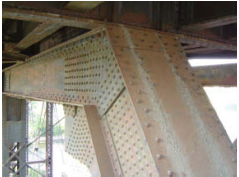
Span 3: Center Truss
