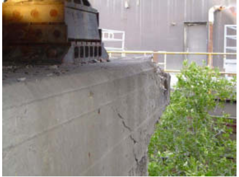
Pier 2: Pier Cap
