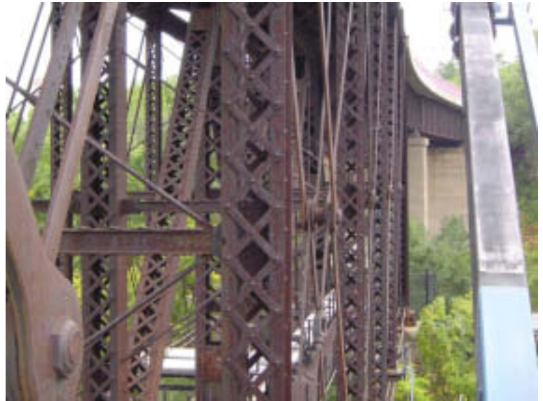
Span 4: Vertical Members
