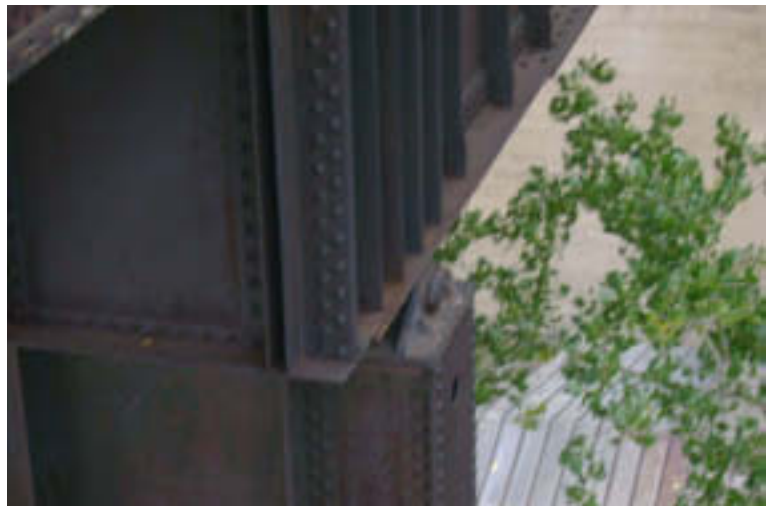
Pier 3: Upper Bearing
