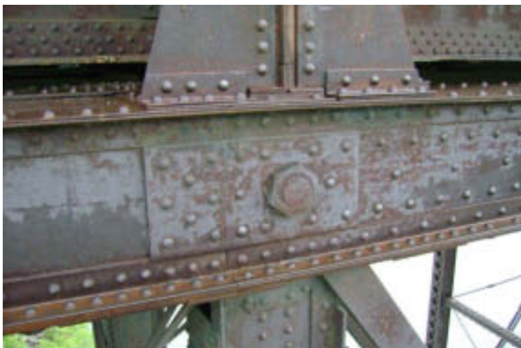
Span 4: Upper Chord Connection
