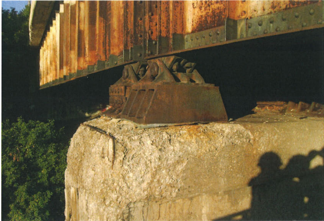
Looking Towards West Approach Span Bearings at Pier 7 of Bridge No. 9
