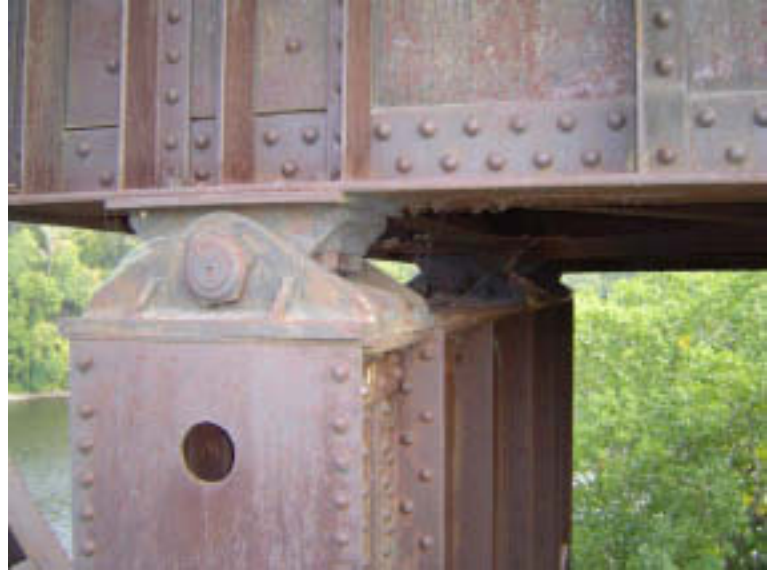
Pier 5: Steel Cap and Bearing
