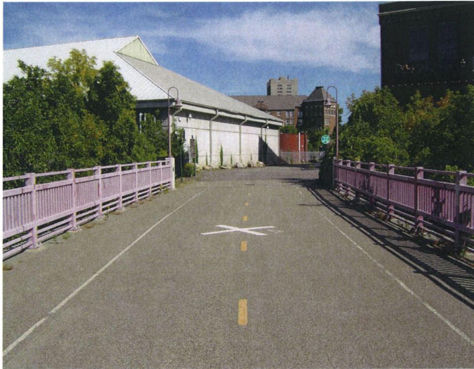
Looking East Towards East Abutment of Bridge No. 9
