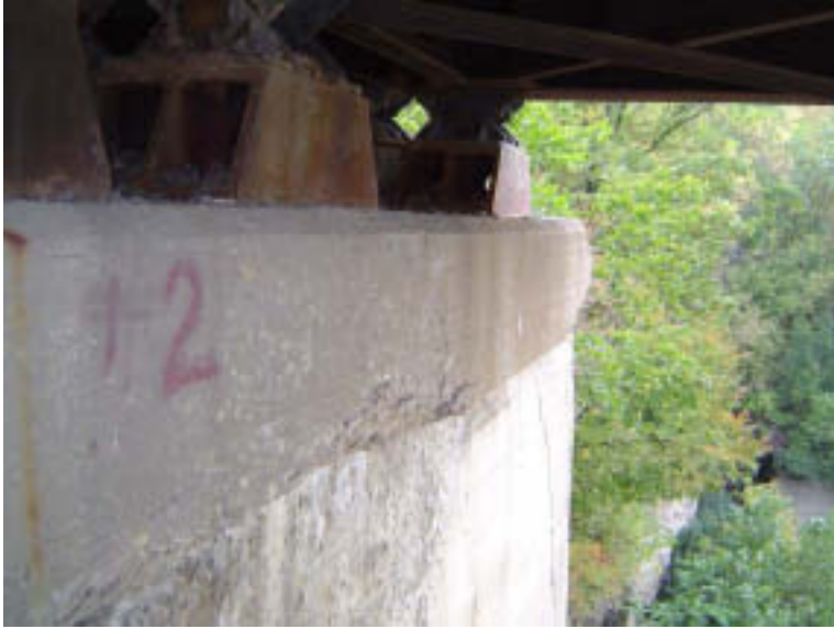
Pier 2: Pier Cap
