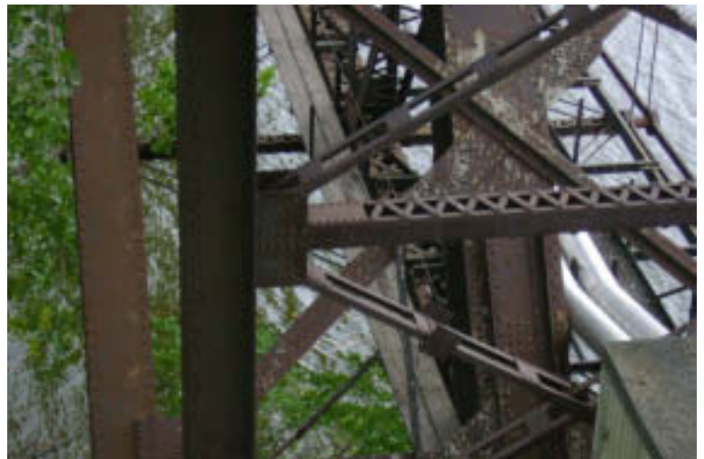
Pier 3: Steel Column Bracing
