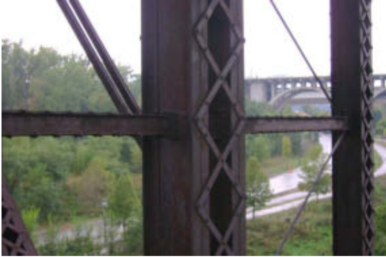
Span 4: Vertical Members
