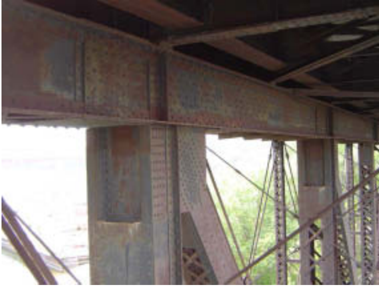
Span 4: Center Truss
