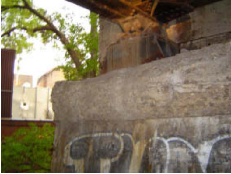
Abutment 1: North Side Bearing
