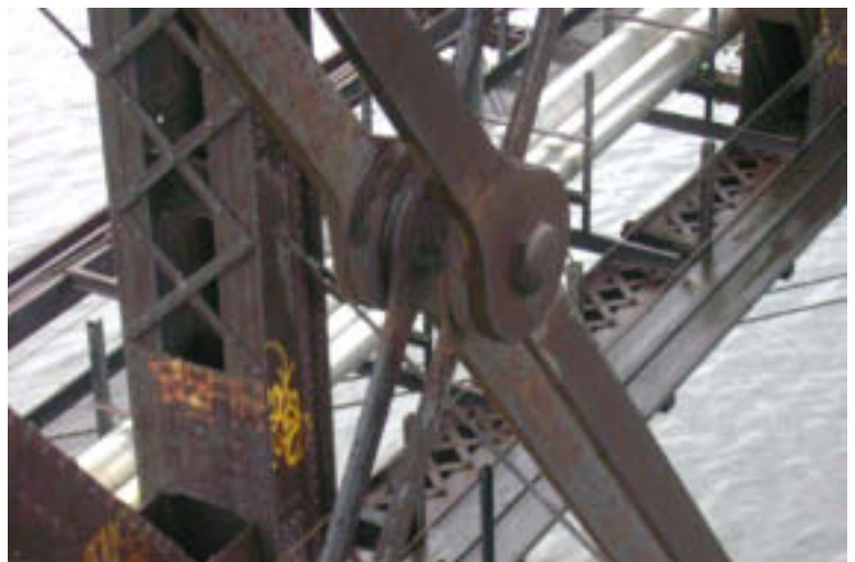
Span 4: Outside Truss Bracing
