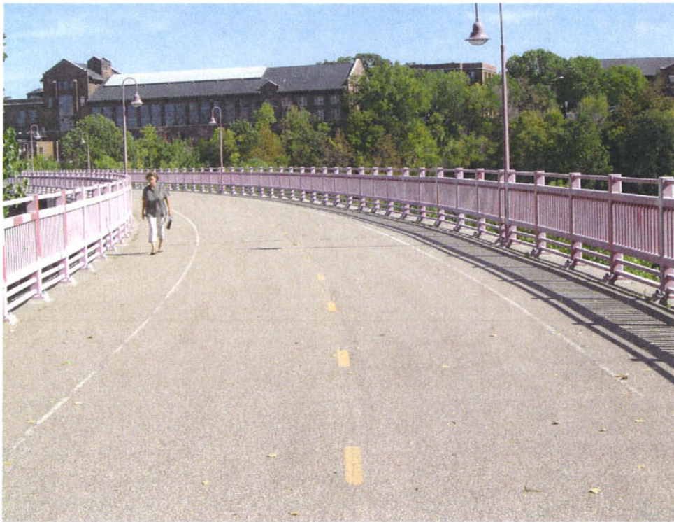
Looking East on Bridge No. 9
