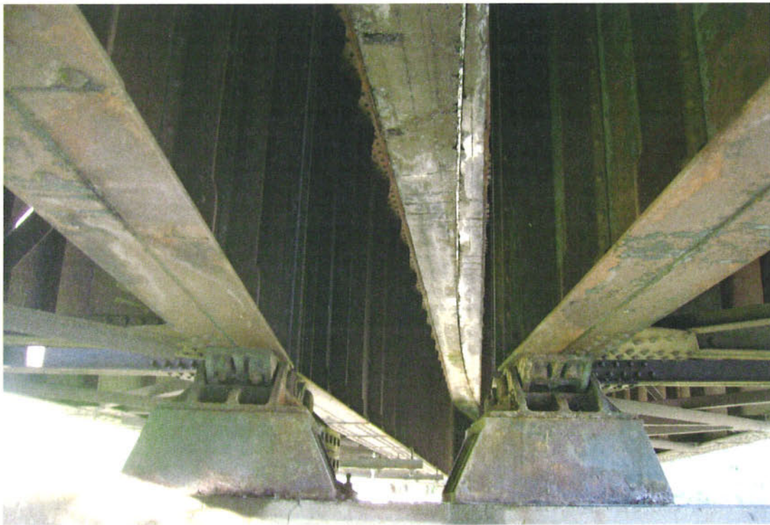
Center Deck Joint at West Approach Span of Bridge No. 9
