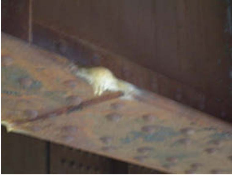
Span 5: Calcium Carbonate Built
