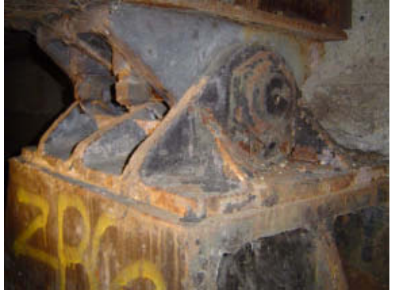
Abutment 1: Bearing
