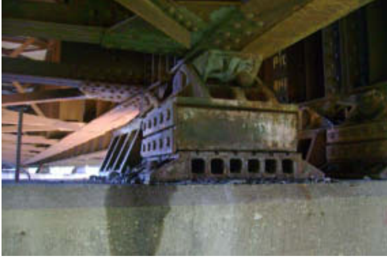
Pier 7: Drainage on Cap from Deck
