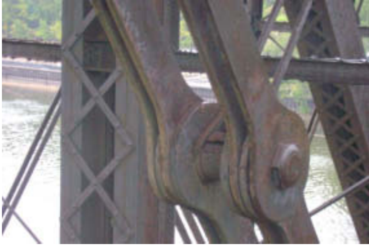
Span 4: Outside Truss Bracing
