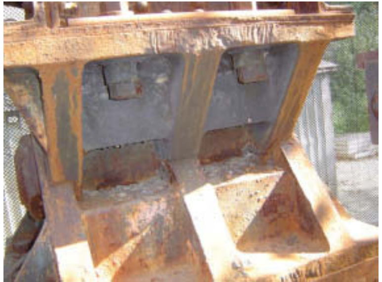
Pier 3: Lower Concrete Bearing
