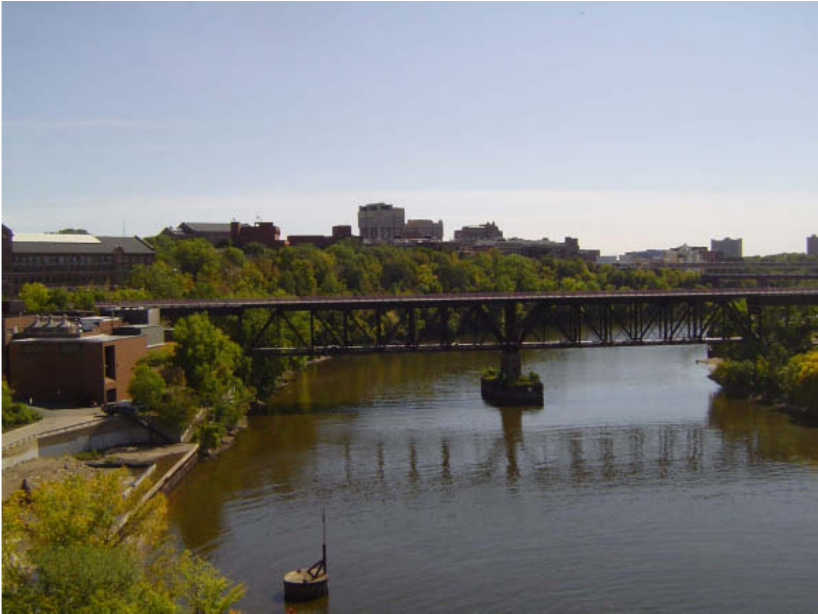
Elevation Photo: Looking South Towards Bridge No. 9
