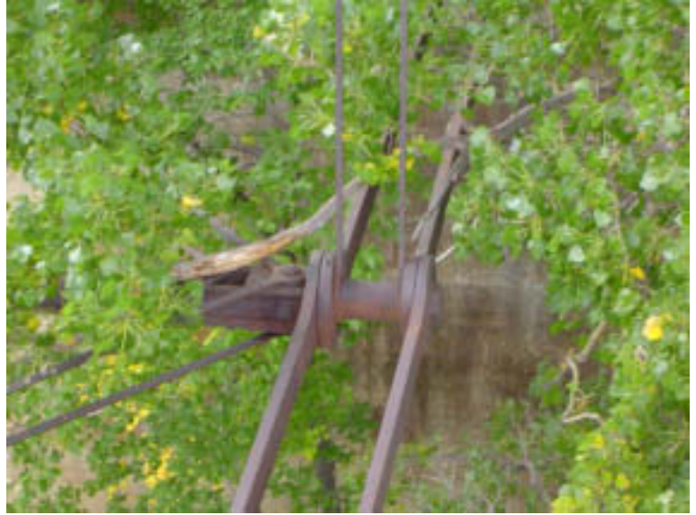
Span 3: Lower Chords
