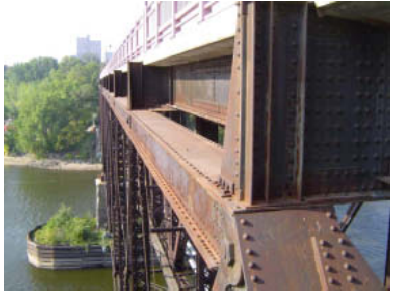
Span 3: Upper Truss Members
