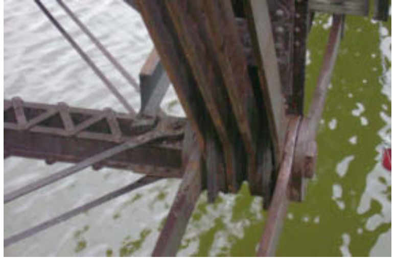
Span 4: Bottom Chord Connection
