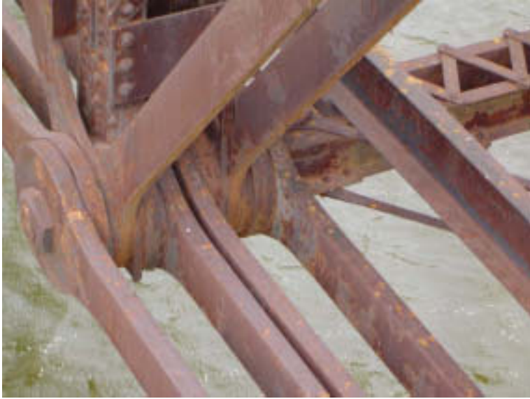
Span 4: Lower Chord Connection
