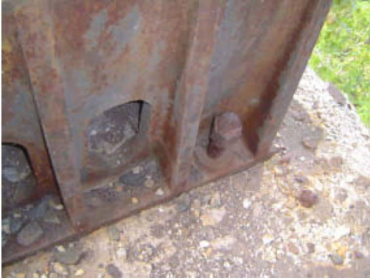
Pier 5: Concrete Cap
