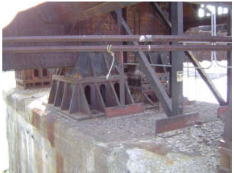
Pier 4: Center Bearing
