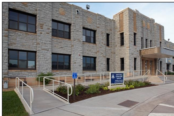
St. Paul Downtown Airport Administration/Terminal Building
