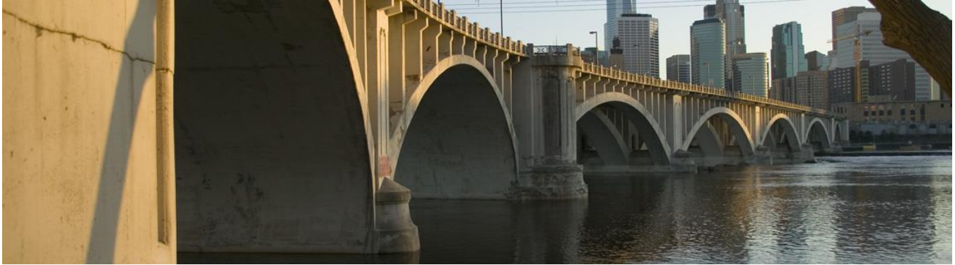
Figure 1. 3rd Avenue Bridge (MN 65)
