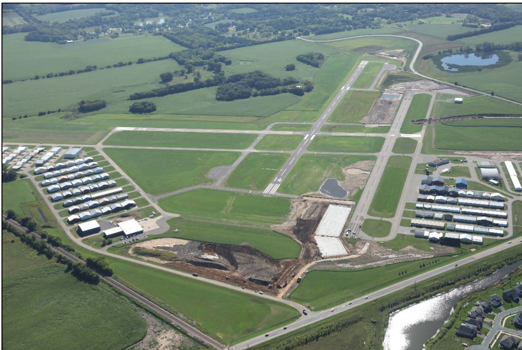
Runway 14-32 Relocation/Extension and Associated Improvements construction site.
