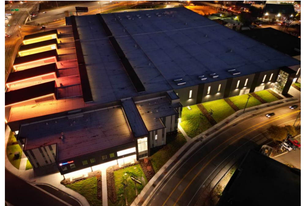
View of North Loop Garage exterior
