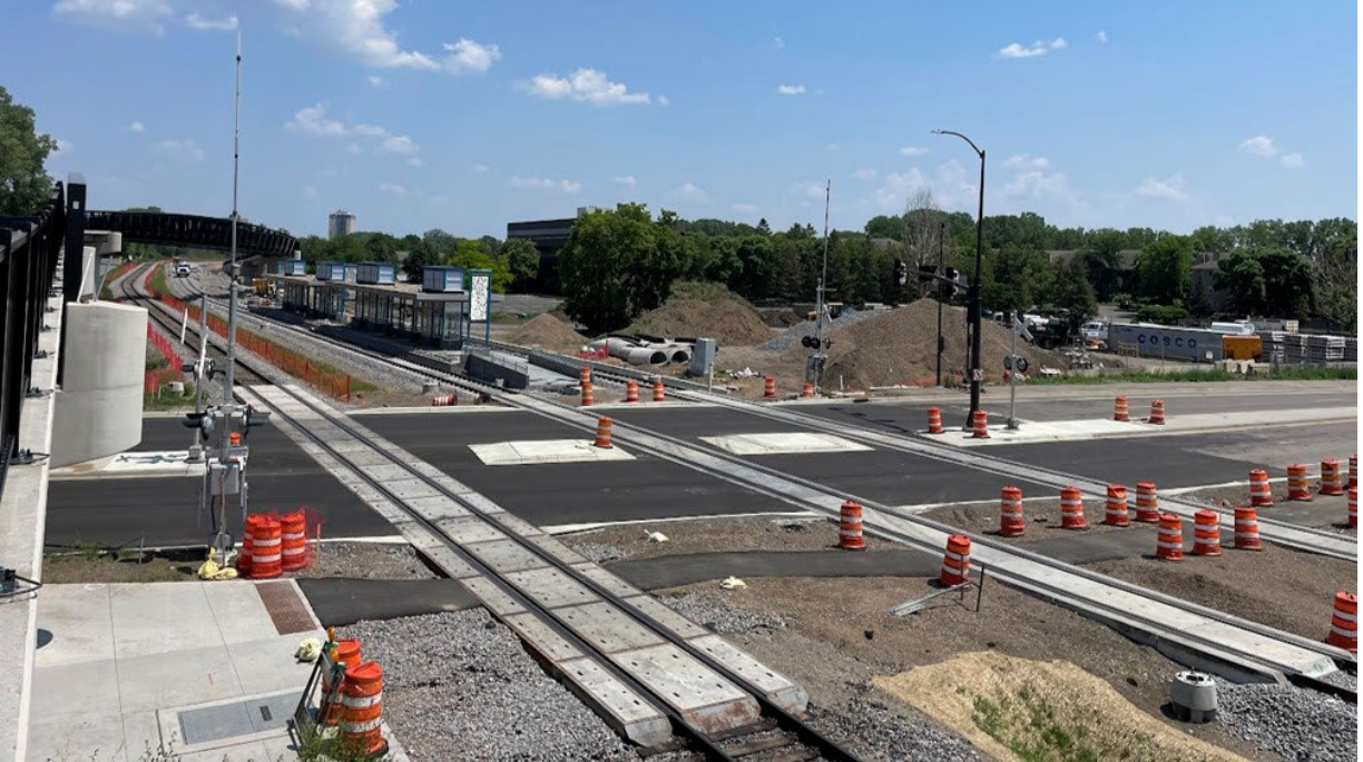
Beltline Boulevard Station
