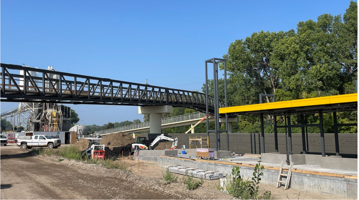
Luce Line Trail Bridge at Bassett Creek Valley Station
