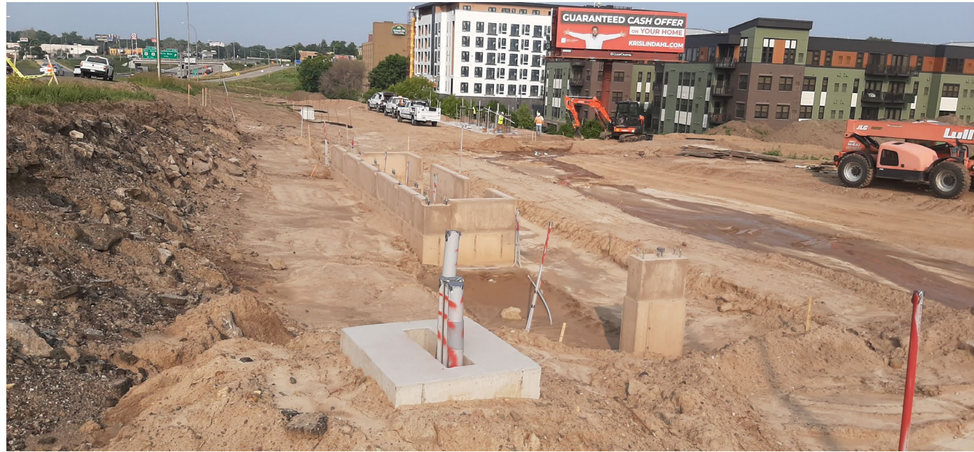
Hazel Station and Guideway grading
