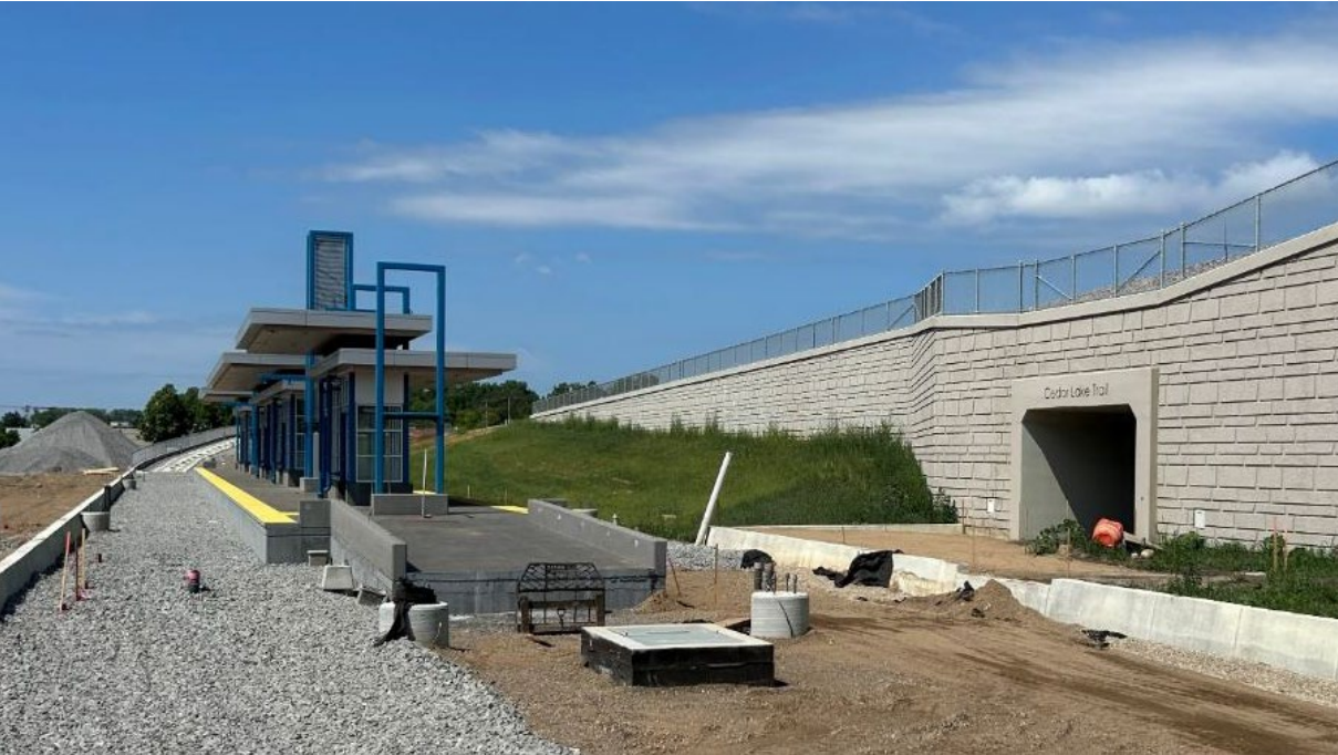
Louisiana Avenue Station
