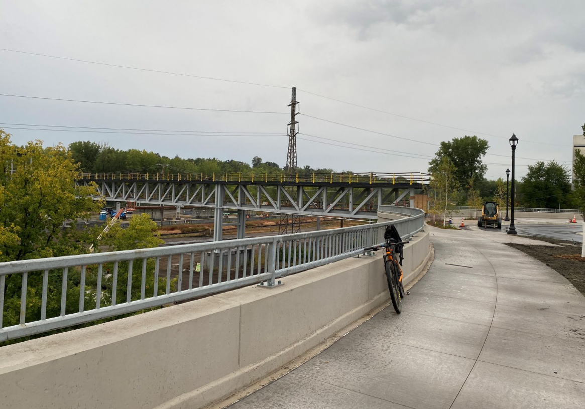
Bryn Mawr Station Pedestrian Bridge
