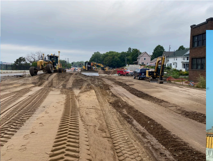
Guideway grading near Mounds Blvd
