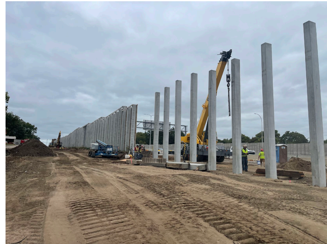
Hudson Road grading and Noise Walls
