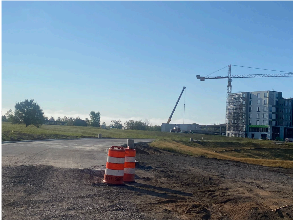
Helmo Avenue near 4th Street
