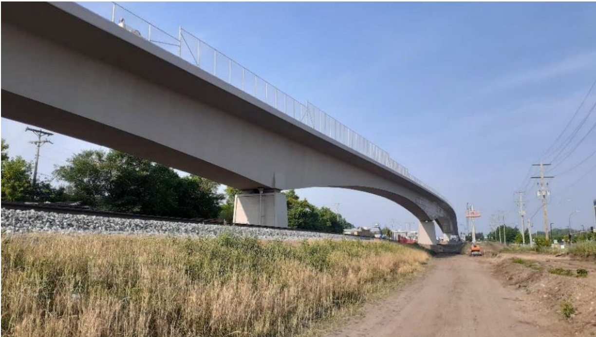
Excelsior Boulevard LRT Bridge
