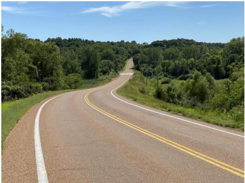
Existing conditions photographed above. This segment of CSAH 40 is a High Priority Segment in the Carver County Road Safety Plan based on crash frequency, narrow substandard shoulders and extensive curvature.
