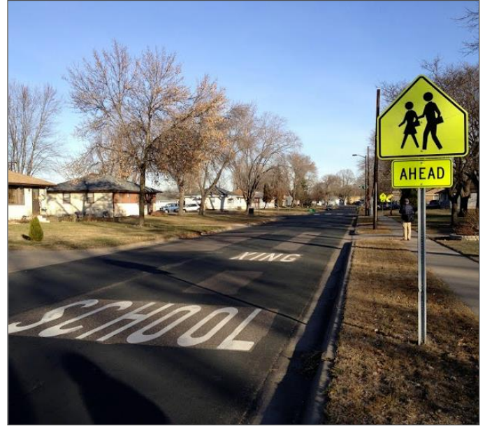
An existing advance school crossing assembly on Unity Ave near Fair Oaks Elementary.
