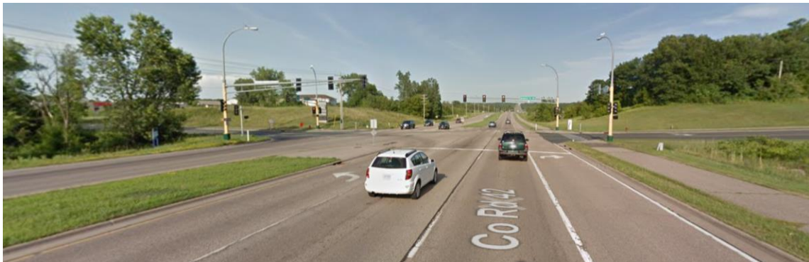
Figure 2: CSAH 42 at McKenna Rd
