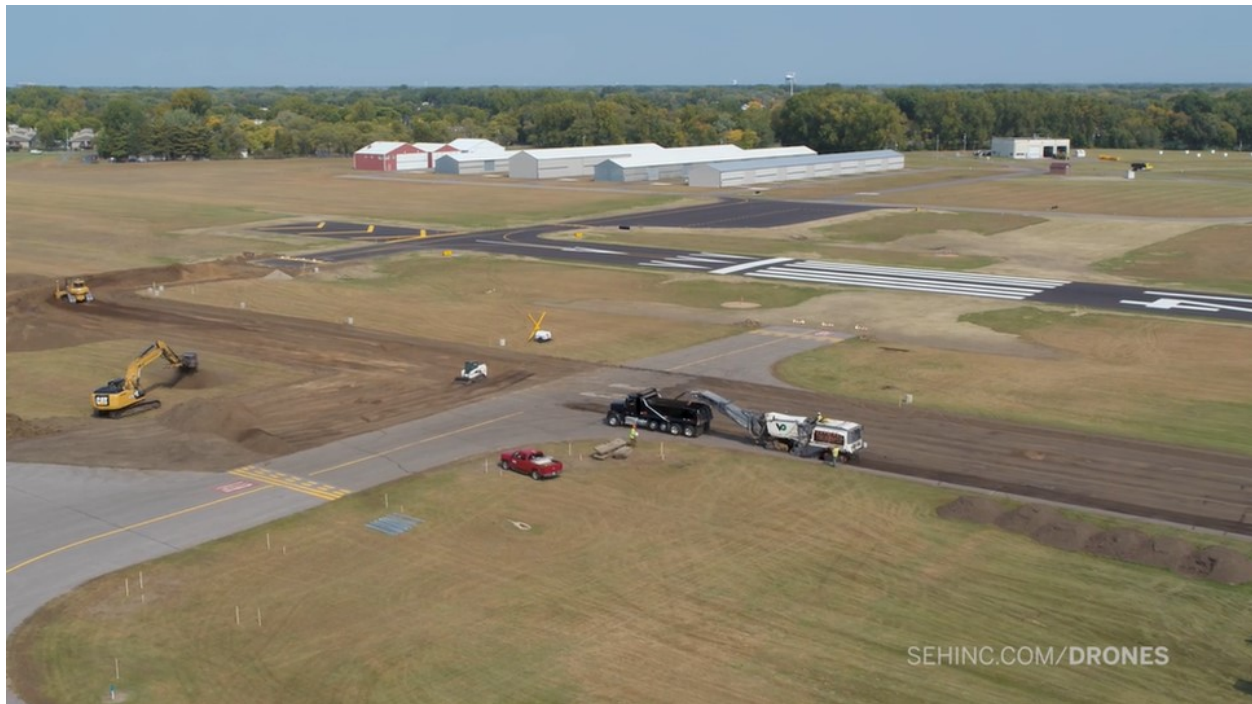
Photo of the Crystal Airport Runway 14R-32L and Taxiway E Modifications project construction.
