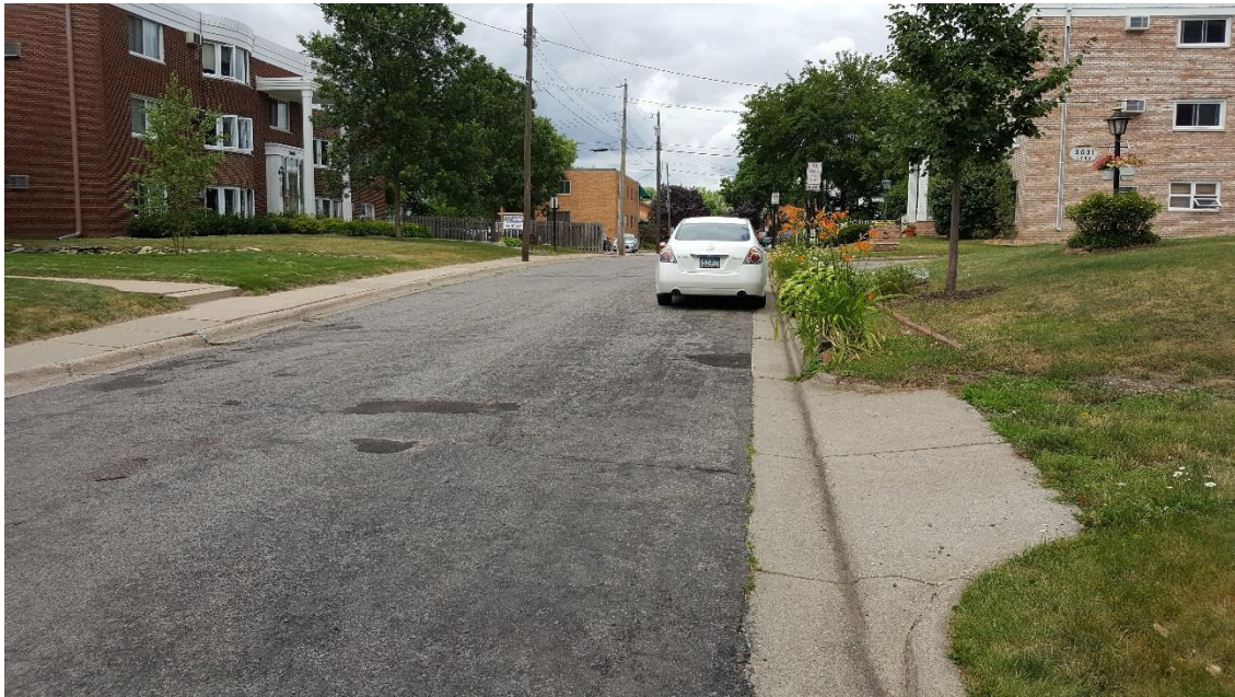
Lynn Avenue near Highway 7 – Looking north
