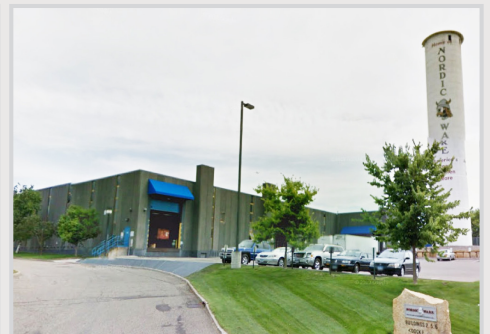
Existing industrial building (Nordic Ware)
