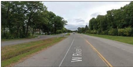
**West River Road (CSAH 12):** Currently West River Road is a two lane, rural county road section with varying widths of road shoulder. Vehicle travel speeds average 45 MPH.
