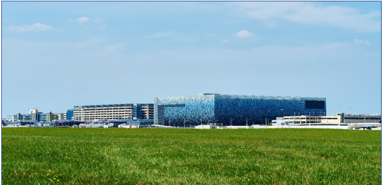
MSP New Silver Ramp with Access to Public Parking, Rental Cars and the Multi-Modal Transit Hub (shuttle, bus, LRT, bike, and walkway to hotel)
