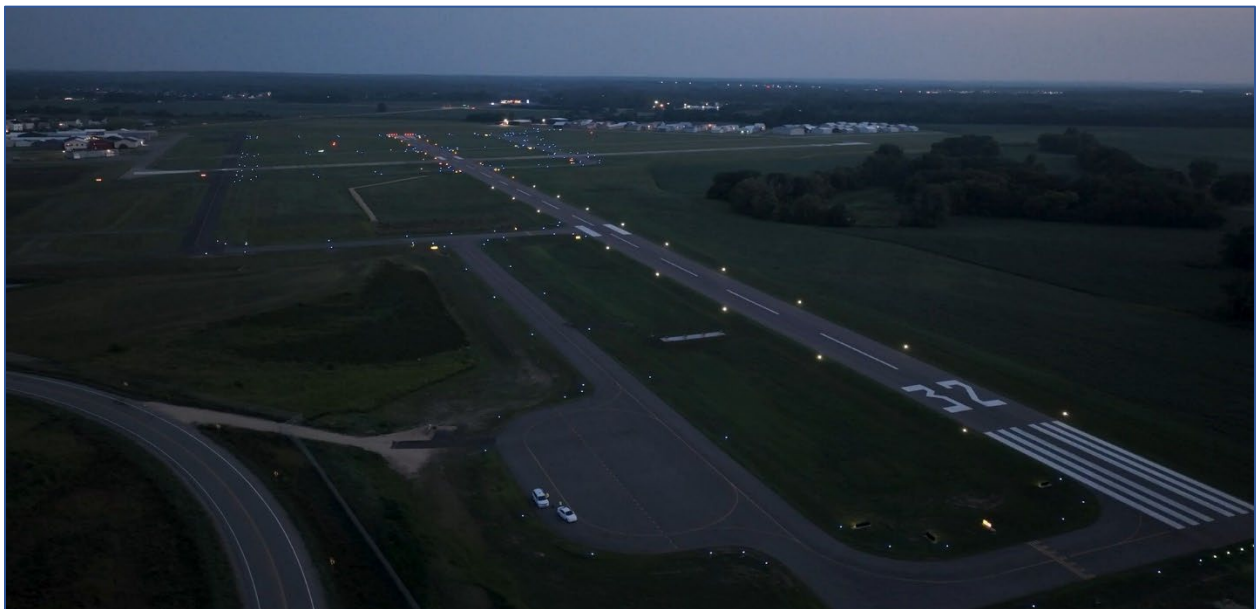
An early evening view of the realigned Runway 14-32
