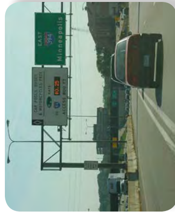
Figure 2-9: HOT lanes represent a method to add market forces to manage congestion.
