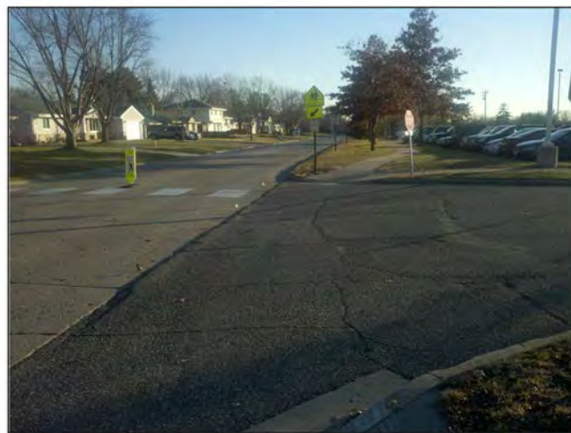
Wide crossing of the school driveway creates potential vehicle/pedestrian conflicts
