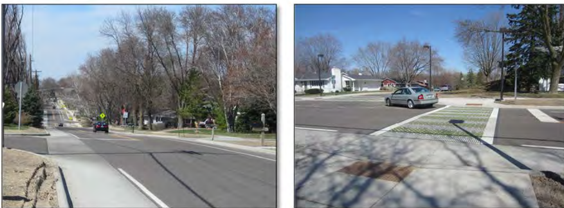
Reconstructed Tracy Avenue with bicycle lanes and high visibility crosswalks
