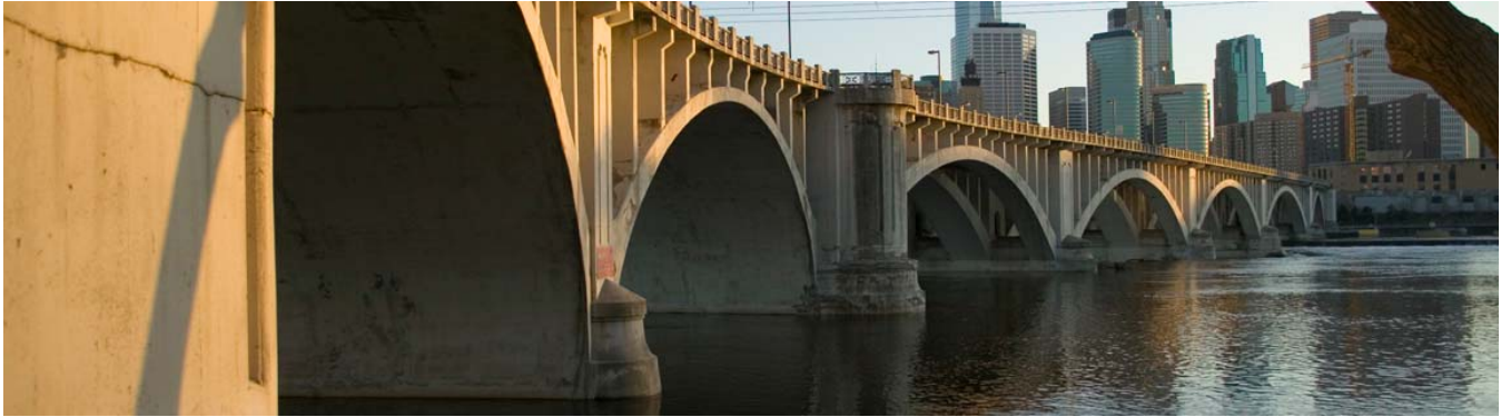
Figure 1. 3rd Avenue Bridge (MN 65)
