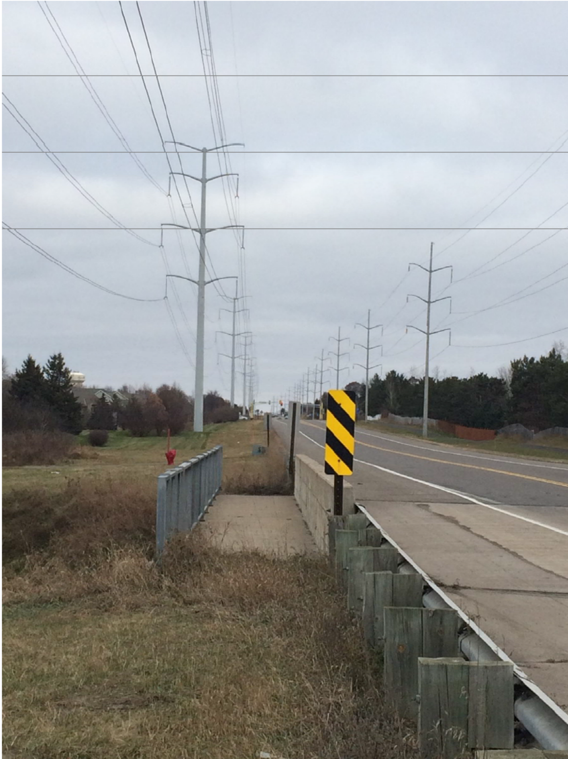
Figure 2: Existing Xcel Energy Transmission Power Lines (west side of CSAH 78)
