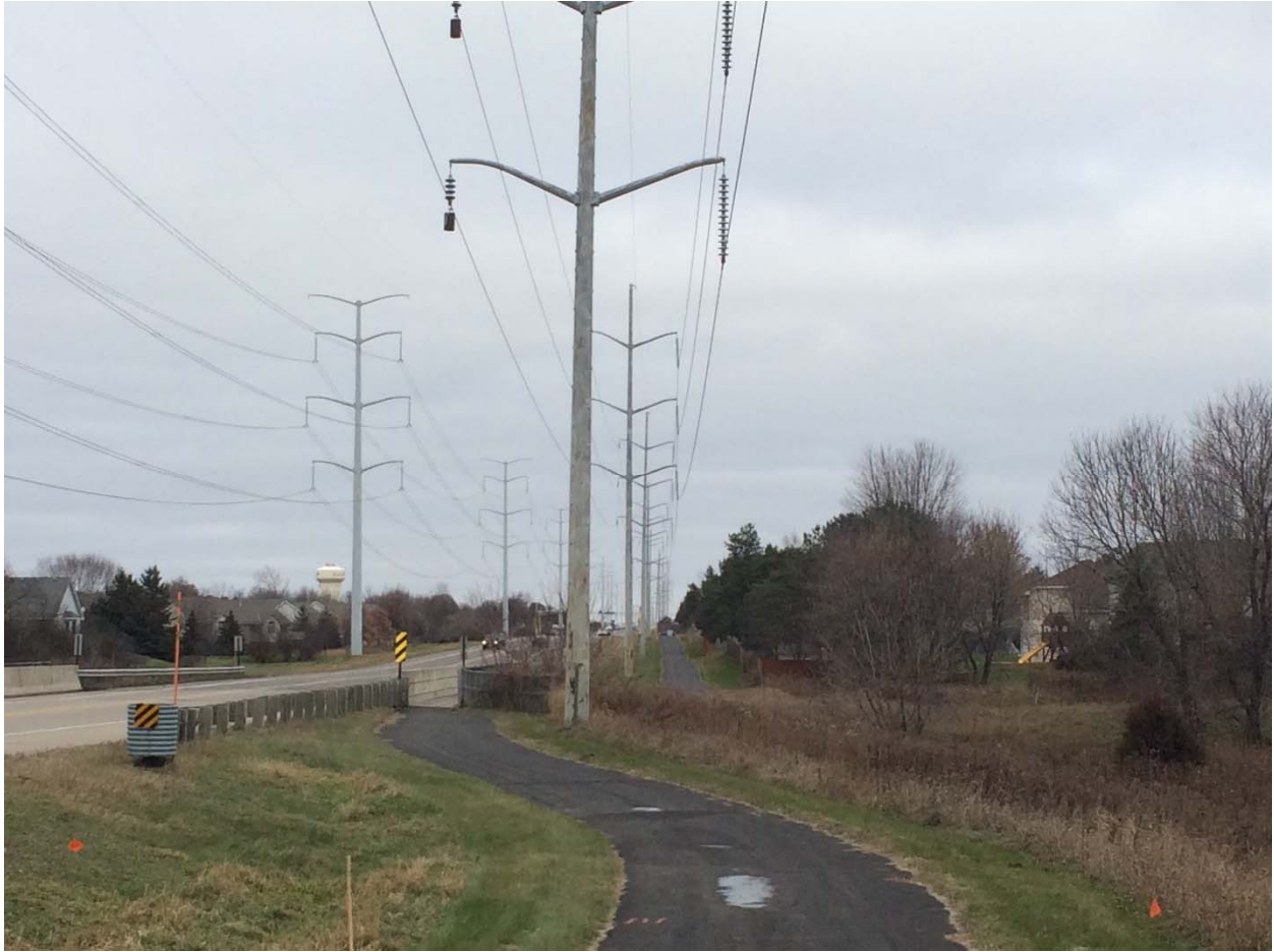
Figure 3: Existing Great River Energy Power Transmission Lines (east side of CSAH 78)
