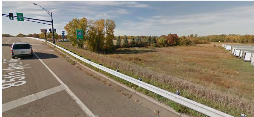
CSAH 32 LOOKING NORTHWEST (FUTURE ON-RAMP LOCATION)
