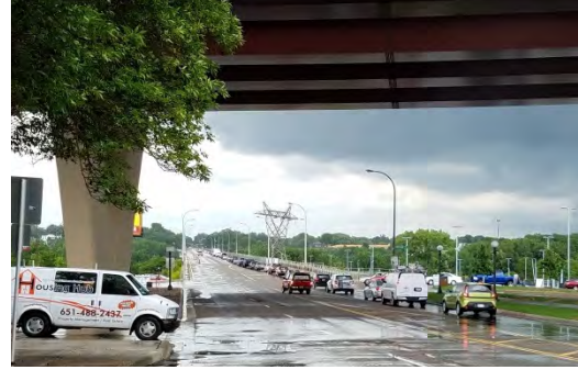
Photo 2. Outbound traffic backup across bridge (photo taken west of bridge, with US Hwy 52. above)
