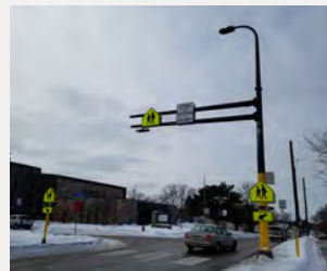
Traffic control device and APS push buttons
