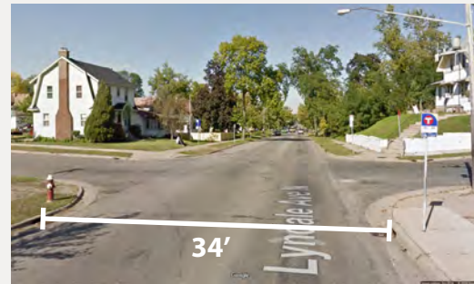
Typical existing cross section with an under-utilized parking lane, southbound travel lane, and northbound curbside travel lane.
