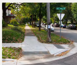
ADA-Compliant Curb Ramps
